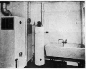
VIEW OF UTILITY ROOM of basementless houses. The heating unit is a gas fired counter flow forced hot air system
