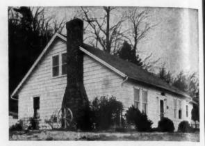
"CONCRETE CLAPBOARD" home of Victor Burkard, Barton, N.Y., whose blocks have ½-inch bevel on front to give clapboard effect
