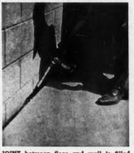
JOINT between floor and wall is filled with hot bituminous material. Right: Concrete masonry is laid with horizontal and vertical shell mortar bedding
