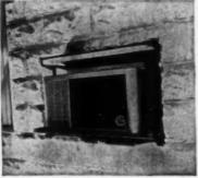
WINDOW FACSIMILE built in concrete block wall houses air conditioning unit
