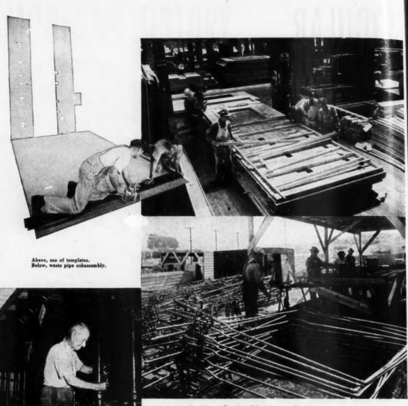
Above, assembly of large wall section. Below, shop assembly of piping.
