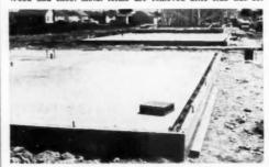
THE FINISHED slab shows the warm air discharge trench and duct openings at one end. As a final operation the trench is cleaned up to aid easy flow and proper distribution of warm air all along the wall
