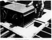
HEATING UNIT is installed and concealed in housing on the roof. Insulated joists form forced warm air supply ducts
