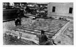
LATERAL DUCTS are laid from main duct to discharge trench along outside wall. Weight of tile-setter standing on block when placed in position serves to bed tile in vermiculite. Broken tiles between laterals prevent fill from spilling into main trunk
