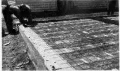
WITH FORMS in place. reinforcing mesh is placed over entire slab. Approximately 300 to 350 tile are required for the average two or three bedroom house. The system can be installed in about 60 man hours including lurnace and slotted baseboards
