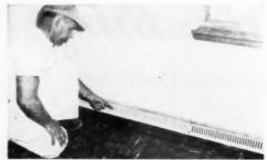
CONTINUOUS STRIP OUTLET GRILLES are placed over the shallow slots at an angle between the floor and wall. The strip, of slotted baseboard is divided into sections, each of which has its own individual control shutter
