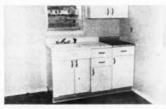
IN PORTION OF KITCHEN where cabinets are placed, ducts do not extend to wall; instead they discharge through grille in front of sink and cupboards
