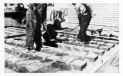
JOINTS ARE SEALED against wet concrete with strips of vapor barrier material. Strips are obtained by cutting roll of material in desired width. A spadeful of gravel on each end holds material while space between courses is filed with aravel
