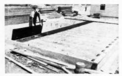
TWO-PIECE FORM of wood and steel plate is bolted to the foundation wall anchor studs. The steel strip angles downward and when mat is poured the slab edge becomes an angular bottle to throw the warm air upward as it comes out of the duct
