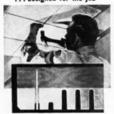
When installing acoustical tile chaose a job designed nail that combines ease of application with these special features: a head end which allows the nail to be driven home without damaging the tiles ...a collar which holds the tiles firmly in place...annular threading which gives superior holding power. The nails are furnished with a plated finish to prevent rust streaks where moisture is present. Send for free samples and descriptive literature.
