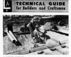
A VAPOR BARRIER is placed over the leveled off fill and is covered with a layer of losse vermiculite. Lateral ducts are laid on this material at right angles to the main trunk duct. Laterals are standard 4x12x12 inch wall tile
