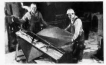
FABRICATING KAISER ALUMINUM into ductwork is so simple the contractors set up shop right on the job — and eliminated several steps in handling, trucking and storing assembled sections. Kaiser Aluminum is less wearing on shop equipment, can be fastened with rivets, by welding or with sheet metal screws.
