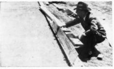
CLOSER VIEW of two-part form used to protect warm air discharge trench. In completed system a slotted baseboard runs full length of trench at an angle between the wall and floor. Wood and sheet metal forms are removed after slab has set
