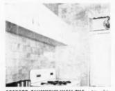
AB12120-ALUMINUM WALL TILE—Alloy Tile Corporation, Dept. A8, Belleville, N. J. This kitchen shows one of many applications of Altro-"Walluminum" individual aluminum wall tile. It provides light wall-load (14 oz. per square foot including mastic) and needs no special understructure, according to the company. Twenty colors, including mattes, are available. Company claims finish will not chip, crack or peel and is fadeproof. Can be installed on any evensurfaced, painted or upointed wall.
