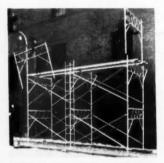
PREFABRICATED STEEL SCAFFOLDING is shown in assembly. Note pulley fitting for raising sections and material, and ladder for safety
