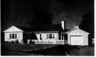
DETACHED GARAGE of this one-story ranch-type house is made a part of the overall arrangement by a connecting breezeway. The garage doors are placed off-center of front wall to provide for workbench on side wall. Roof ridge is centered on door. thus extending the roof line on one side and purposely establishing a lower eave line
