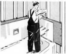
FOR TUB SURROUNDS. Prefabricated Carrara units are available for use in bathroom recesses. Panels are shipped to your job ready to install with all cut-outs made and holes drilled to your specifications. No cutting is necessary on the job. You have a variety of colors and a choice of 24- or 28-inch panels.
