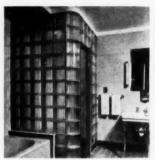
GLASS BLOCK custom-built shower stall keynotes bathroom with walls of structural glass "tile"
