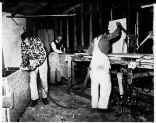
INDOOR CUTTING SHOP OF CONTRACTOR. Workman at left uses power plane: at right, door is mortised for lock; third workman rabbets for butts with router. Power tools speed work and cut costs
