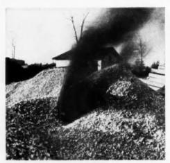
Heating of materials is necessary for cold-weather mixing and pouring of concrete. A fire in a large pipe keeps aggregates heated
