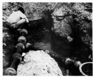
VITRIFIED CLAY TILE is extensively used for underground sewage lines. Connections are shown leading from both the house sewer and a catch basin to a septic tank
