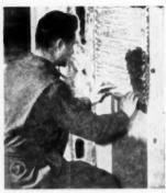
(3) Multiple layers of treated wood fibers stitched to heavy creped paper with a reflective aluminum foil cover on one side
