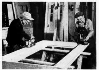
WORKMEN USING POWER SANDERS to finish doors. Power drill press with guxiliary oversize table is shown in the background
