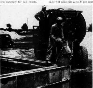
Prefabricated forms save the builder time and money. The units shown above are of rigidly braced metal panels
