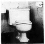
THE ONE-PIECE CLOSET and tank unit above requires no wall support. This siphon jet model is quiet in operation
