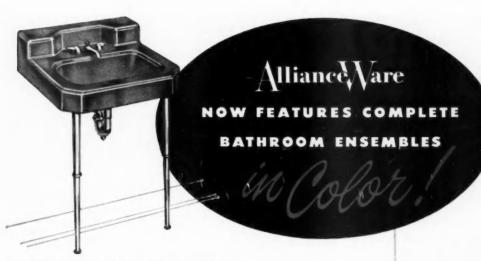
Shelf-back lavatory, porcelain-on-steel Model L-2018 has a bowl of generous capacity with a deep apron at front and sides that creates an unusual smartness in style. May be wall-hung or installed with legs as illustrated.
