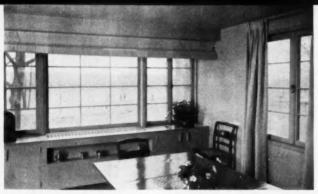
WOOD CASEMENTS are easy to install and to make weather-tight. Double-paned glass may be used, and screens and storm sash may be constructed as a part of the sash
