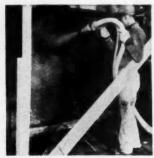
Pneumatically applied concrete is successfully used both on new construction and for repairing old concrete which has deteriorated
