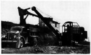
IN SAVING LABOR AND COSTS, modern equipment does much for the builder. Power shovel and truck dig and move earth quickly and efficiently
