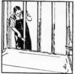
FIG. 22-After tub has been leveled, place roll of mastic around rim for waterproofing. Also, butter studs with mastic before setting glass panels
