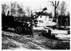
HOIST ON TRUCK can be used to lighten work and shorten time in a multitude of ways on building jobs
