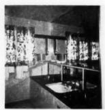
BATHROOM WALLS combine glass with structural glass; the polished plate glass mirrors are moisture resistant
