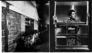
DOUBLE-HUNG aluminum windows are weather-stripped at the factory and do not require painting. Care should be taken to prevent scratching or staining during construction
