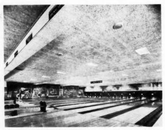
Rough surfaced acoustical tile material has decorative as well as acoustical function. Material may be treated with paint without impairing its sound-absorbing qualities
