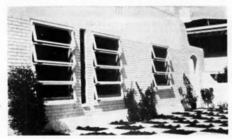
AWNING WINDOWS supplement architectural treatment where horizontal lines are wanted. Good ventilation is possible; wood and metal units are supplied in a variety of sizes
