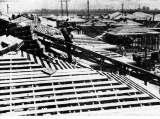
You may be paying more than you think, for "inexpensive" roofing. Don't fail to figure the cost of sheathing when estimating roofing expense. Certigrade cedar shingles, because of their great strength and rigidity, require only half the sheathing that you must use on ordinary roofing.
