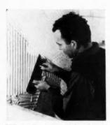
FIG. 13—Mastic is applied to the wall first in a vertical and then in diagonal pattern
