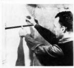
FIG. 17—When all of the tile is interlocked in position, feature strip is then applied
