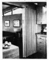
PLASTIC AND FABRIC coverings for folding doors mounted on steel frames make possible great space saving and can be used as design features
