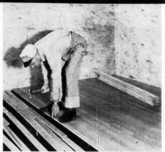
WHEN FINISH FLOORING 1/2 by 2-inch or 1/2 by 1 1/2-inch is used, 6d bright wire casing nails are best—one nail every 10 inches. Flooring 3s-inch thick takes 4d nails spaced 8 inches apart.
