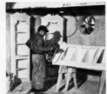
A POWER SPRAY UNIT, fed from a pressure tank, is used in the shop for spraying doors, cabinets, and bookshelves. Note exhaust fan for worker protection against fumes
