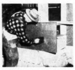
INSULATING BOARD SHEATHING IS applied by nailing to intermediate studs first with the nails about six inches apart. Nails around the edges are then spaced three inches apart.
