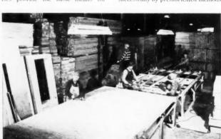
PRODUCTION LINE for roof panels. Plywood sheathing covers the rafters and serves as the base for roofing paper and asphalt shingles which will be applied at the site
