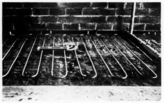
A TYPICAL sinuous radiant heating coil of 34-inch copper tube on 9-inch centers
