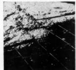
Steel reinforcing rods are used to increase the tensile strength of concrete. Note how the concrete is placed under the rods so that the reinforcing is imbedded in the concrete. Rods should be at least 3/4-linch from the surface
