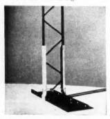
SNAP-ON Trussteel stud shoe designed to speed erection of metal studs for metal lath construction. The snap-on holds shoe in place while wire tie is applied near floor
