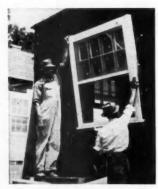
STEPS in the installation of a factorybuilt unit. This window, complete with screen and storm sash, may be quickly installed in one operation on the job
