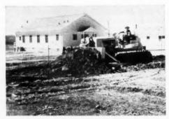
CRAWLER TRACTOR WITH BULLDOZER BLADE and cleated treads is efficient for heavy scraping and grading, can also dig shallow excavations
