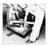
A Hunter Package Fan is the most practical and least expensive method of keeping a home comfortable on hot nights. This compact unit is easily installed in any new or old home. Furnished complete with ceiling shutter and trim-no extras to buy or build. Choice of four sizes, to fit any home and climate.
