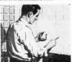
FIG. 21—Excess adhesive is removed and the joints are pointed with a finger. The tiles are then cleaned with a sponge dampened with water or mineral spirits
