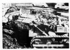
THE CRAWLER TRACTOR AND FRONT-LOADING ATTACH-MENT are a versatile combination for digging, earth-moving, and many jobs of handling materials on the job
