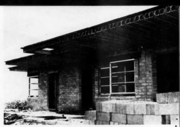
Slabs of prestressed concrete make the 8-foot overhang of the eaves possible here
