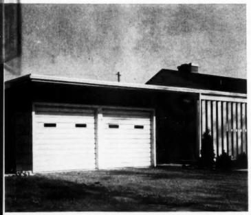
WIDE OVERHANG gives protection from the weather while small windows set into upward-acting doors add note of interest
