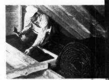
WOOD FIBER BLANKET with nailing flanges which fasten to framing members
