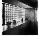
HALLWAY is transformed to attractive, light area with glass block wall treatment. Casement window at left
