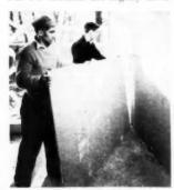
Second stage in double-wall construction with wallboard in horizontal application as finish layer
