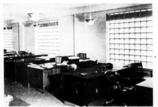
PANELS OF GLASS BLOCK admit flood of daylight that is softened and diffused throughout entire office
