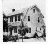
fumes are a problem. Both houses were painted at the same time, No. I with a first-quality white lead and oil base paint, No. 2 with a lead-free paint. The houses are shown after 14 months of exposure.
