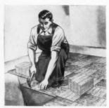
PARQUET FLOORING may be nailed to a wood subfloor or an old finish floor in the same manner as strip flooring. Proper construction of the subfloor is essential. Floor joists must be on 16-inch centers and covered solid with 25/22 by 4-inch or 6-inch subflooring thoroughly dried and nailed securely. The surface must be even-boaring
