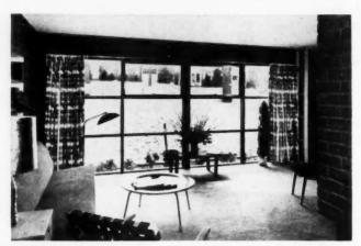
WINDOW WALLS using a combination of hinged sash and glass set in stops may be purchased as a stock unit in various sizes. Double pane construction reduces heat loss
