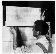
PHOTO ABOVE Illustrates the approved method of applying asbestos-cement siding shingles. First, the sheathing or old siding is covered with a felt underlayment. Shingles are then aligned and natled in position, using non-corrosive natis, with a felt backer strip at each joint. Strips lap lower courses. At least one nall penetrates each strip
