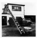
CONVEYORS provide an efficient method of lifting brick, tile, roofing materials to second or third-story level. Extensions are available to adjust the height of the conveyor to the level needed
