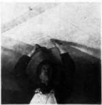
Tile is applied to ceiling, starting at center with temporary straight-edge nailed up for a guide
