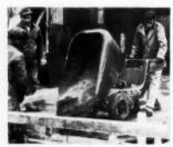
POWER-OPERATED CONCRETE BUGGY has large capacity, speeds production, cuts majerial-handling costs
