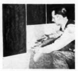
INSULATING BOARD LATH is applied with the long edges at right angles to framing or furring. When small greas are to be filled out insulating lath must be used; not wood.
