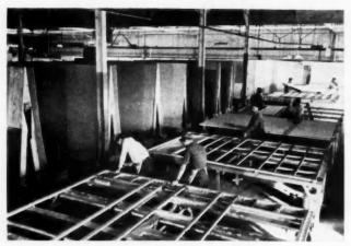
JIG AND FLOW LINE for interior wall partitions. "Starting" jig is in foreground, and subsequent stations complete the panel assembly
