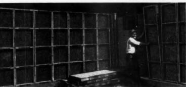
To strip wall remove locking wedges and connecting bolts. Pull panels back easily. Break off tie loops with a 1/2 twist. Wall is smooth, strong and waterproof.
