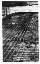
TYPICAL adjustable steel post is shown at left. It can be used to level up floors. Right, steel wire reinforcing mesh
