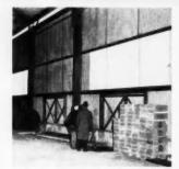
WHITE CORRUGATED plastic panels mesh with galvanized iron sheet siding, provide light with privacy
