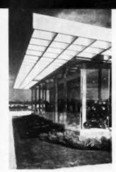
ATTRACTIVE plate glass displays can be site-built with glass precut by maker
