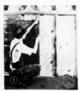
(5) Wool bats with vapor barrier and nailing flange
