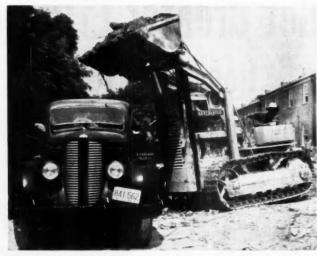
CORRECTLY SIZED EQUIPMENT for the job to which it is assigned is always important. It is costly to use a small unit for a heavy job or a heavy unit on a small job
