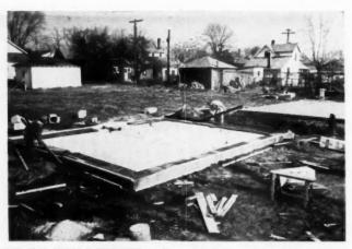
THE SLAB FLOOR FOUNDATION is the prevailing type for prelabricated houses in the lower price brackets, but full basements are often used. The builder prepares the foundation in advance of delivery of the packaged house from the factory
