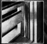
Dura-seal is cut exactly to the pitch of the sill—another feature that helps make a more attractive and efficient window.
