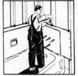
FIG. 24-Do the same with the end panels. Let plasterboard extend beyond tub to next stud. If wainscot is 48 inches high, follow the same sequence in setting around second course
