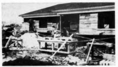
STONE VENEER being cut and laid with aid of radial saw equipped with special cutting wheel
