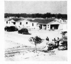
TRANSIT MIX CONCRETE is loaded into wheelbarrows for construction of the ribbon driveway. The overall view of the project shows root lines and many house variations
