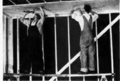
nailing near the center of board working outward toward the edges. Press the board hard against the traming while nails are being driven. The last hammer blow should set the nail flush with the surface without breaking the paper.
