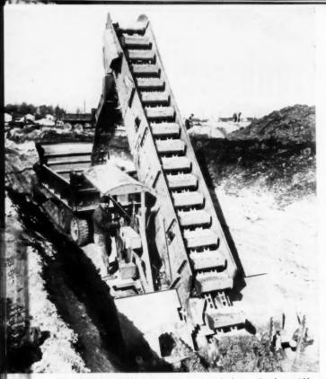
BIG. POWERFUL TOOLS such as this expensive loader are found to quickly pay for themselves—li kept busy and cared for properly. Spinning teeth at the bottom break up large chunks of packed or frozen earth into a "fluffy" mass before placing it in the buckets
