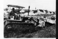
CATERPILLAR D-6 diesel-powered bulldozer, at work on backfill. This machine is also used for preliminary leveling of the home sites, digging and grading
