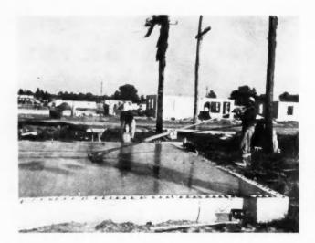
FOUNDATION AND SLAB: The first two courses of concrete block are plumbed and leveled so that they can be used as a screed in the slab finishing operation. A pipe brought up to level is the center screed. The long handled wooden float keeps finishers off the slab
