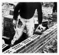
UNDER NORMAL conditions, a mason can easily lay 450 SCR brick per day, or 100 square feet at wall. The hole size and arrangement were selected to duplicate the grip and finger spread used by masons in laying 4-inch brick. SCR brick is laid with 1/2-inch mortar joints, turns corners nicely and builds jambs or openings without special additional units
