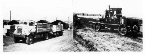
LARGEST LUMBER TRUCK is an Autocar 4-ton flatbed with a war surplus trailer. Plywood is being delivered to the precutting site
