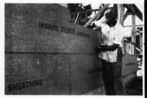
BILDRITE GOES UP FAST. One carpenter can sheath 1,000 square feet in six to eight hours and cut labor costs at least 25 percent! What's more, carpenters like to work with Bildrite because if's so clean and easy to handle, easy to cut and easy to apply.
