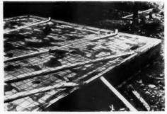
DUCTWORK PLACED prior to pouring concrete slab
