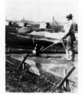
FLOATING and finishing floor slab. Whiteman Model J machine weighs 105 pounds, has small trowel diameter for operation on small crowded areas and around obstructions. For small contractor
