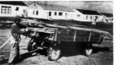
PRECUT LUMBER is sized and then loaded at the centrally located yard. Saw is a Comet Clipper radial arm. Lumber is loaded on the trailer in the foreground for delivery to the site. A model A ford moves the trailer mounted saw
