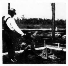
WOREMAN TAMPING the under-slab fill. The Jackson Compactor tamps 12-inch thicknesses to highway specifications. One man operates the machine
