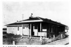
A 6-FOOT PORCH and a 2-foot roof overhaug give the new addition the length needed to tie in harmoniously with the house. Windows were framed into each of the three walls to give as much natural light as possible. A louver was installed to help insure proper ventilation above the ceiling.
