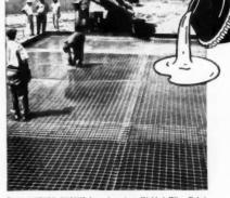
THIS PICTURE SHOWS how American Welded Wire Fabric knits the floor of an entire home into one solid concrete salb. It distributes the strength of steel eventy throughout the salb, controls cracking, prevents heaving and spalling. Floor salbs like this insure long-lasting living comfort and rock bottom economy for home owners.
