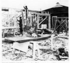
INSULATING BOARD is cut by Skilsaws powered by generators taken to the job
