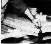
DRIVING <sup>3</sup>s-inch nickel plated thumb tacks (one at each end) in groove at bottom of wardrobe door to facilitate sliding. Doors slide on hardwood guides pressed in slots
