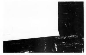
BASEBOARD: Miami baseboard styling was used throughout the house at a considerable saving. The installation acts as a plaster ground as well as the finished base. The top of the board is beveled on the back side to allow the plaster to run down behind it. Plasterer scores the joint between the base and finished wall material
