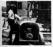
INTO THE MIXER goes one of 6,000 bags of Atlas Mortar used to put up 700,000 face bricks and additional concrete masonry work on the Kenwood job.
