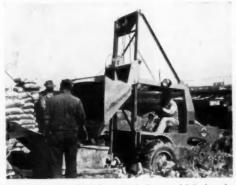
WAGNERMOBILE SCOOP, dubbed "scoopmobile" by the builders, pouring aggregate into one of the mixers. Three of these are on the job and each is estimated to save the labor of three mon and do the work twice as fast
