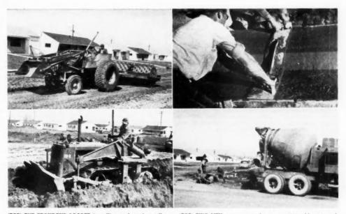
(TOP) THE FRONT-END LOADER is pulling a sheepsloot roller compacting street fill. Front-end loader is a L.I. Case tractor. (Bottom) crawlspace construction requirements are 30 inches. Builder uses International TD-3 to push out for crawl space and foundations. Later machine will be used to backfill
