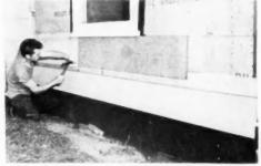
**COMPLETE INSULATION** is an essential feature of a job like this. Mineral wool batts were used. Insulating sheathing was used as well as an insulation board shinglebacker, instead of low grade shingles as under-coursing.
