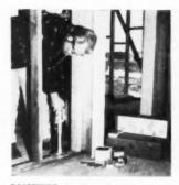
FASTENING partition plate to concrete floor with Drive-It. Avoids costly quessing about where bolt should go, placing in wet concrete, and finishing around by hand. Drive-It uses 3<sup>3</sup> inch case-hardened bolts, sinks two inches in concrete, costs 27 cents a shot, fires about 100 in an hour
