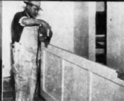
ELECTRIC screwdriver (Van Dorn) attaches butts. Foreman estimates 45-minute saving compared with ratchet type screwdriver
