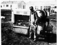
ENOUGH POWER TO OPERATE 8 power handsaws is delivered by a  $37\frac{1}{2}$  K.W. Buda generator. The rig is mounted on skids to be pulled along the ever moving building line
