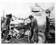
CONCRETE MIXER, which keeps a crew of three men busy pouring foundations. Two of these machines are used at each site. A third is set up in advance for the next foundation. A fourth mixer services a flatwork crew
