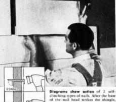
clinching types of nails. After the base of the nail head strikes the shingle, further tapping flattens the head and clinches the foot against the backside of the Weathertite Sneathing.
