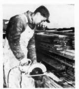
ELECTRIC SAW poised to do a quick job of cutting 2x8 joists. A generator supplies the power whenever an outside source of electricity is unavailable
