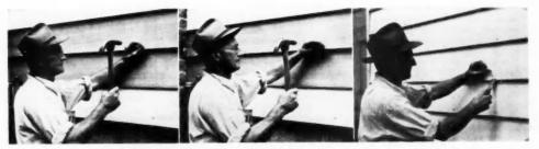
**SIDING SHOULD BE NAILED** both top and bottom to prevent curling. Exposed nails should be countersunk and puttied for best appearance and service, after the primer goes on. When the putty has dried, the siding is ready for the finish coating.
