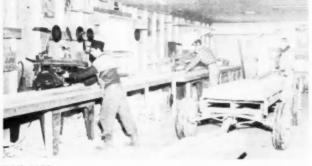
IN CUTTING ROOM, two DeWalt table saws. of 220 volts. carry the work load. Lumber for each house is cut. loaded neatly on a trailer and bound with steel tope by means of ratchet and steel binder. This package is then delivered to the individual site
