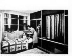
A PATTERNED GLASS PARTITION was framed into the wall which divides the new room from the old. An opening was left at the top to allow cross ventilation, Three-quarter-inch factory fuished insulating was used on the walls. Tempered hardboard in its natural brown color was used as facing on closets and drawers of storage wall.
