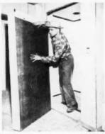
METAL SHOWER CABINET is soundproofed with backing of Masonite tempered hardboard. The usual metallic sounds caused by water spray are said to be deadened by the hardboard. Application is, with mastic; here, workman presses board in place to assure a good bond. Shower unit is a product of Fiat Metal Manufacturing Co., which recommends sound deadening in all recessed residential installations
