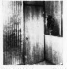
PLASTIC PARTITIONS AB55243 lexolite, is a shatter-proof plastic material manufactured in 12 colors and available in either plain or corrugated sheets. Thicknesses of 1/16,  $\frac{1}{6}$ , and  $\frac{1}{4}$  inch are manufactured and can be used for room partitions, window openings, sky lights, shower doors, awnings, and decorative effects. Plexolite Company, Dept. AB, 4223-25 W. Jefferson Blvd., Los Angeles, Calif
