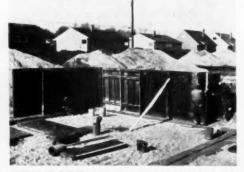
SETTING UP FORMS faced with 4x8 sheets of %i-inch plywood for the pouring of a 10-inch concrete foundation. During the winter, about four foundations can be poured daily: in warmer seasons, the rate can be doubled or trebled
