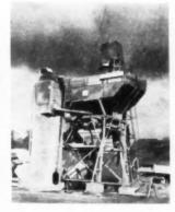
READY MIX plant specially set up on job site for this development to save costly trucking of concrete up mountain side
