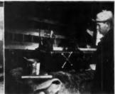
FASTER AND CHEAPER is the pipe cutting operation using a Toledo 999 pipe cutter. Journeymen plumbers install but do not cut pipe. Various stack fittings are predabricated in a plumbing shed
