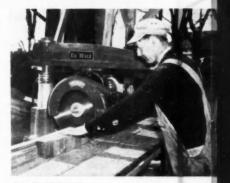
RADIAL ARM SAW, one of two operated by five-horsepower motors to pre-cut nearly all the framing lumber from plate to ratiers, as well as aable ends
