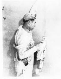
WALLBOARD TAPER reduces taping costs approximately 50 per cent in a 1000 sq. ft. house. Builder claims that a better job is done as the correct amount of joint cement is used. Later joint finishing is easier Wallboard Taper Saves Labor
