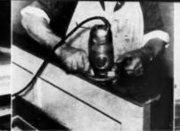
TEMPLATE is tacked to edge of door to rout out for butts
