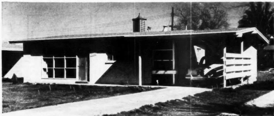
Cost Estimate on the Lux-Econ House Erected in Phoenix, Arizona, on Owner's Lot
