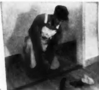
3. Next attach guide to the floor. No drilling is necessary.
