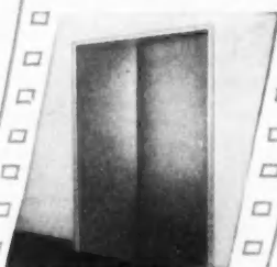
8. Finished closet door assembly, ready for painting to match any color scheme.
