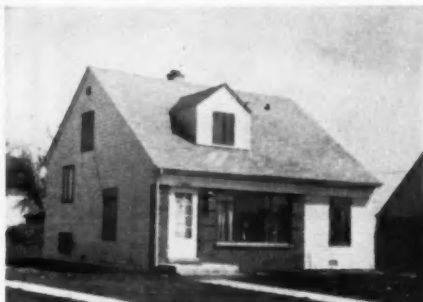
Tri-level model with conventional front elevation, has half basement. A large unfinished third bedroom is on top level. Elevation below left, layout right
