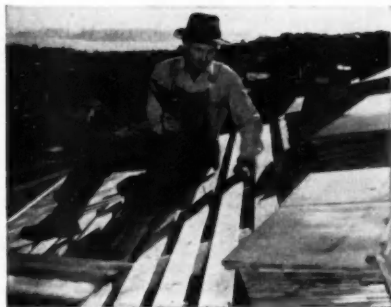
SPACED SHEATHING —Cedar shingles add strength to the roof! They can be applied on spaced roof boards. Save half the sheathing cost. Save nails. Save labor.
