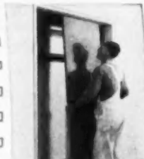
6. Set doors in place by inserting top in guide channel. Place rollers in floor guides.
