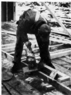
Power hand saw cuts cripples above doorway header. The sidewall construction begins after both gable ends have been tipped into place. House is framed and sheathed in one day
