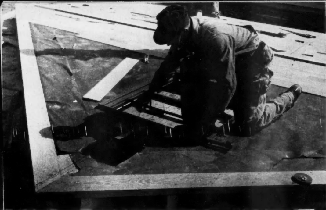
Metal window is set in the horizontal one-piece gable end
