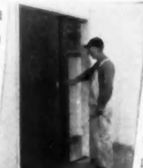
7. Make final adjustment on guides so they move smoothly and easily.
