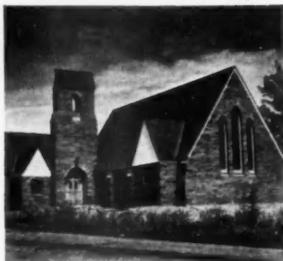
A JOB TO BE PROUD OF. The uniformly good color and appearance of Atlas Mortar do much to enhance the beauty of the church.
