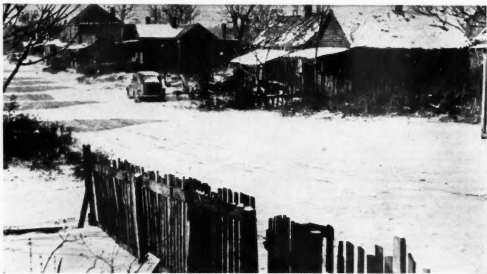
TYPICAL SLUM AREA of Indianapolis will be rebuilt by private enterprise. Redevelopment Commission clears land, saves tax money
