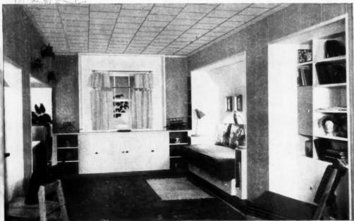
This effractive room was built in wasted attic space. Walls are J-M Plank in Buckskin Tan. J-M Ceiling Panels are Ivory. Notice the broken-joint ceiling treatment which saves time in application.
