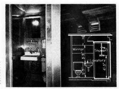
Bathroom walls are marine plywood. The ventilating panel is above and to the left of the fluorescent fixture. Air is channeled through louver in the exterior wall. The lowered ceiling in the shower stall forms the duct
