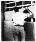
Applying panels horizontally over furring strips above studs. Nails placed in the inch tongue are covered over by the joining panel, leaving no marring of the
