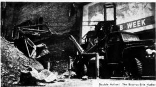
tions: the first is the conventional agshavel action of the dipper movag through its digging arc; the second, separate horizontal strake, obtained telescoping the boom. I
