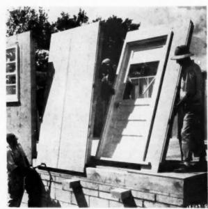
Plywood sheating on sections is engineered to overlap level of the finished floor, providing a weather-tight seal
