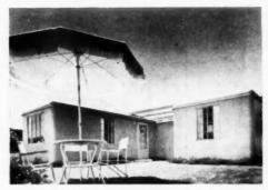
Windows are steel casements, equipped with roto-type hardware and screens. A terrace roof is provided, made of Corrulux and mounted to a beamed construction. A wide choice of interior and exterior finish color is available
