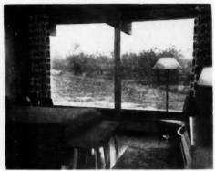
Floors are asphalt tile over a cement slab. Fixed glass, wood ceilings, and plywood walls carry out the ranch design
