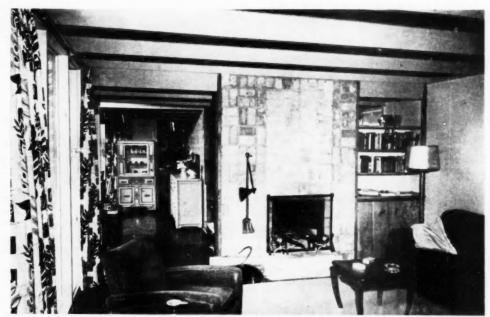
Facing of the fireplace and the stairwell are made of the brick panel. The grouted side of the panel is covered with gypsum board when used as a partition. Back side of the fireplace accommodates handy bookshelves. Ceiling beams are the steel joist boxes used to support floors of 3-inch slabs of precast lightweight concrete
