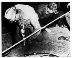
PORTABLE TOOL EXPERT from Skilsgw, Inc., uses Skil drill with hacksaw attachment to make pocket cuts for outlet boxes
