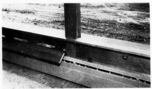
Ventilating panels are located between the window stool and the baseboard heating unit. Front of sill is faced so rain cannot enter through the ventilator
