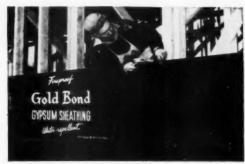
Fireproof Gold Bond Gypsum Sheathing gives extra strength, too. Racking tests prove these big knotless panels give greater structural strength than other commonly used sheathing materials. And the core of gypsum rock is asphalt-treated for increased moisture resistance.
