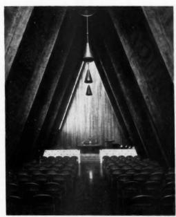
Inside surfaces of the hemiock boards were kerled every inch. thus hiding joints and giving acoustical value. Light comes not only through glass panels over chancel but also from glass panels at rear of nave. The building has radiant heating from copper tubes imbedded in the concrete floor
