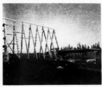
Laminated beams made up of 12 thicknesses of 2x7inch Douglas fir form the skeleton and are set on 8-foot centers. They are left exposed on interior. 2x6-inch hemlock tongue and groove boards are applied over beams and form the base for metal foll insulation
