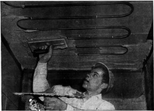
Extra-strong, lightweight coils of Bundyweld Tubing are easily mounted onto ceilings.
