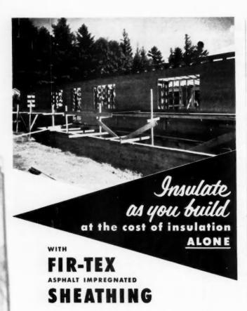
No home is modern without being insulated. In new construction Fir-Tex asphalt impregnated sheathing not only seals homes against heat, cold, dust and noise but also has greater bracing strength than ordinary sheathing. For better homes for your customers, recommend Fir-Tex sheathing. Two types-large sheets 4 feet wide up to 12 feet long and horizontal type 2 feet by 8 feet.
