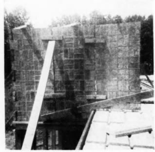
Close-up of panels after they have been lifted into place and temporarily supported by beam and bar
