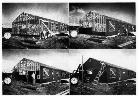
Two-hour operation sequence, indicating the speed at which gypsum sheathing can be applied to the framework of house. In one hour's time, over half of the material had been put in place by the 4-man crew. By 10:00 o'clock, the complete sheathing operation had been finished
