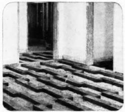
Now, with new methods of laying oak flooring over concrete slabs, builders of low-cost homes are able to include oak flooring in their plans. This is important because 85% of all prospective homeowners want oak flooring. (Laying oak on screeds set in mastic has been approved by FHA.)
