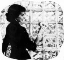
ANSWER . . . Install PC Glass Block panels. They are very easy to put up. They involve no wood or metal sash to rust, corrode, warp, decay or rot: eliminate periodic painting and puttying. Panels are easily cleaned as large, smooth units—not small panes. They stay clear and clean langer.
