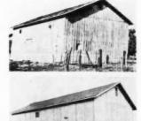
Here's a picture story of the rejuvenation of a 70-year-old barn near Monica. Illinois, which, before remodeling, gave the impression of being hopelessly dilapidated. The framing lumber was still sound, however, so the owner had the building straightened. He then covered the sidewalls with large sheets of as-bestos-cement board.
