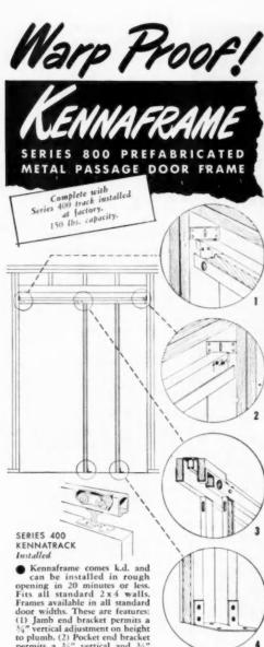
to plumb. (2) Pocket end bracket permits a 3/4" vertical and 3/4" horizontal adjustment to plumb
