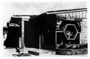
Used brick or rough unpainted lumber comprise the material surrounding the store fronts. Adobe is also used. All buildings rest on concrete slabs. The casual way in which the materials and joints are combined contribute to the charm and atmosphere of the center
