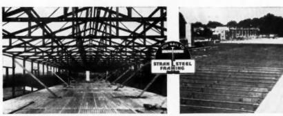
Non-combustible Stran-Steel framing members were used for exterior walls, interior partitions, roof trusses, and floor joists in New York State Conservation Department building at Sherburne, N. Y.
