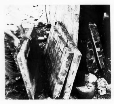
A solid layer of grout covers the "inside" surface of the panel. Rods used primarily for handling purposes can be seen protruding from the horizontal and vortical sides of the panels. Brick is Chicago treated common brick in banketweap pattern
