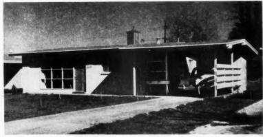
Use of "revolving" plan gives buyer choice of three elevations. In this example, breezeway connects with carport and storage room; also serves as cover for water heater, washer connection and laundry tube, installed on outside concrete platform
