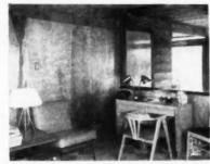
Office window is the only glass area facing the front of the structure. Heavy beam construction can be seen at the top of the side wall. Piywood panels cover all walls
