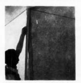
Cement is spread on each side of the corner and Peri-A-Bead is placed in position by holding one end near the top of the corner and pulling the bottom end slightly away from the corner
