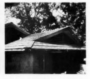
Hot air is exhausted through these louvers. Cool fresh outside air is pulled in through open windows. Result: temperature in house drops 10 to  $20^{\circ}$ .
