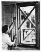
ATTACH INSIDE FINS — To complete the installation, apply the inside metal fins at head, sill and jambs. Fins fit under the lip of the steel frame and are nailed to the studding. This insures a tight weatherseal all the way around the window.
