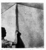
Perf-A-Bead is even seated by running the hand up and down the outside nose of the corner. Applying pressure to both sides of the paper flanges forces out excess cement at the sides
