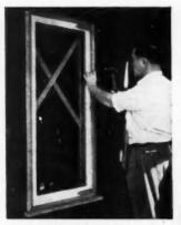
ATTACH OUTSIDE FIRS — Next, grooved edge of the fin fits over the edge of the steel frame. The flat surface of the fin is nailed to the sheathing. Exterior trim can now be applied.
