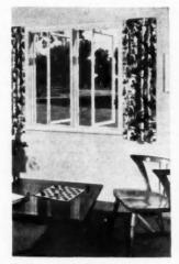
Flexivent units installed on end in casement position. Double glazing panel fits on outside of sash
