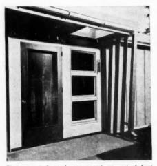
Flexivent unit in stack arrangement, as part of front entrance design
