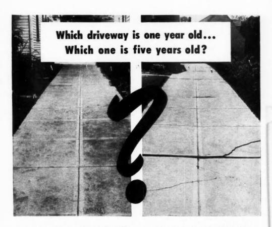
BOTH driveways are located in the same city, and subject to the same climate conditions. You would expect that the cracked and broken driveway had been built five years ago, and that the one with unbroken paving had been built recently. Actually the reverse is true. The one on the left was constructed five years ago with American Welded Wire Fabric reinforcement; the one on the right was built a year ago without reinforcement.
