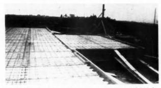
Reinforcing mesh is laid over the blocks prior to pouring the two-inch finished concrete slab. Flooring system is rated to withstand a four-hour fire and water test
