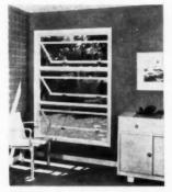
Three units in stack arrangement, with sash in awning position
