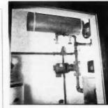
Compact arrangement of all the apparatus required to provide hot water radiant baseboard heating fits into this small utility room in the Des Plaines Villas homes. Heart of the system is the booster pump which circulates the hot water from the boiler through the baseboards
