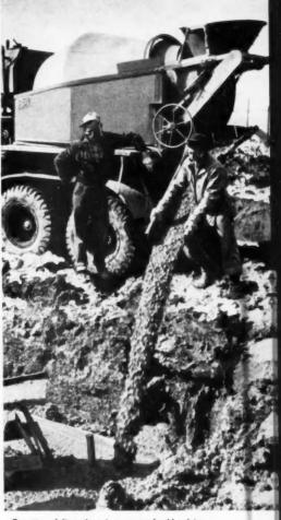
Operators deliver the mix warm and add calcium chloride if the builder requests it. After the footing is poured, straw will be placed over the concrete to protect it from freezing
