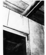
Header is cast with V-joints to match panels. Special hangers are nailed to a full size panel and support the header. The header has the necessary steel reinforcing cast into it
