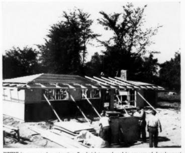
HOUSE in process of construction. Sandwich-type of roof in process of development
