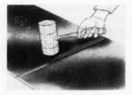
**13.** The cross seam is malleted down flat. to produce a flat locked seam of the same type as the vertical seams of the roof. Cross seams must be staggered. as shown in step 7. to avoid undue thickness of terne metal roofing on the vertical flat locked seams of the roof
