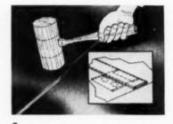
**6.** The single locked seam is now malleted, folded side down, flat against the roof, producing a flat locked seam
