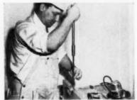
"I figure a door and jamb with 3 hinges takes 2 minutes to fit, 6 minutes to mortise and another 2 minutes to screw hinges. That's 10 minutes a door – 6 doors hung an hour."
