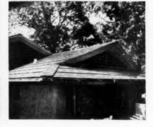
Hot air is exhausted through these louvers. Cool fresh outside air is pulled in through open windows. Result: temperature in house drops 10 to  $20^{\circ}$ .
