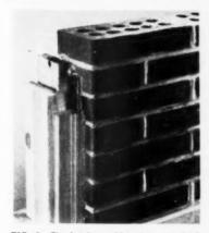
FIG. 9-The brick mould is then attached. leaving at least 1/4-inch clearance between mould and masonry jamb
