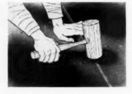
9. This type of seam is malleted down flat against the roof, producing a flat locked seam of the same type as shown in the first six steps. The preferred method of seams is to cut the terme into strips as long as can be handled in a brake to make the bends shown in step one
