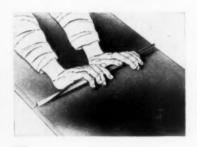
**12.** Position the two strips to be joined by the cross seam so that the half-inch flange of one strip is adjacent to the oneinch flange of the other strip. and the top half inch of the one-inch flange is bent down over the half-inch flange
