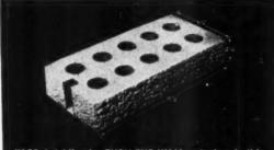
"SCR brick"—the THRU-THE-WALL unit that builds solid brick homes for the cost of frame. Developed by the Structural Clay Products Research Foundation. T. A. Hutchinson • Hutchinson Carey Homes, Denver, Colorada
