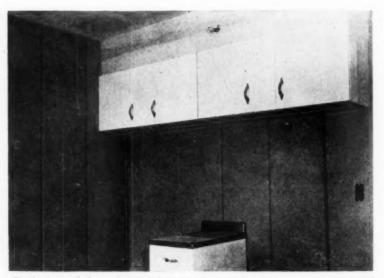
The kitchen soffit has a frame skeleton and is covered with plaster board. The metal cabinets are fastened to the panels as in standard framing
