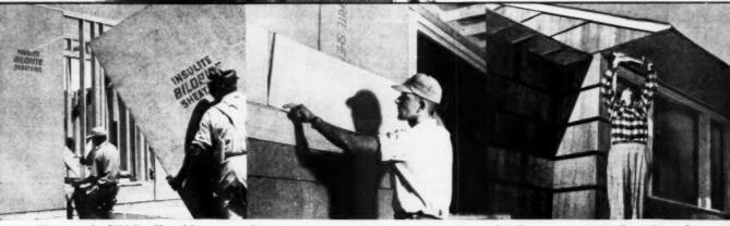
First, apply Bildrite Sheathing-cut sheathing time as much as 43%. One carpenter can sheath 1,000 sq. ft. in 8 hours or less. Saves corner-bracing (4-foot Bildrite was the first insulating sheathing to be accepted by F.H.A. for use without cornerbracing). No building paper needed . . . Bildrite is waterproofed throughout. Saves material-no matching loss or waste.
