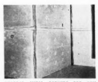
AB13263—METAL CORNERS FOR DRY WALL—The Richkroff Co., Dept. AB, 228 N. La Salle St., Chicago I, III. Richbead consists of a metal angle glued to joint tape. It comes in two types, one for exterior corners and one for interior corners, giving a lasting finish, clean lines and true angles to corners. Available in 1/2-inch and 1/4-inch sizes, Richbead is simply cut and fitted, does not require special tools. Photo shows completed application at interior (left) and exterior (right) corners.
