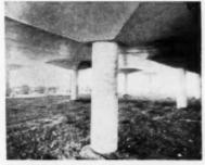
AB13020-BOOTH NO. 246-FIBRE CON-CRETE FORMS—Sonoco Products Co., Dept. AB, South St., Hartsville, S.C. "Sonotube" concrete forms made of laminated fibre provide a fast, economical method of constructing concrete columns, cylindrical voids. They are furnished in 19 standard inside diameters from 3 to 24 inches. The forms can also be used for upright piping by pouring concrete between two tubes of different diameters. Two coatings are available, for clean finish or form on column.
