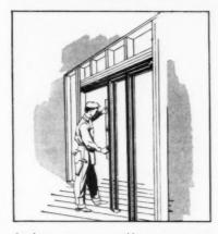
It takes a carpenter several hours to trame-up a rough opening, and install hardware for a disappearing door. But at best, he can't guarantee the job, simply because warpage often ruins the installation. Exposed to the ravages of heat and humidity, horizontal wood members-and the door itself-tend to buckle and bind.
