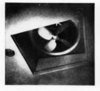
**Compact Package Fan** rests on attic floor of Pace Setter House. This unit is ideal for homes with low roofs as it requires less than 18" clearance.
