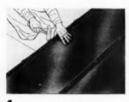
4. The second strip is installed with its one inch flange adjacent to the half-inch flange of the initial strip, and cleated down to the roof deck along its half-inch flanged edge
