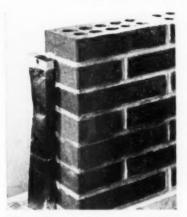
FIG. 4—Rough buck built into wall. Note that flashing material has been temporarily stapled back against the rough buck to keep it out of the way
