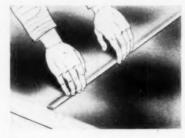
8. The next strip is laid overlapping the preceding strip with one half-inch flange facing downward, and the strips are locked together by sliding the downward turned flange of the second strip into the upward turned flange of the first strip. thus tightly locking strips together
