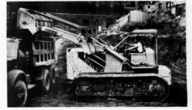
**Excavating dirt and rubble** from old building and loading to trucks is one of many jobs this Allis-Chalmers HD-20G tractor shovel handles fast because of its 175 net engine hp., easy maneuvering ability and big 4-yd, bucket capacity. Working on large housing projects, the 61,600-lb, HD-20G's economically dig a basement an hour *in any weather*, clear out trees, move big rocks.
