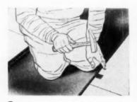
2. The initial strip is laid on the roof and attached by cleats hooked on the hali-inch flange of the initial strip, each cleat being fastened to the roof deck with two nails side-by-side on the width of each cleat
