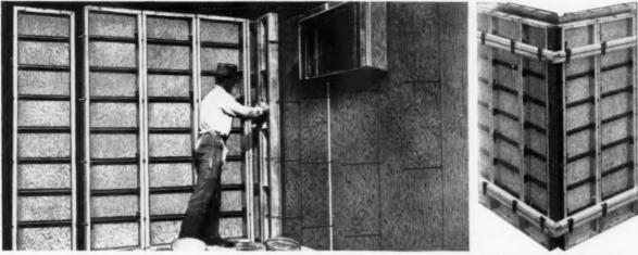
Starting at a corner, panels of the outside form are erected. Spreader ties are placed in position and anchored on the same connecting bolt, locking panels together.
