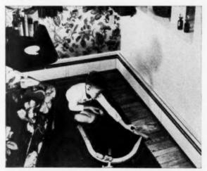
**HEATRIM PANELS.** Specifically designed for forced circulation hot water heating, these baseboard heating panels provide convected warmth throughout each room. The panels take the place of regular wood baseboards, allow use of virtually all the floor area. Panels can be installed free standing or recessed . . . are ideal for use under picture windows.
