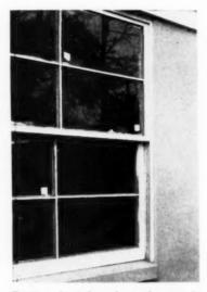
Exterior of window shows the stop in place. Sill and header units are precast. Builder does no cutting of the panels
