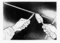
**14.** Solder all cross seams along the free edge, which must face downward with the flow of water on the roof
