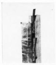
FIG. 3—Rough buck with flashing material stapled to it and buck anchors attached
