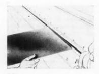
**10.** When a cross seam is unavoidable, one end of one strip is bent to a 90-degree flange one-half inch high, and one end of the other strip is bent to a 90-degree flange one inch high, using tongs or a cornice brake
