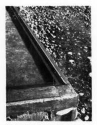
Metal channel, fastened to the foundation, aligns the panels. A similar channel is also at the top of the panels
