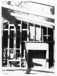
POURED CONCRETE CHIMNEY and fireplace using lightweight plaster aggregate
