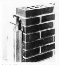
FIG. 10-The space between the brick mould and masonry jamb is then filled with caulking
