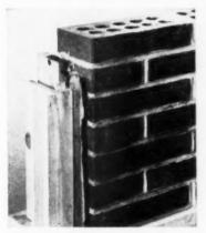
FIG. 7—Window frame is then put into position, plumbed and shimmed if necessary
