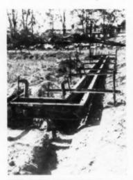
STEEL INTERLOCKING FORMS for concrete walls. Note special leveling device
