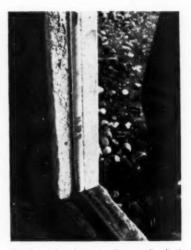
Tubular spline between the panels eliminates shear stresses
