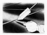
**15.** Solder all vertical flat locked seams along their free edges, and a finished leakproof metal roof results
