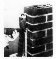
FIG. 5—Applying bead of caulking compound between the flashing and brickwork. Since the jamb slots in the "SCR brick" are not used here, they may be filled with mortar by the mason as he builds the wall
