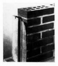
FIG. 6—Flashing material straightened out and formed around caulking bead
