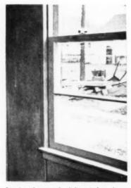
Interior photograph of the window shows that frames are eliminated. Wood sill and window stop are the only trim items. Stop covers pressure type sash balance
