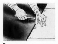
3. The back end-tab of each cleat is bent back over the nail heads and malleted flat to protect the nails and the terne metal strip subsequently laid over them
