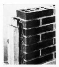
FIG. 8—Flashing material is then doubled back to form a loop and tacked or stapled to the face of the window frame
