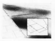
**7.** For shop fabrication, the strip may be cut into eight or ten foot-lengths, and formed on the brake. The half-inch flanges are bent on the long sides of each strip, and the flanges bent upward on one long edge—downward on the other long edge. Upturned flanges are cleated down
