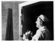
"You can forget all about hand chiseling and shims. You don't even have to figure out the location for the hinges. The templet does it for you."
