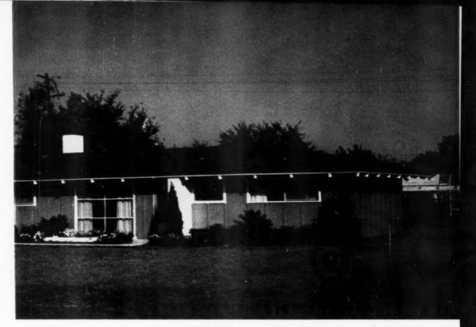
FRONT VIEW: low sweeping lines dominate the exterior. Vertical wood battens on walls cover joint of asbestos board siding. An arresting motif is found in the brick pier adjoining the front door
