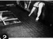
Place the required amount of reinforcing in the panel and be sure to provide suitable means to hold it in the proper position.
