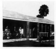
Exterior of house is produced by concrete bricks of red tones veneered to the block columns
