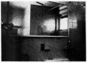
Large medicine cabinet has sliding mirror doors. Cabinet is shop built by builder. Mirrors are shipped ready for builders' installation
