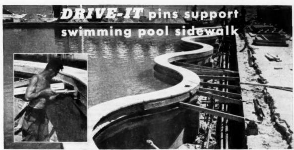
DRIVE-IT was used to help build a tunnel alongside the swimming pool at the Sans Souci Hotel, Miami Beach, Florida. The tunnel was needed to give workmen access to repair leaking pipes without the need of tearing up the sidewalk each time. The curved 1/4" angle iron was anchored to the concrete wall with DRIVE-IT. Cross (1/4" "1")
