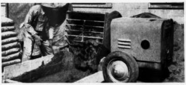
Jacoer Multi-Blade 31/2 Ft. Power Hoe -- the heavy duty small mortar mixer. 61/2 ft. size for larger jobs.
