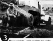
Place concrete, using quality mix yielding durable walls. Use care to prevent honeycombing, especially along bottom edge.
