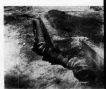
Regular sheetmetal elbows carry the large tube ducts around the perimeter of the building. Duct work is tied to the foundation wall and grouted before the slab is poured
