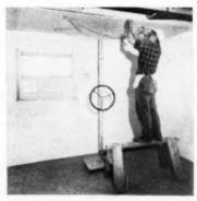
The entire jack rests on a heavy steel base with four steel casters angled inward, assuring levelness and portability. Gypsum Ceiling Jack Co., Dept. AB, 112 22nd St., N. E., Cedar Rapids, Iowa.
