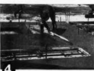
When concrete has partially hardened, trowel, float or brush the surface to obtain the kind of smooth or textured finish desired.
