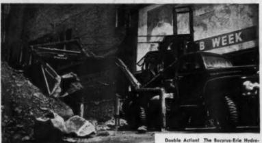
Double Actions him bucyrus-trie mydre-hoe gives you two separate digging actions: the first is the conventional dragshovel action of the dipper mov-ing through its digging arc; the second, a separate horizontal strake, obtained
