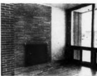
Living room fireplace wall has built-up hearth. Windows in the living room are floor to ceiling units. Above is fixed glass, below are sliding units that provide ventilation. Front entrance is to the left of the brick partition
