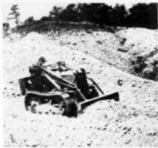
The tractor is particularly suited for backfilling foundations, winch operations, cleaning ditches, landscaping, moving concrete, industrial material handling. As is seen in the illustration, it is also useful in light bulldozing operations. The unit is rated at 21.85 drawbar horse-power, and 26.36 belt horse-power. The Oliver Corp., Industrial Div., Dept. AB, 19.302 Euclid Ave., Cleveland, Ohio.
