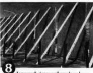
Temporarily brace wall panels as shown before adding reinforcing and forms for the columns that will tie the wall together.
