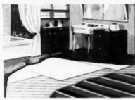
Homosote Underlayment is nailed directly to the rough flooring. No felt or pad is needed.
