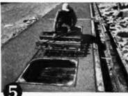
Incorporate decorative designs before the concrete hardens. The illustration above shows workman adding a low-relief design.
