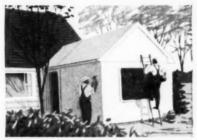
◆ Homasote Big Sheets (up to 8' x 14') save time and labor in the sheathing of roofs and exterior walls.
