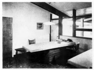
Wood office partition is used when it does not correspond to the beam module. Material is full 2-inch random width "V" jointed planking. Splines were used to eliminate shear action of the wood members. Builder claimed splines set in dado are easier to erect than using 2-inch t&g material
