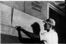
Cut sheathing and under-coursing time in half with this approved system for double-course sidewalls. 4-ft. Bildrite eliminates need for corner-bracing and building paper. Shingle-Backer applies faster, easier than wood under-course shingles. Provides deep shadow-line. System has tremendous holding power. Test wall was exposed to 250 m.p.h. winds. Not a shingle came loose!
