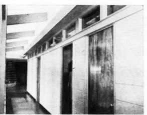
The roof pitch is 2.4 in 12. This pitch gave same angle of cut to all blocks in the interior partition walls. Only three basic cuts were needed for interior wall construction
