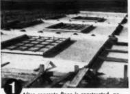
After concrete floor is constructed, position edge forms and frames or forms for openings. Apply bond-preventative to floor.
