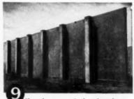
Place the concrete in the column forms and allow it to cure properly. Then remove the forms and braces. Wall is now completed.
