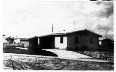
Two types of carport can be added to the basic one-plan house. Driveways are graveled. Cost of the carport is \$600. The barrel tiled roof adds \$248 to the cost of the house. The living room has cross ventilation which builder claims takes the place of an open screened porch. Jalousie windows are used throughout the house
