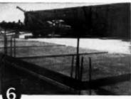
Cure the panels until concrete has attained the desired strength. Then carefully remove all the edge and opening forms.
