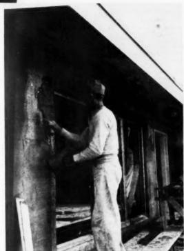
Workman is applying brown coat of stucco to block. A second coat followed by two coats of paint finish the exterior
