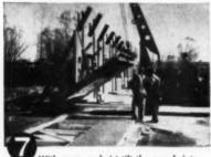
With crane or hoist tilt the panels into position in wall. Grout joint between the wall and the floor to make it weathertight.
