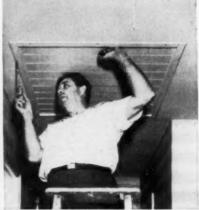
Above: Screw-fasten the automatic shutter to ceiling, with metal trim covering edges—no re-plastering.
