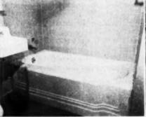
Bathtub in all 1953 models has heat duct placed under it to warm tub. Tub is raised one inch so warm air can also heat room
