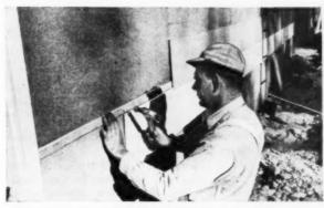
3. Next, apply 11¾" Shingle-Backer and asbestos-cement shingles. System is self-aligning. No special nails or fasteners needed. Increases shingle exposure from customary 10½" to 11"... gives 5% greater shingle coverage. Provides cushioned base to reduce impact breakage... reduces shingle waste as much as one-third. Increases insulation value of wall. Waterproofed throughout with asphalt.
