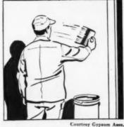
To obtain full, uniform coat, sizer should be brushed on with semi-circular stroke. Primer and/or sealer give bonding surface for paint
