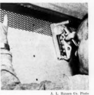
Tacker Saves Time Worker using onehand tacker to attach cornerite for reinforcing walls and concrete. Operating as fast as the hand can grip and squeeze, tacker also saves time by leaving other hand free to hold work.
