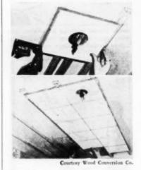
Left: First fiber tile is applied to starter strip. Entire first row should be applied across ceiling before second row is installed on opposite side of strip. Second row (above) takes shape opposite starter COUTER
