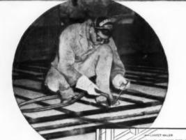
Zonolite Insulating Concrete under radiant heat pipes promotes efficient operation of heating system, better temperature control, saves fuel.
