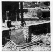
STEEL access panel to provide access to drainage pipe in basementless building. Installed with metal wall around area of panel
