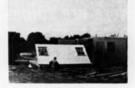
12 Men here are raising exterior panel that will complete the rear wall of this home with full basement. Quality control in factory insures "fit" on the site
