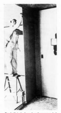
One-half inch. long length gypsum lath with grooved or square edges is set into the floor runner, and tie-wired or clipped to the ceiling runner. Adjacent laths must be butted tightly
