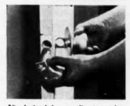
After boring holes according to template guide, slip inside knob assembly into hole in door face, followed by slipping lock into aligning tube. Then insert aligning pin to hold these two components in proper position
