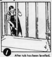
place roll of mastic around rim for waterproofing. Also, butter studs with mastic before setting glass panels.
