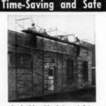
No wonder builders like balanced Safway steel scaffolding! It's engineered for structural stamina-Eav-to-assemble units speed erection of scaffolding and make dismantling simple. Pictured here is the lowest cost steel scaffold on the market for loads up to 50 lb. per sq. ft. with heights up to 40 ft.
