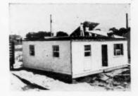
15 With first roof section in place, second section goes up to meet it. Factory equipment such as large tenon saw makes 23 notches in raiter at one time
