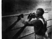
For deep shadow line. nail strip of plywood or 3/2-inch furring strip along top edge of each course and (below):
