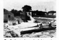
9 Trailer trucks are loaded to conform with order in which panels and units will be required on the site. Care is taken to preserve finish of surfaces
