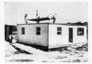
14 Carrying first roof section to its position. Notched rafters have been prepared to receive roof sections and speed erection
