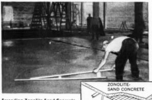
Screeding Zenolite Sand Concrete, grade-level floor. United States Tobacco Co., Chicago, III. Ideal concrete for one-pour floors on grade, or for lightweight upper story floors.
