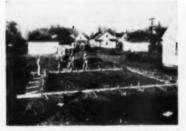
1 First step in erection of prefabricated basementless home. Crew stakes out ground area for slab. Pipes and conduits are put into position
