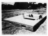
8 Laying finish floor for home with basement. Panelized sub-floor has already been installed. Finish flooring is laid on the job
