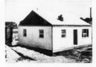
17 All roof sections are now in position and being nailed down. Pre-assembled gable ends will be moved into position next to complete roof structure
