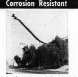
Weather and corrosion won't hurt the Safway scaffolding used in this 185 foot ski slide in Los Angeles. It's corrosion and rust resistant. Special phosphate bath converts surface of Safway steel scaffolding to non-metallic oxide. Baked-on weather resistant paint gives exite protection.
