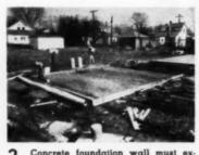
Concrete foundation wall must extend below frost line. Depth varies with climate of location. Inside area is filled with 4 inches of pea gravel
