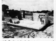
10 Trailer is backed up to one corner of home. Panels are erected directly from truck with no rehandling. First corner is being erected
