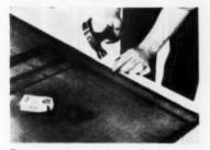
First step in attaching plastic saran screening is to start at top corners to hold material in place. Nail tacks or staples about  $1\frac{1}{2}$  apart
