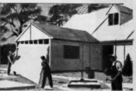
• Hemasote Big Sheets (up to 8' x 14') save time and labor in the sheathing of roofs and exterior walls.
