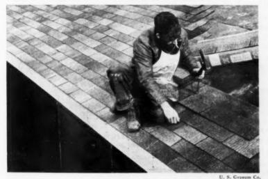
Laying three-tab, square butt asphalt strip shingles with cutouts centered over tabs from course to course
