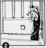
Set the plate at the back of the tub first. Then merely nail through plasterboard flanges and use special clips supplied.
