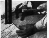
To make your linoleum underlays hold tightly and lie flat permanently, secure them with Hassall annular-threaded linoleum underlay drive screws. They are cement-coated for maximum aripping power. Heads are flat countersunk type. Size: 11/4" x #3 gauge. State quantity when writing for prices to:
