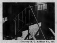
Install railing in three simple steps: (1) Build concrete forms to fit stock sizes of railing. (2) Set rail in forms, plumb and level. (3) Pour concrete.
