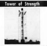
Workmen safely reach into the sky 75 feet high. They're using Safway scatfolding to dismantle a heavy steel stack in Minneapolis. Safway carbon steel frames are solidly joined with using nuts to tubular steel cross braces for strength. All welds are made by master welders.
