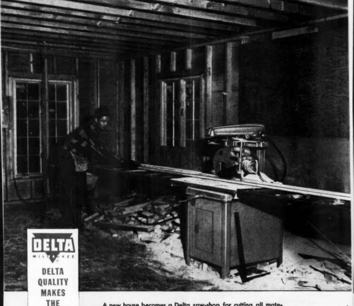
A new house becomes a Delta saw-shop for cutting all material. An 8-foot roller conveyor section solidly mounted at each side of the saw makes work handling easy.
