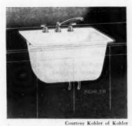
Contrest Konter of Konter Enameled iron laundry tray has round corners to protect fabrics, swing-spout mixer faucet, provides attractive as well as efficient laundry facility. Designed for building into counters or cabinets, tray measures 24"x21" length and width, with 13" deep basin. Accessory metal frame makes counter installation easy
