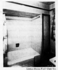
Attractive bathroom wall installation is made with structural-type glass. Material has good resistance to moisture and
