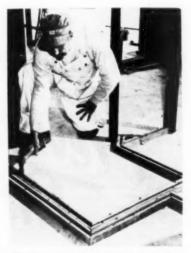
The first step in the installation of a twoinch solid gypsum partition is to secure a grooved wooden runner or  $\frac{3}{4}$  inch steel channel to the floor according to the partition layout with nails or adhesive
