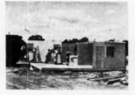
11 Center bearing-wall in position with first ceiling sections temporarily located. Note room size panels with doors, windows, and trim already installed
