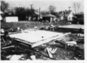
4 Fiberglas insulation is laid around rim. Entire surface is covered with wire mesh, and concrete is poured. Slab is insulated and vapor-sealed
