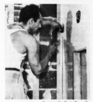
Courtesy St. Regis Paper Co. One all-plastic panel is set in place with cutout area for fixtures. Workman nails corner moulding to studding to provide firm anchorage. No backing or insulative material is used
