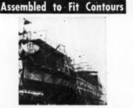
Standard Safway equipment is easily assembled to fit the curved bow and sloping sides of this vessel at the U. S. Navy yards. Only a few basic types of interchangeable members are needed to assemble scaffolds of any required shape and height.
