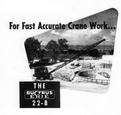
Erecting structural steel, pile driving, placing and removing forms, loading and unloading construction materials and equipment - these are just a few of the many construction applications of a Bucyrus-Erie 22-B crawler crane. And it can do each job for you at considerable savings in time and money. Here's why:
