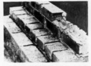
POOR WORKMANSHIP—likely to leak. Deeply furrowed bed joints and only partly filled head joints with no mortar in vertical or collar joints allows water to seep in and damage structure
