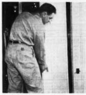
Plank is 16 inches wide to cover one stud space. has 16g joint for concealed fastening. Scoring is to resemble 6 and 10-inch alternating planks. Application here is a basement amusement room
