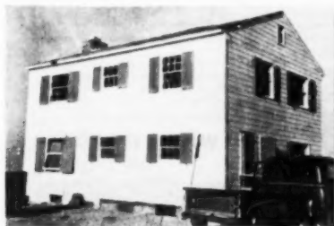
A mile-and-a-half from the bomb blast, the rear of a "typical" frame house looks virtually untouched . . .
