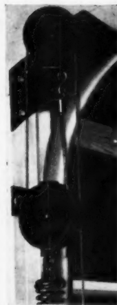
Steel cables operating in conjunction with enclosed pulleys and vertical springs counterbalance the weight of the doors.
