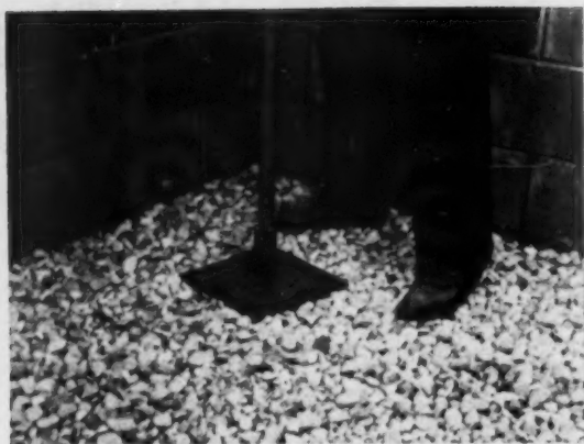
Compacting coarse granular fill before application of grout coat
