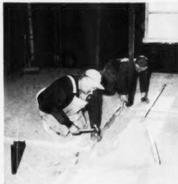
Step 1: Wood runner is fastened to the cement floor with concrete nails. Step 2: Rib lath is set into the centered groove in the wood runner and wire-tied to ceiling runners
