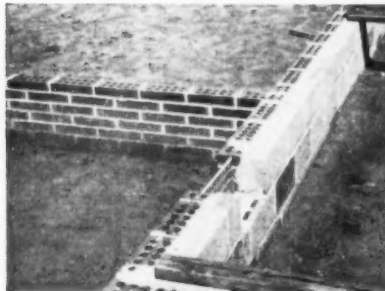
Four inch concrete block was used as the backup for the SCR brick foundation. The back-up for basementless job costs $100
