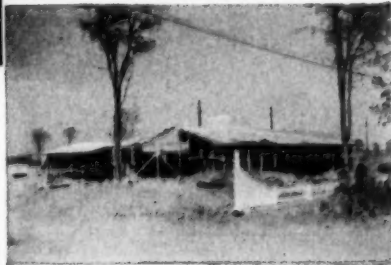
House in framing stage ready for surfacing
