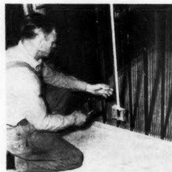
Step 4: Shallow electrical outlet is wire-tied to partition. Full line of shallow electrical switches, outlets is available
