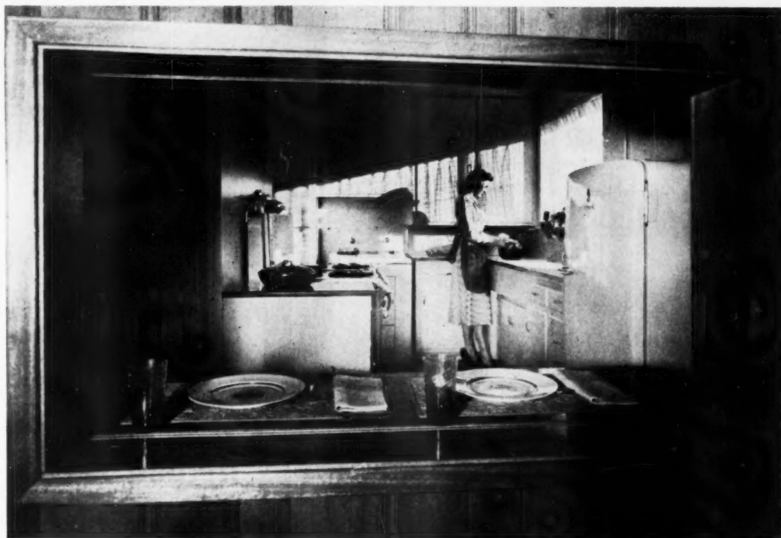
Kitchen side of the pass-through has an 18-inch by 8-foot long breakfast bar. Unit is large enough to accommodate four persons
