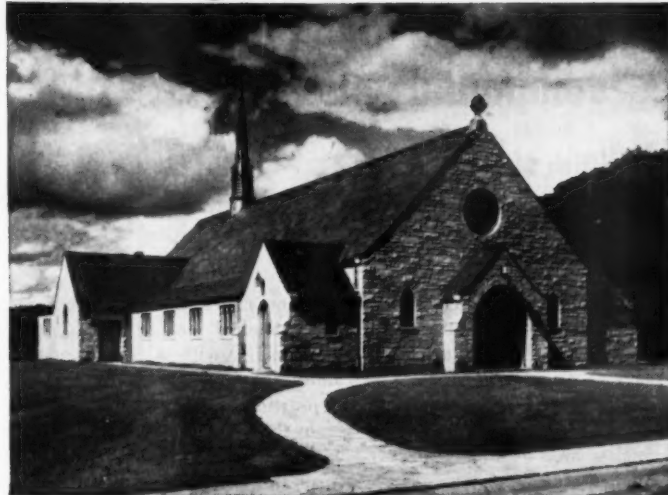
Saint Louis Roman Catholic Church, Princeton, Illinois: Zonolite Concrete provides a warm, dry, comfortable floor according to Rev. Father Edward M. Farrell. Architect: A. F. Moratz, Bloomington, Ill.
