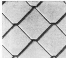
HEXAGONAL ROOFING SHINGLES A smooth-finished asbestos-cement shingle, applied in a diamond pattern.
