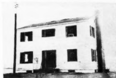
But the front, which faced the explosion, shows greater damage . . .
