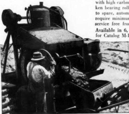
3 1/2 Auto-Loader, with Power-Shaker Hopper, loads while mixing, produces 12 to 15 more yds. daily.
