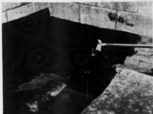
Membrane dampproofing being applied over grout coat
