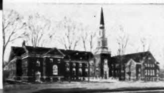
Adas Israel Synagogue, Washington, D.C. . . . Zonolite insulating Concrete used under radiant heating coils in the floors. Architect: Frank Grad & Son, Washington, D. C.
