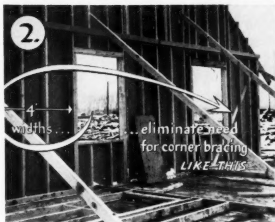
Insulation board sheathing, like that applied vertically on this Mills & Sons home, is accepted by FHA for use without further corner bracing. can be used as the only sidewall insulation
