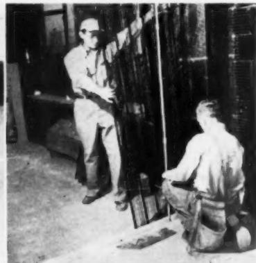
Step 1: Wood runner is fastened to the cement floor with concrete nails. Step 2: Rib lath is set into the centered groove in the wood runner and wire-tied to ceiling runners
