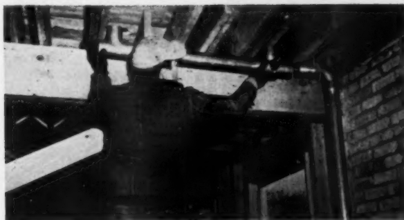
One man can easily lift 16-pound copper assembly into place
