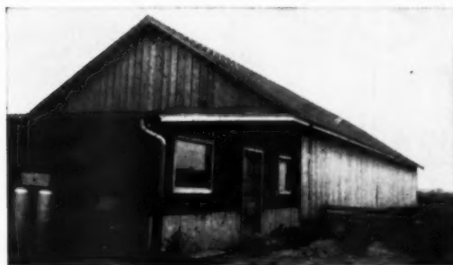
Heat inside the barn during winter is maintained by the manure pack. Concrete barnyard is important in the loose housing system. Cows enter the milking parlor at the doorway on the right
