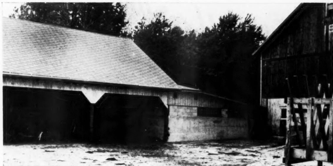
Heat inside the barn during winter is maintained by the manure pack. Concrete barnyard is important in the loose housing system. Cows enter the milking parlor at the doorway on the right
