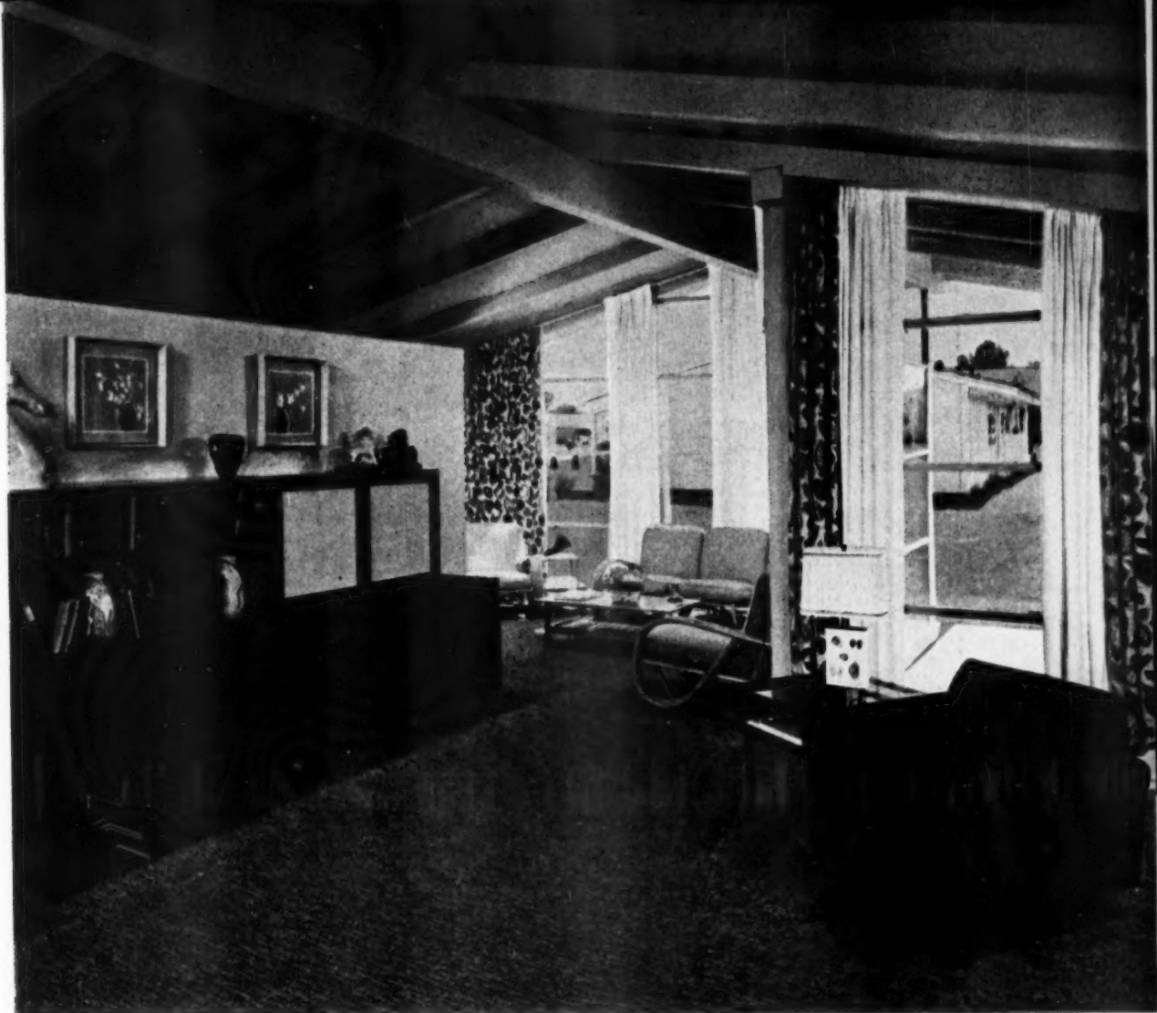
Stub walls of kitchen make possible a continuous ceiling pattern over main living areas of house
