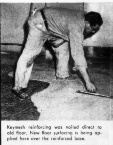
Keymesh reinforces plaster or any base for wall or floor tile assuring maximum crack resistance.
