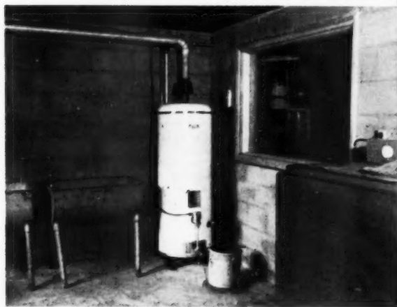
Window separates milk room and milking parlor. Heat for the two rooms is from the water heater
