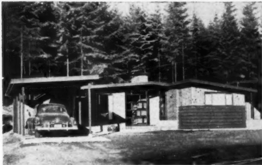
Semke uses various exterior finishes. Natural finish vertical cedar siding gives this model individuality. Front door treatment is striking, sometimes is done in single plate glass, without muntins
