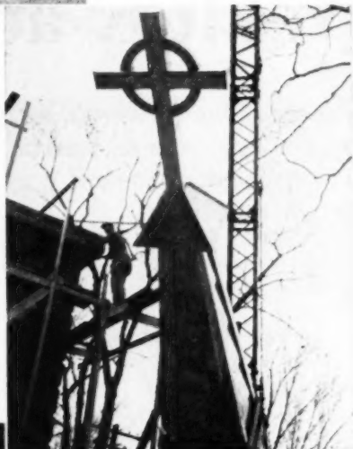
Steeple was first lifted to upright position. A rope was tied to lower end of steeple to keep it from swinging
