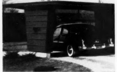
Carport, glass areas, chimney and roof lines that when considered collectively produce a well designed modern exterior
