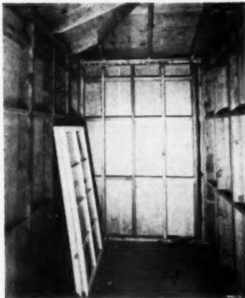
Interior of the storage car port shows the panelized construction of these houses. Panels are built at centralized locations hauled to the building site
