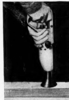
Anchoring wood sleepers to concrete
