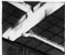
Aluminum ductwork is easy to handle and install. Won't rust, is a natural insulator, minimizes heat loss.
