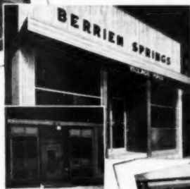
Before: left After: above. Kawneer village hall modernization.
