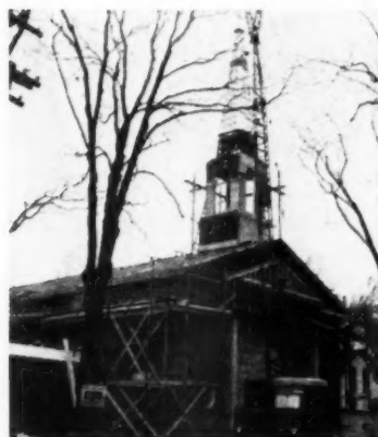
Steeple now in place is held by crane while carpenters fasten it to the belfry
