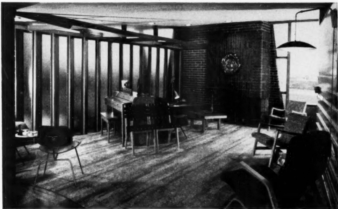
View in living room from dining area. Exterior wall at left consists of a series of vertical panels glazed with amber colored cathedral glass, which diffuses the east light and blots out the view of the adjoining house
