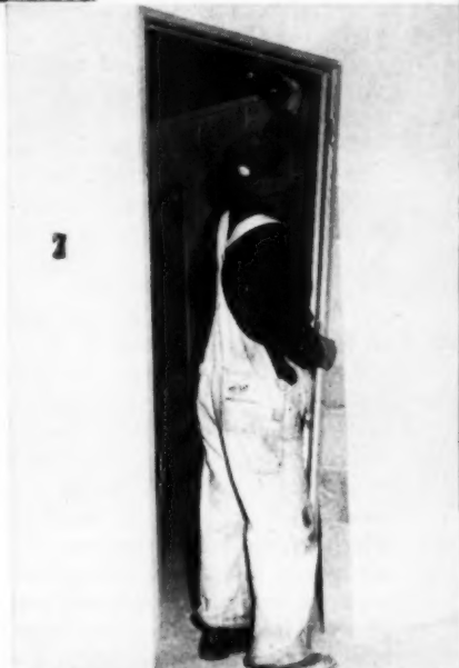
Aluminum door and frame assemblies are installed after the house is finished
