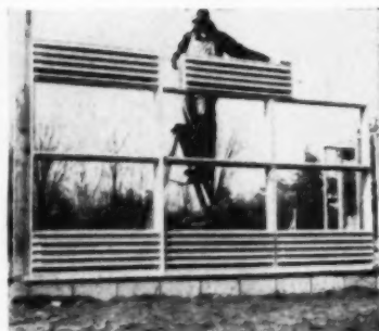
Stacking a louver unit into a window wall. Note channel in the end of vent unit (top)
