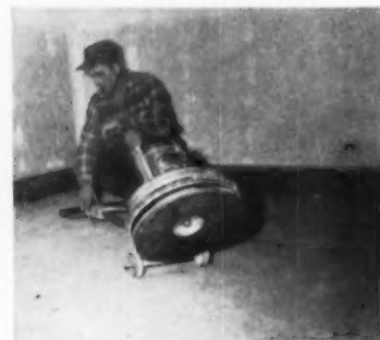
An open grit silicon carbide grain paper is used to cut through the droppings
