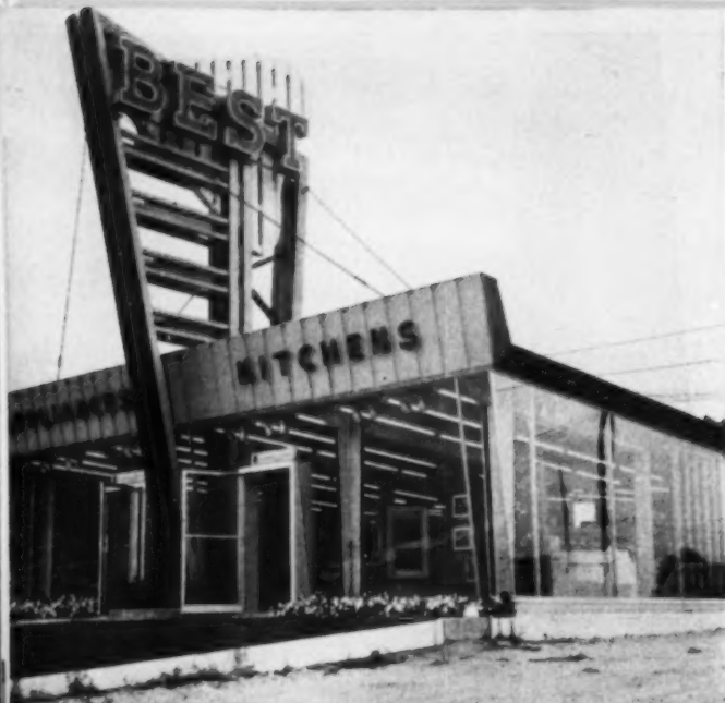
Dramatic facade of lumber dealer's specialty building is constructed of wood. Cement block and glass are the other materials used
