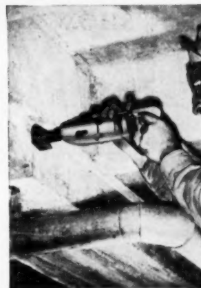
Anchoring steel fittings to concrete for pipe and duct suspension
