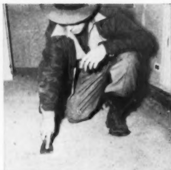
Bud Henson, Nathan Manilow's construction superintendent shows the old way of scraping a slab. The hand operation took six hours for a 1,000 square foot house
