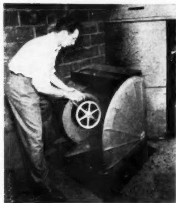
Installing the blower-filter unit is a simple one-man operation of three or four hours
