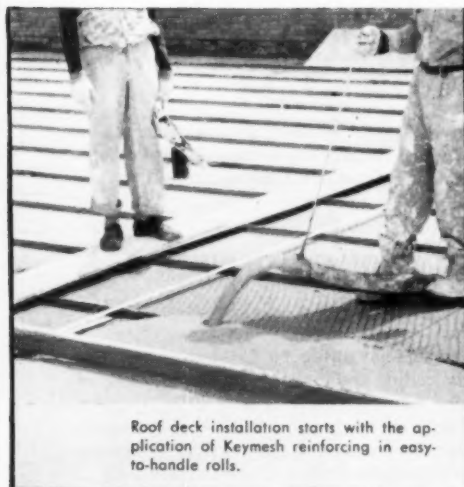
Keymesh reinforcing was nailed direct to old floor. New floor surfacing is being applied here over the reinforced base.
