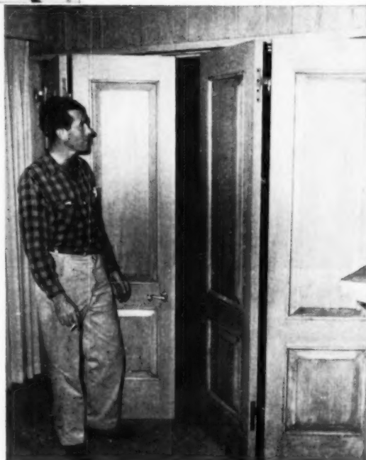
Close-up of door with raised panels produced on the special shaper. Bob Crowe himself inspecting the work.
