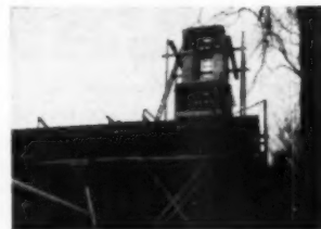
Bellry supporting steeple has large steel gusset plates at corners to insure stability. Steeple was bolted to top plate of bellry
