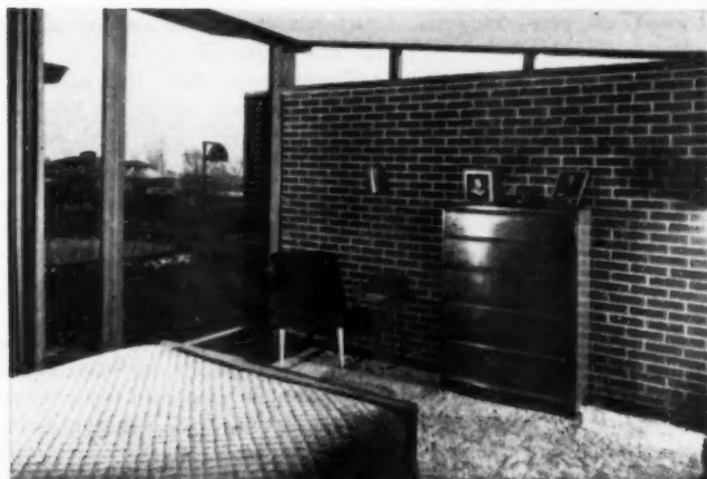
Master bedroom. Brick wall is of cavity type with 2-inch air space
