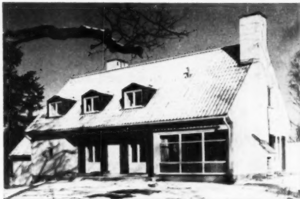
A typical Swedish home in which slabs of the new lightweight concrete form both floor and ceiling
