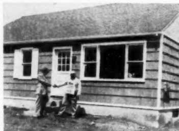
Finished sidewall creates appearance of double-coursed shake exteriors
