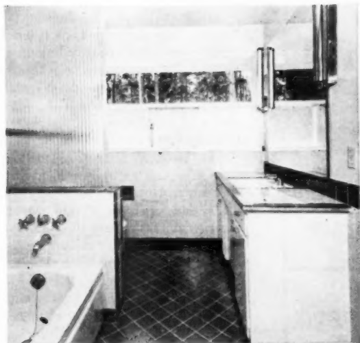
Center panel in outside wall swings out for ventilation. Obscure glass on either side, clear glass above
