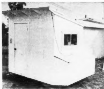
Crowe's portable job office has telephone, light connections, plan table, etc., and a storage box on outside.
