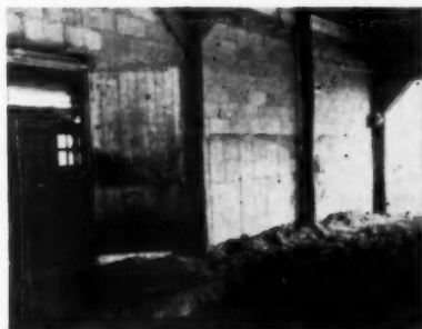
Exit doorway is raised for ultimate raising of the manure pack. Pole barn abuts concrete block structure. Farmer stores machinery in barn during summer
