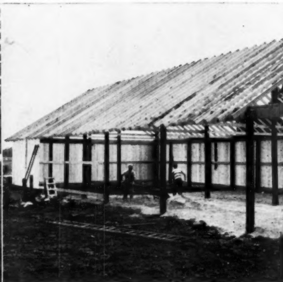
Floor for the pole barn is finely ground limestone. When packed it gives a suitable floor covering at little expense
