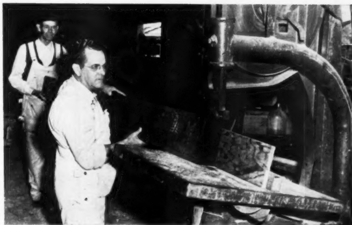
Straightening a door on the Pryor jointer.
