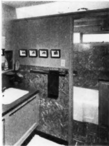
Wainscot and tub area are Rose De Brignoles Marble Panel. Wall at right (not shown) is Natural Walnut Marlite Woodpanel.
