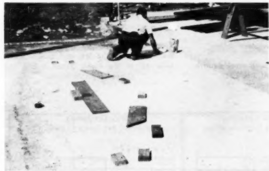
Scrap wood blocks nailed along truss outline for jigs
