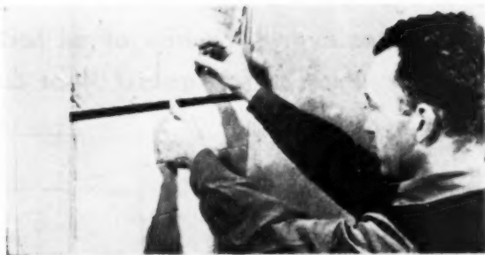
Setting an interlocking above the feature strip
