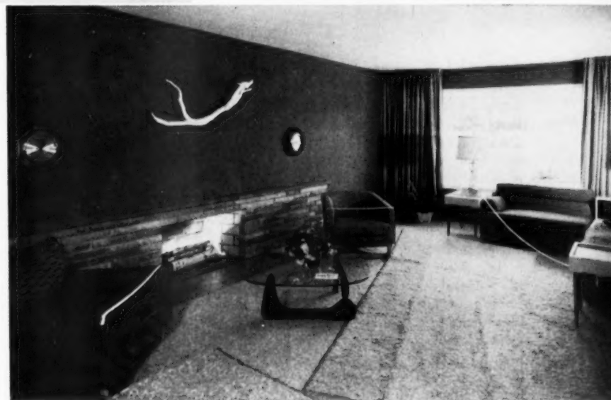
View across living room from steps shows long, low lines of stone veneer and flagstone fireplace. Note how builder uses extra cuttings of carpeting instead of the traditional building paper for his prospects to walk on
