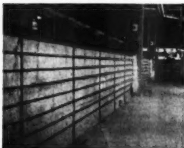
COPPER TUBING was specified for radiant heating panels that are installed in walls.
