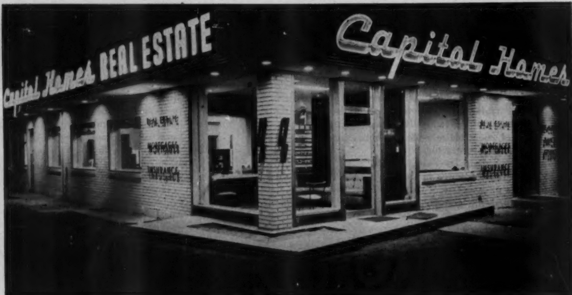
Night view emphasizes changes. Double-channelled neon signs and spots recessed in wide overhang concentrate light on entire exterior of store, keep it away from apartments above. Front, flagstone terrace being prepared for landscaping, is carried through walls into reception room floor
