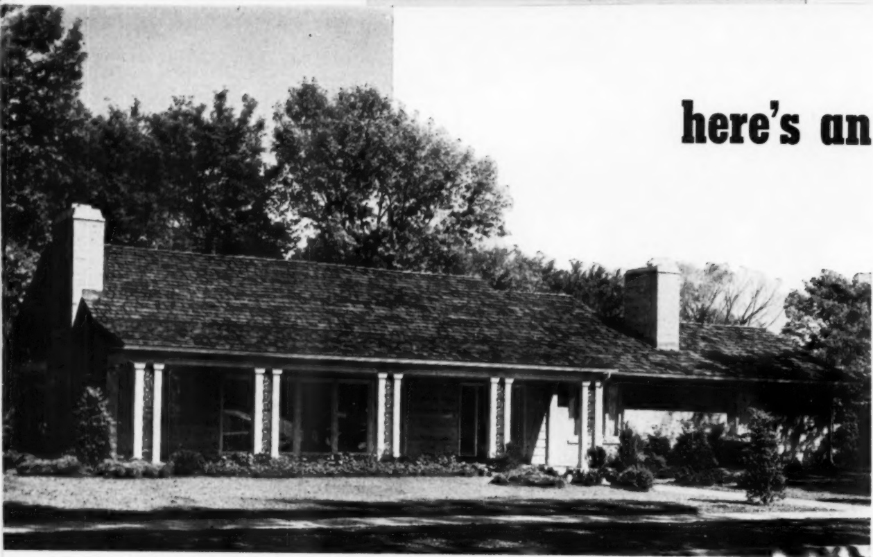
The finished woodwork of cornice and columns on portico, complements the rough texture of roof, siding and stone walls
