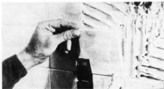
Fitting plastic tile around an electrical socket
