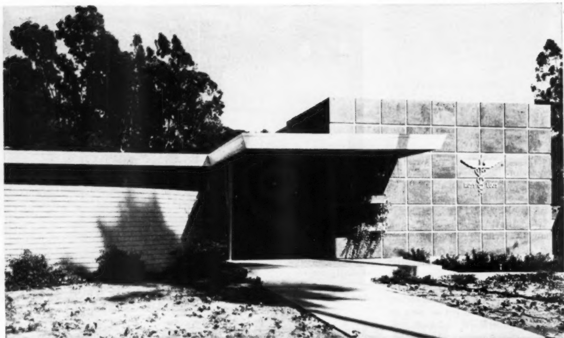
Detail view of exterior showing patio wall adjoining entrance
