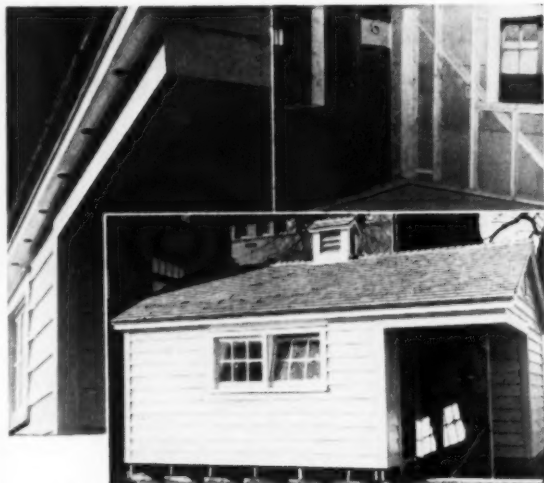
Detail views of model milk house indicating features of the construction used. View (1) shows the vented box cornice at eaves. View (2) shows a portion of the walls with an application of vapor barrier insulation. View (3) shows the covered loading platform portion of the milk house
