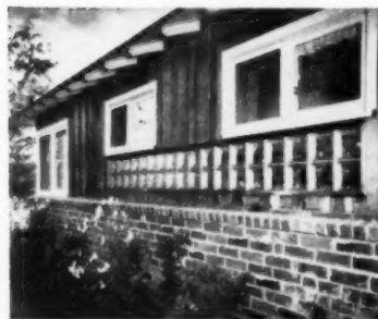
ON THE EXTERIOR—Glass block as a construction material blends well with brick and wood. In a kitchen wall, as here, permits daylight at the work counter.
