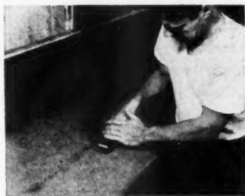
After removing paper separator, entire surface is firmly rolled with a steel roller
