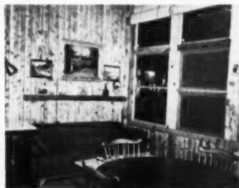
Corner of window wall has storm unit set as a fixed pane. Eight operating sash are included in the installation
