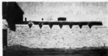
Seven diamond-shaped skylights project above roof line and slope to roof level
