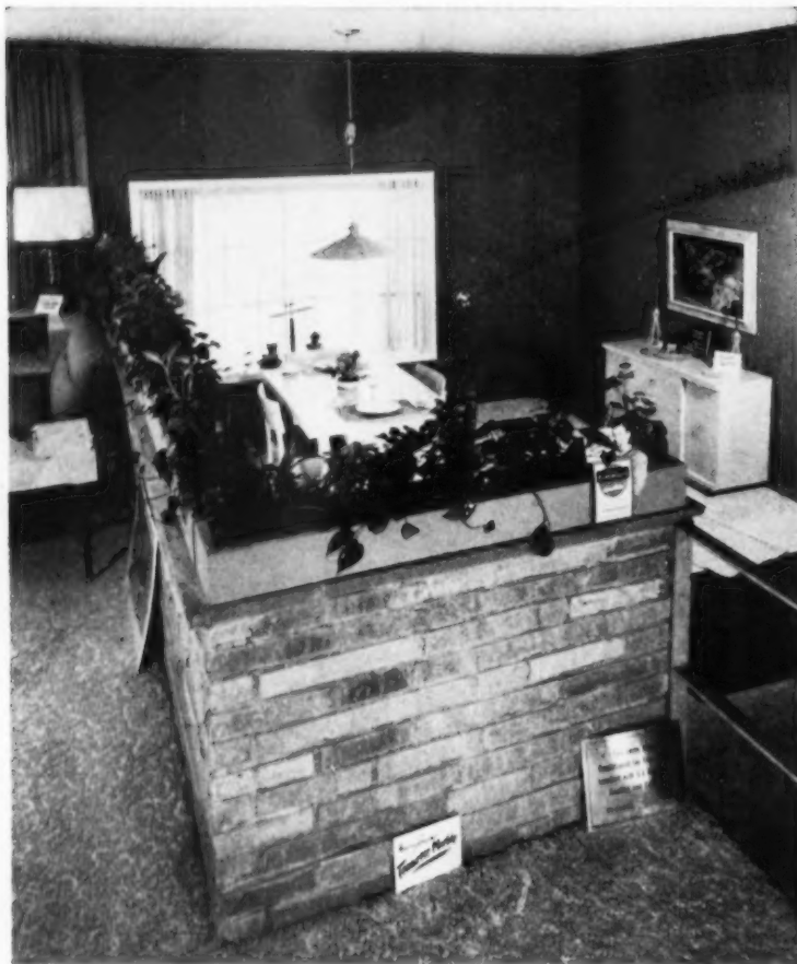
Veneered wall of Tennessee marble 30 inches high extends 17 feet along open side of living room. On dining room side, this wall is 54 inches high, faced with brick veneer. Ceiling area of living room, dining room and foyer is unbroken by partitions and is 10 feet above the lower level
