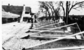
Roof view of skylights shows triangular prisms; 26-inch green glass clerestory (left)
