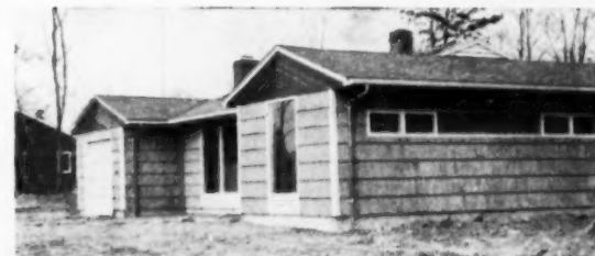
Roof lines of demonstration house indicate change of roof pitch and installation of gables instead of hips
