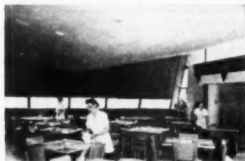
Ceiling, finished in vermiculite acoustical plaster, slopes from sides to center line
