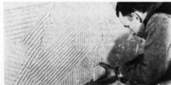
Applying the first tile . . . note the observance of the level line
