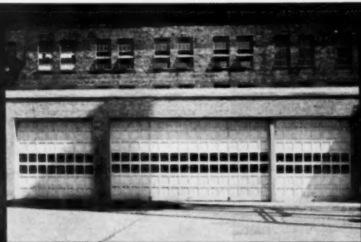
WIDE loading area is provided by these three Barcols at National Lock Company. Center door is 27' 9" wide and 14' high. Maintenance Foreman Tony Vincent says, "We have over 50 Barcol OVERdoors—some of them open and close over 250 times daily!"
