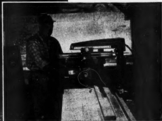
On-the-job sawing center builds profits for Metcalfe-Hamilton, Kansas City builders. Close up shows typical sawing shed at apartment house project. Delta radial saws, because they are more versatile, make more cuts, need less maintenance, are ideal for construction work.
