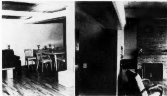
Two views of the Televue light trough built at ceiling level between living room and dining area. Ceiling is air-dried 2x6-inch t&g V-jointed fir car decking, also used for roof sheathing
