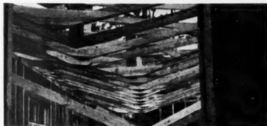
Trusses placed in position on walls ready to be nailed
