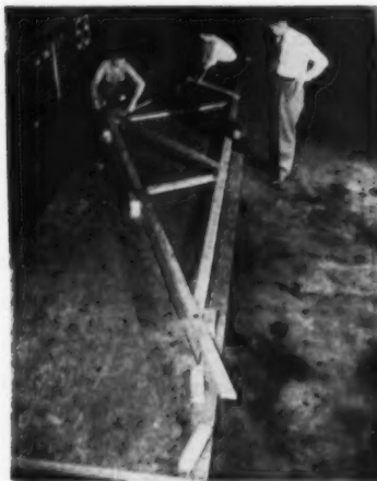
Construction of a "W" truss
