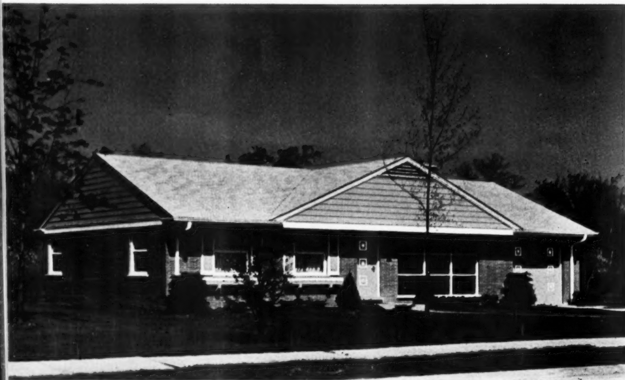
This typical mid-western ranch house, a favorite with builders, adapts itself well to any site
