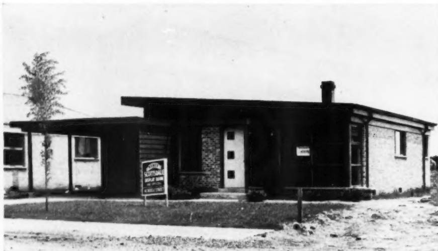
Combination flat-shed roof of this model, introduced to test the market, found a ready response in young homeseekers. They prefer it to the pitch roof models offered
