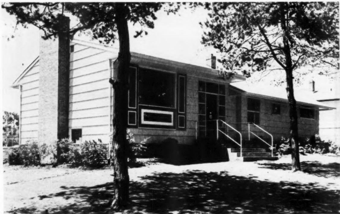
Reverse split-level design has a 26-foot through-the-house living room placed over the garage, four steps higher than other rooms. Heated air is exhausted from cooling tower through grille on lower side wall, partially obscured by shrubbery
