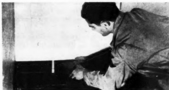
Applying the cove base after the entire wall has been tiled
