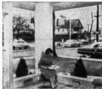
Expansive windows in reception room are set just high enough above floor to install diffuser grilles for supply ducts
