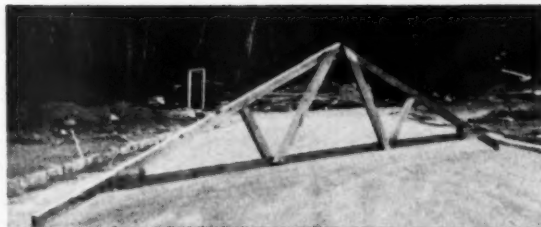
As each truss was completed it was stacked for future use
