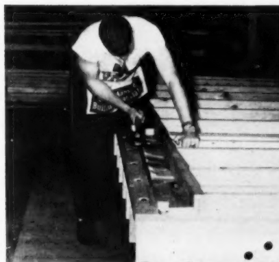
Face-nailing wall section on jig table
