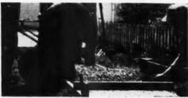
Concrete mix is placed between screeds. Strikeboard used for leveling the concrete
