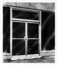
All exterior surfaces are polished and alumilited. The frames and doors are factory-assembled with concealed fastenings and factory machined joints.
