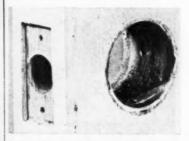
Door shows latch hole and lock hole with old lock removed, ready for replacement
