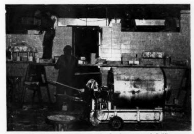
Silent Glow helped keep building warm for glazed masonry work. Building was heated to above 40 degrees
