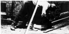
Tamping subgrade as d constructing forms enough to hold concrete in place asset preliminary steps in laying a driveway
