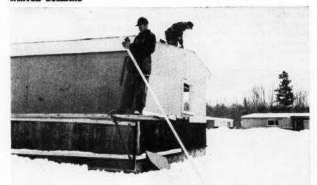
To protect structure from accumulated snow, architects specified this waterproof membrane be installed around perimeter of building
