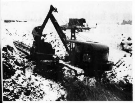
Excavations went on during the winter, Frost penetration was as deep as seven feet on unprotected land. Excavations went below frost line
