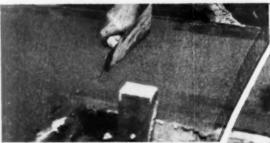
Trowel cut, about one third the depth of slab, is r rade at fivefoot intervals. Cut is then edged with a gro ying tool
