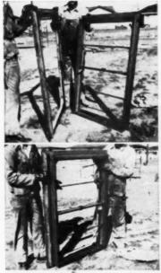
Windows are placed in wall and mix is poured around them. Photos show frame placed around window to get proper wall thickness
