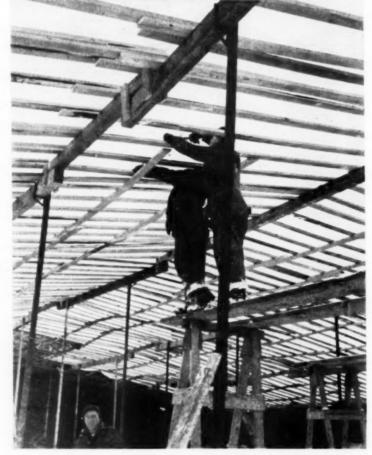
Shelters were built to protect concrete work. Tarps covered frame
