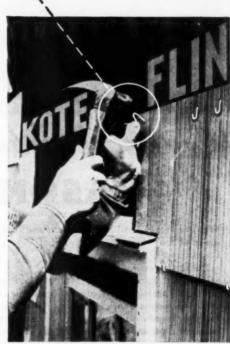
It's easy to get the knack of driving the Flintkote Hook-Nail. Application time is fast, good alignment is assured. And the siding really stays put. The siding will break before the Hook-Nail can be pulled out.
