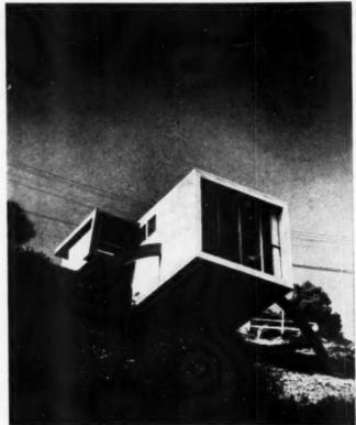
A laminated plywood arch with a span of almost 60 feet supports this living room as it projects out over a 45-degree grade
