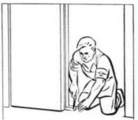
Open doors. Place floor guide halfway under doors, screw to floor. Move doors and secure other side. (55 sees)
