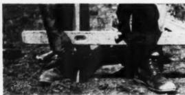
Setting stake for form in preparation for laying sidewalk. Grade of other form is established by means of a level
