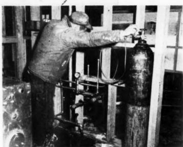
Nitrogen used to test service lines in place of water during winter. Tank had enough gas for four or five houses
