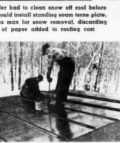
Standing seam was crimped to make it watertight and to hold it in position. Material had a base coat of paint
