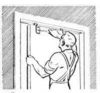
Bottom clearance should be 's". Loosen screw, raise or lower door, tighten. Insert other screw. (100 secs)
