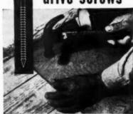
To make your linoleum underlays hold tightly and lie flat permanently, secure them with Hassall annular-threaded linoleum underlay drive screws. They are cement-coated for maximum gripping power. Heads are flat countersunk type. Size: 1¼" x #3 gauge. State quantity when writing for prices to:
