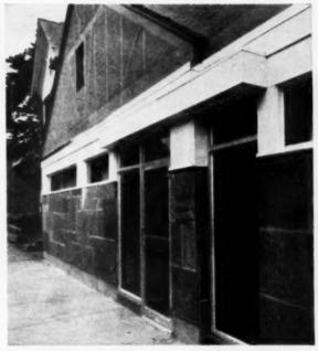
Detail view showing the application of the two-inch Bluestone and cement grout applied to the face of the masonry wall
