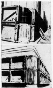
Corner has rolled steel form attached to the regular form. Three horizontal bars are placed below and four above the window
