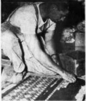
Making the ceramic tile facings for fireplace walls. (l. to r.) Each small tile is set by hand in small forms. Small sections are made into larger panels. Large panel is comented to brick fireplace wall
