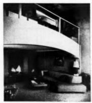
Balcony of second level extends out into living room. Metal rails extending up from arch have glass panels fitted into them to protect children from falling. Breakfast bar, above arch, can be hidden by folding screen
