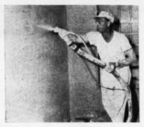
From the inside, two inches or more of perlite concrete are sprayed onto the lath in layers by the E.Z-On plastering machine. The paper-backed lath is torn off and an additional layer of perlite concrete is sprayed onto the exterior to form a reinforced concrete slab
