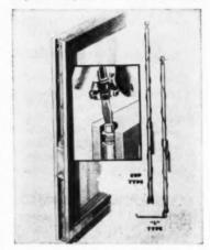
quality coiled spring contained in a dust proof, pre-lubricated tube is said to assure positive lifting power and true counter-balance. Turner & Seymour Mfg. Co., Hidalift Division, Dept. AB, Torrington, Conn.
