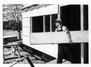
• The 2' x 8' size of this 25/32" asphalt-free sheathing is easily han-dled by one man. The V-groove feature cuts air leakage to minimum, assures the same high insulating value and sound-deadening qualities as in the larger sizes up to 8'x 12'. Completely weatherproof. Send coupon for full details
