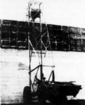
Special lifting device is attached to Ford tractor, lower section is used for house construction. Bucket holds 1/3 yard
