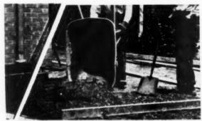
Cr.ncrete mix is poured and spaded against forms. Surface should be at least one inch above grade and pitched for drainage
