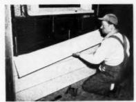
For a house job, aluminum siding applied with clips to studding serves both as wall finish and backing for sprayed-in-place wall
