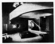
Cantilevered steps lead from entry at second level to living room and patio at bottom level. Floor at base of steps is 2-foot square concrete panels. The arch cuts into room, becoming a feature of the design
