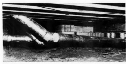
Ducts radiate from concrete block plenum placed under down flow furnace in crawl space
