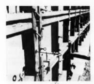
Forms are leveled by large I-bolt in foreground. On first form it screws down against footing to level. Only first set of forms needs leveling. Rod seen in middle of photo insures uniform thickness of form; is pulled while concrete is green
