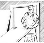
2 Use template to position carriers, attach with single screw. Mount guidestrip on bottom rear. (2 minutes)
