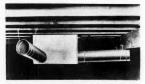
Metal plenum with connecting ducts is placed under down flow furnace in crawl space
