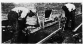
Excavating and placing of screeds for sidewalk
