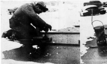
Lead vent flashing was prepared for soldering to terne metal
