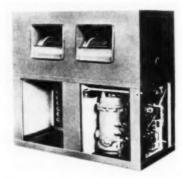
unit in which the refrigerating unit is located outside the home and the cooling coil is mounted in the main furnace air discharge duct. Both are produced in two- and three-horsepower sizes to cool average homes of up to eight rooms.
