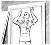
Mount track to header, keeping face of track flush with opening. (35
