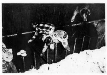
The concrete was screeded. Tarps were lowered and heat placed inside shelter during curing stage
