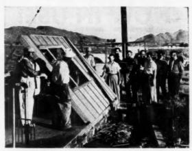
FIRST DAY—the job begins at 7 a.m. with 18 carpenters setting up wall sections on slab foundation
