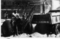
Efficient performance of the Sherman Power Digger is assured by positive hydraulic action and patented actuated bucket.
