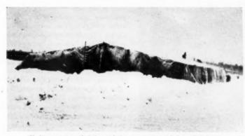
Shelters were needed if outside temperature was below 40 degrees. Temporary heating units insured proper curing of concrete
