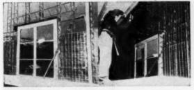
First a light steel frame of vertical wire trusses is erected. Paperbacked lath is wired on the outside of this frame. The procedure can be varied if conventional wood framing is used
