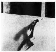
Better nailability. Fiberglas-reinforced gypsum board is less brittle, doesn't flake as readily during nailing. Nails hold better, too; reduces likelihood of unsightly pop-ups by nailheads. Installations look better . . . longer.
