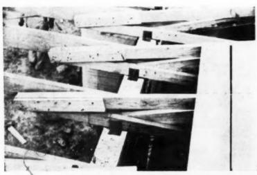
Roof trusses are bolted to the poured-in-place wall. Bolts are placed in position when concrete is poured
