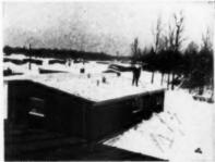
Roofer had to clean snow off roof before he could install standing seam terne plate. Extra man for snow removal, discarding
