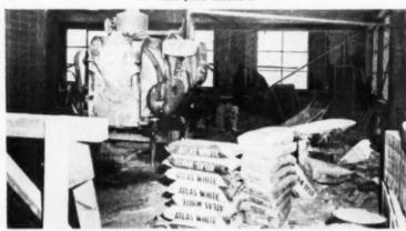
Mortar mixer was under cover in area warmed to 40 degrees to help batching
