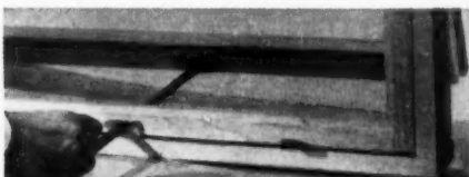
Window is opened by swinging bar-type sash operator to right angle with window and pushing sash out to desired distance.
