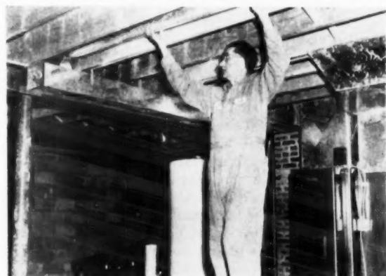
Making connection of small branch duct to main supply line
