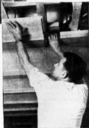
The extra-wide Lok-Bevel joint on tile and plank speeds application, hides staples or nails, and insures even, neat-looking joint lines.
