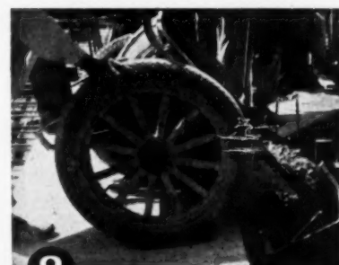
8 Use of rubber-tired buggies reduces chance of segregation. Spade or vibrate mix enough to settle and work it against forms.
