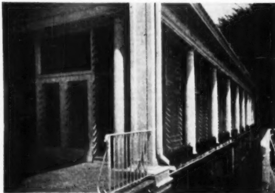
Two applications with extra-wide glass louvers. Slats in jalousies at left are 6 5/16 inches wide, enclose porch for restaurant at Wilmette Country Club, Wilmette, Illinois. Installation in southern Florida home has seven-inch louvers
