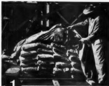
1 Always protect your portland cement from moisture. Store it on raised planks and keep well covered with a waterproof tarpaulin.
