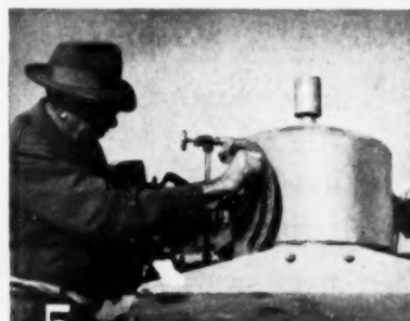
5 According to the conditions to which the concrete will be exposed and the strength desired, set mixer gauge for needed water.
