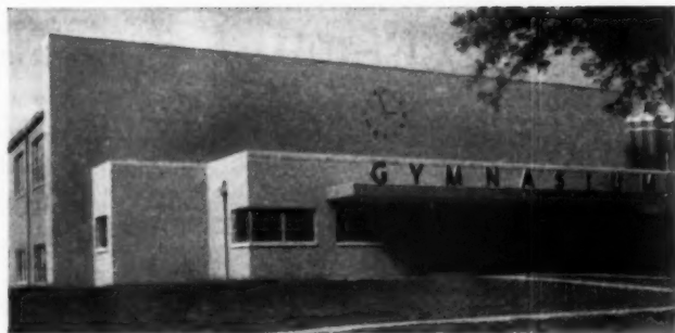
Green Valley School Architect— GEORGE POPPO WERDA , Pekin, Illinois Contractor— C. IBER & SONS, INC. , Peoria, Illinois Dealer— SCHUREMAN HARDWARE & LUMBER COMPANY , Green Valley, Illinois
