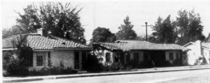
Left, a 2-bedroom house. Entrance shown leads to second bedroom, front entrance faces avenue. To right is a triplex comprised of three separate apartments. End units have single bedrooms; center unit has large living room, kitchen-dinette, and bath
