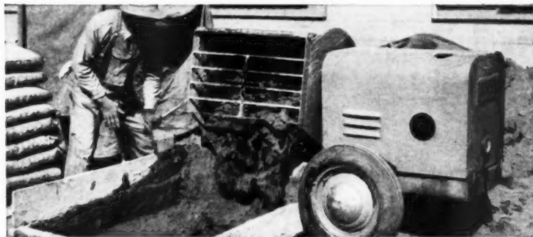
Jaeger Multi-Blade 3 1/2 Ft. Power Hoe — the heavy duty small mortar mixer. 6 1/2 ft. size for larger jobs.
