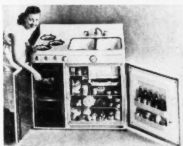
AB14081—PACKAGE KITCHEN —General Air Conditioning Corp., Dept. AB, 4542 E. Dunham St., Los Angeles 23, Calif. A large oven has been added to this unit, which includes double sink, gas or electric burners, six cubic-foot refrigerator, double bottle shelf. The new oven includes a broiler. The refrigerator has a freezer which holds 12 frozen food cartons or nine ice cube trays. This unit was designed for use where space and dollar economy are important; occupies 42 inches of wall space.
