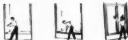
1. Screw side jambs to the walls. 2. Secure bottom rail to the tub with mastic. 3. Slide doors into top rail and slide into position.
