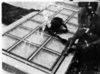
Oakum is forced into expansion space between curb and panel
