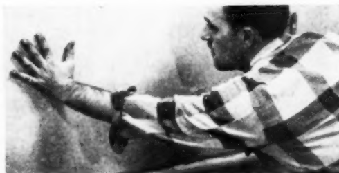
Place bottom glass panel against back wall (resting on cardboard tabs) and apply pressure against glass to give proper adhesion between glass and wall
