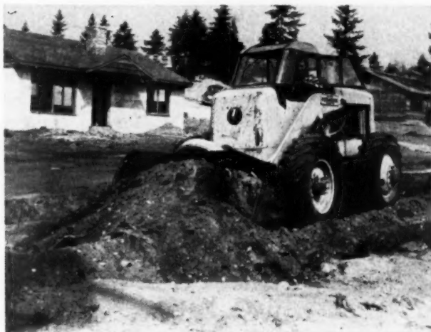
PAYLOADER: moves dirt and gravel on the site by loading truck; also does rough street grading, rough land clearing and brush clearing. Indispensable for work on rugged terrain
