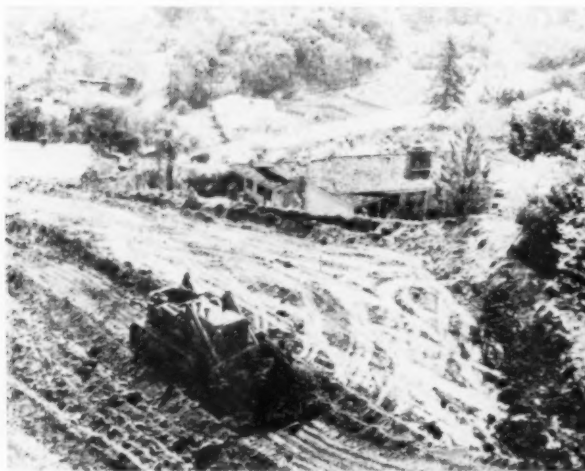
BULLDOZERS, BIG AND LITTLE: Diesel-powered crawler tractors compact the earth of a given site to specifications. The small machines do the work of close grading near houses, spread gravel preparatory to pouring slab floors. The machine also back fills and pulls utility trailers
