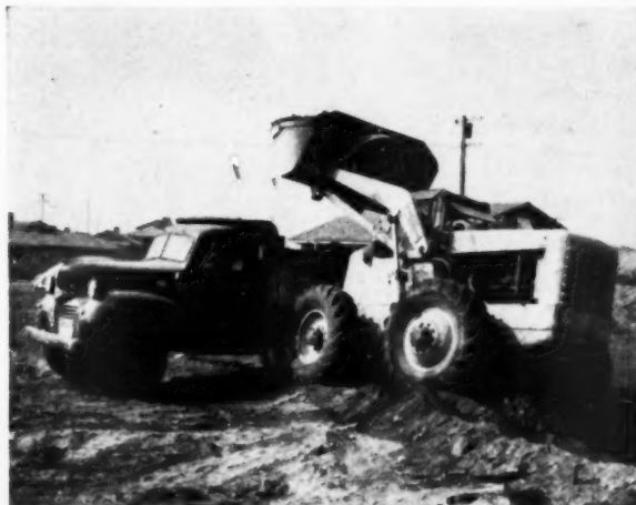
PAYLOADER: moves dirt and gravel on the site by loading truck; also does rough street grading, rough land clearing and brush clearing. Indispensable for work on rugged terrain
