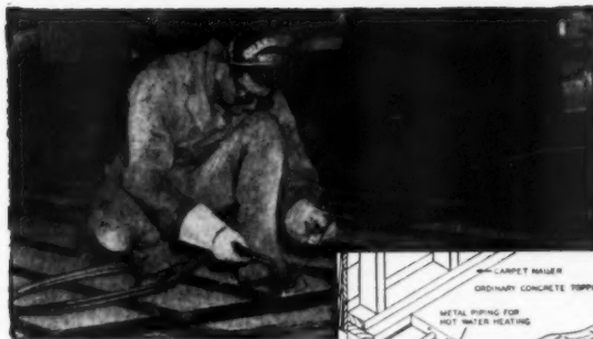
Under radiant heat pipes for more efficient operation and control.
