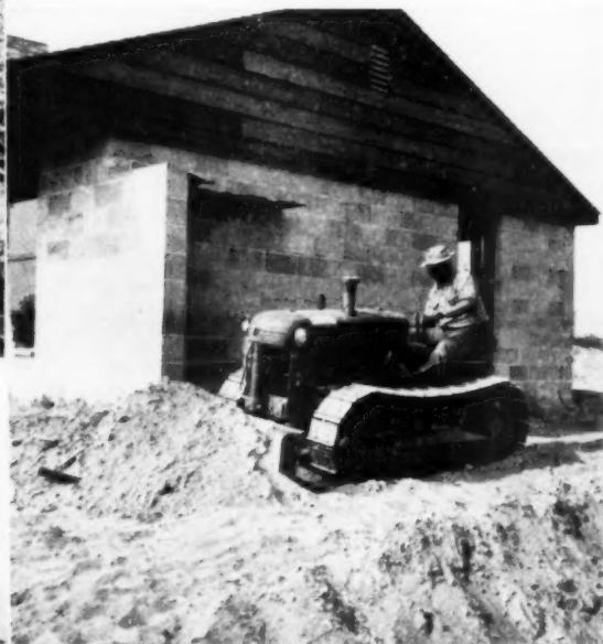
BULLDOZERS, BIG AND LITTLE: Diesel-powered crawler tractors compact the earth of a given site to specifications. The small machines do the work of close grading near houses, spread gravel preparatory to pouring slab floors. The machine also back fills and pulls utility trailers
