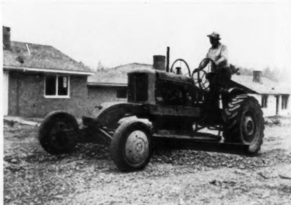
ROAD GRADER: finishes the job of bringing streets to final grade
