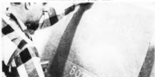
Reverse cardboard and mark "tub side" and "bottom side" on cardboard for reference
