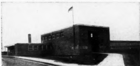
First building to incorporate Toplite panels is the W. K. Kellogg School Addition in Middleville, Michigan—14,600 square feet at a cost of $13.25 per square foot
