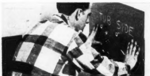
Place template over fittings to check hole alignment
