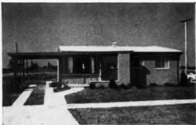
Front of house showing the tie-in arrangement of entrance and carport
