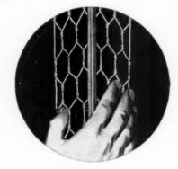
**Keybead** combines open-mesh reinforcing lath with a precision-formed galvanized steel bead. It assures a solid plaster corner, reinforced with a network of galvanized wire that is strong and prevents rust streaks.
