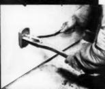
Insert cutter—SQUEEZE HANDLES TOGETHER
