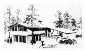
This split-level house takes full advantage of a sloping lot, featuring a patio on the lower grade, front entrance at the intermediate level, and a kitchen "housewife supervisory" area on the top level. Structural steel frame of basic house is exposed along side walls
