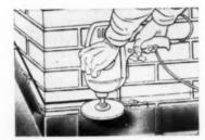
Using grinding wheel, roofer cuts a ½-inch groove, 4½ inches above roof line
