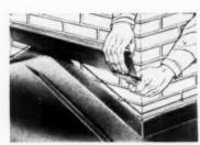
Cap flashing is cut and bent all around chimney to fit into the groove in masonry
