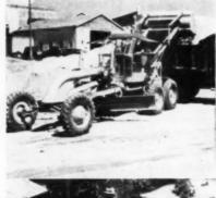
LOADS OR TRANSPORTS sand, gravel, cement, other bulk materials with ½ yd, rear-mounted hydraulic bucket. Dumping height of 8 ft., 8½ in, allows easy loading of high truck bodies.
