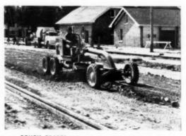
ROUGH GRADES for curbs, gutters; finish grades shoulders, sidewalks, between forms; cuts and cleans drainage ditches; removes weeds and brush.
