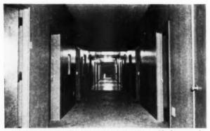
FLOOR TO CEILING INSTALLATION OF BOLTA-WALL provides beauty and protection in busy corridors and rooms at Seton Hospital. Note that Bolta-Wall is applied first; floor and rubber cove base are installed later.
