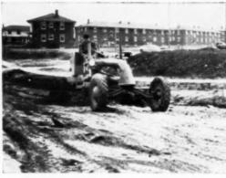
BUILDS AND MAINTAINS roads, streets, alleys, driveways; spreads rock; scarifies; cleans up on construction work. Excavates shallow for slab foundations
