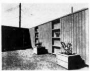
Fence combines panels of both wide and narrow grooved fir plywood, applied to redwood frames
