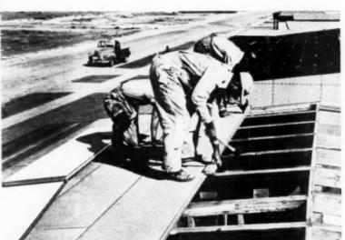
Particularly adaptable to flat or low-pitch roofs, this roof deck material can be applied quickly. Three men shown in the photograph applied 1.000 square feet in two hours
