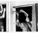
**Step 2.** Screw in jamb clips, attach jamb post to them. No planing or fitting necessary. **Step 3.** Job is done! No hardware to install. No painting or finishing required.
