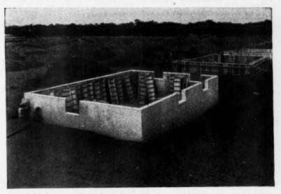
First of foundations put in by Centex Construction Company of Dallas, Texas, General Contractors for the Waukegan Home Project. Note Symons Forms and the minimum walling and bracing required.
