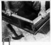
Inter-Lok frames for 13/4" are shipped knocked-down. Frame locks together to form neat, mitered corners. Designed for use with Amweld 1 % " Flush Doors, these frames can also be used with wood doors. Available in all standard sizes to match Amweld Flush Doors. Can be furnished as assembled unit if required.
