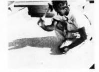
Large-headed galvanized nails. long enough to penetrate the framing members at least 1<sup>1</sup>2-inch. are used to apply the 2x8-loot roof deck sheets
