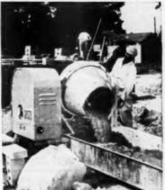
Jaeger 31/25 tilter has double-action "V" bottom drum Famous Jaeger-patented drum design doubles the mixing action of any ordinary tilter; also produces cleaner discharge of concrete, mortar or plaster.
