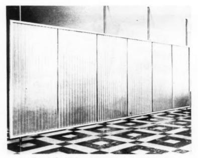
Mounted "Sturdalite" panel, showing use of manufacturer's Seal Strip, which joins butting sheets of panel, avoids lapping
