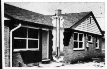
SECTIONAL CONSTRUCTION saves 30% to 50% on time and material over brick chimney cost. The Van-Packer may be placed directly over furnace in center of house as easily and inexpensively as against a wall.
