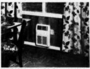
DINING ROOM, showing SelecTemp unit which has 12,000 Btu per hour maximum output capacity.
