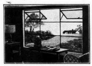
Lok'd Bar Joints at muntin intersections. Ventilator corners are solid-welded. Ventilation is 100% flexible. Awning type ventilators may be inserted in frames where desired. Any type of glazing may be used: Thermopane, Twindow, or single double-strength glass.
