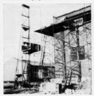
Self-raising "Hoister" tower handles loads to 2000 lbs. Available with either material cage or 14 ft. concrete bucket, and in 10' sections up to 67 ft. high. Up to 37 ft. heights it is selfraising. Moves around job on its own skil base. Automatic safety device positively pre-
