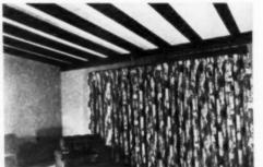
The living room ceiling in this home is the finished surface of the underside of the roof panels. These panels combine three functions in one—roof decking, roof insulation, and a prefinished interior ceiling
