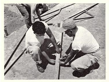
(A) To assemble steel truss, workers in foreground bolt intermediate struts to top chord. Man in rear folds one-piece strut to W-shape for next truss
