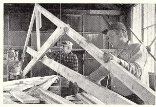
(H) Workmen lift scissors truss from jig. Builders fabricate truss on project site under cover of old hangars which builders inherited with purchase of land they are developing, deliver trusses to house by truck
