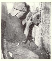
The saw can be used to cut openings in concrete walls by scoring walls to maximum depth along dimension lines and then breaking concrete between cuts. Diamond grit blade is used on hard concrete with water feed attachment. Flex or cut-off wheel is suitable for soft concrete
