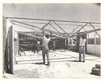
(D) Trusses are hung upside down on exterior walls, then turned upright into position. A sheet-metal bird stop is shaped to fit between trusses, automatically spaces them 24 inches on center
