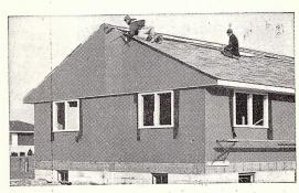
There's virtually no waste with Upson All Weather Sheathing. Small pieces from window cut-outs used to finish gable.
