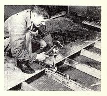
squeezes the boards tightly together and holds them in position, leaving hands free for nailing.
