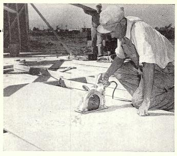
Celotex or similar wallboard or sheathing products are cut best with a fine tooth blade. Carbide tipped blade should be used on asphalt coated material. Support firmly while cutting
