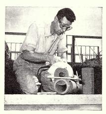
The abrasive flex cut-off wheel also makes short work of concrete septic tank pipe. Diamond grit is recommended for hard concrete, using water feed attachment to keep down dust
