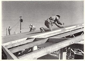
(E) Sheets of 4x8-foot, %-inch plywood can be nailed directly to steel trusses with screw nails. Roofing felt is fastened to plywood with tin discs and a stapling machine
