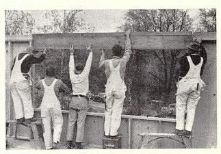
Special header over picture window goes into position. . . .
