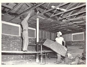
(F) Insulation batts are installed on wires strung from trusses. Blown insulation may be put in after ceiling material is applied. Electrical outlets may be fastened directly to trusses or blocking
