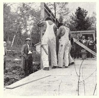
Carpenters tip panels into position. Nail bottom plate to sill and panels to one another through butting studs. . . . .
