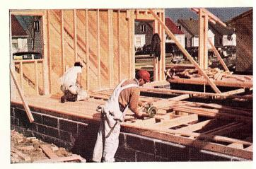
Tilt-up method is used to erect Studio House. Five to six weeks is total construction time per house
