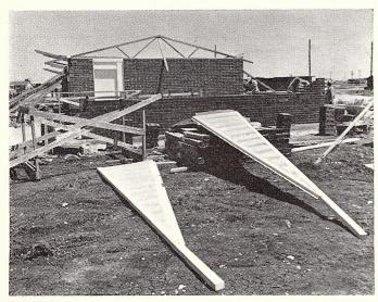
(C) First truss is in position. Taut string from gable at one end to first truss at other end aligns the trusses. Steel ventilating gable end is built in two sections, will be erected upon completion of its bearing wall
