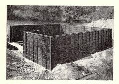
handle, easy to set-up, easy to strip. The width of the steel frame is only  $2\frac{1}{2}$ " wide compared to  $4\frac{3}{8}$ " for wood frame forms. The forms are so constructed that, when necessary, panels can be easily replaced right on the job.
