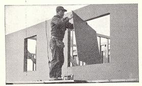
Only Upson offers king size sections. Work time cut 50%. Windows cut out after application, pieces used in gables.
