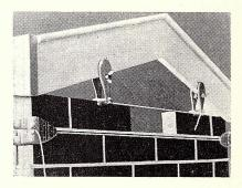
face-board. Moving from one row to another is simply a matter of sliding the fastener up the face and re-tightening the thumbscrew. The line is fastened by a pull of the cord into a vee, which wedges the line firmly into place.
