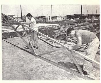
(B) Bottom chord, with its wood filler strip, necessary to attach ceiling, is bolted to struts. At rear, assembled trusses are stacked ready for erection
