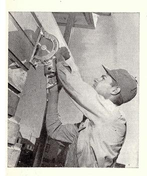
Builder saws are offered in three sizes—6-inch, 7½-inch and 8½-inch. Portable power saws reduce wood cutting operations from hours to minutes. The carpenter here is trimming wood siding
