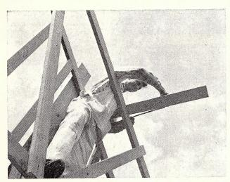
Carpenter spaces trusses as they are lifted into position . . .
