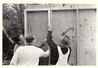
Panels are nailed through butting 2x4 studs. Note two foot panel on the left. . . . .
