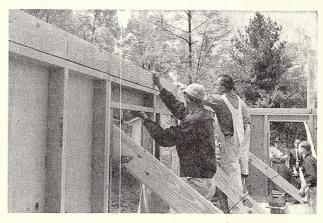
Building has continuous double 2x6 header which is nailed and lag screwed to the top 2x4 plate of the panel....
