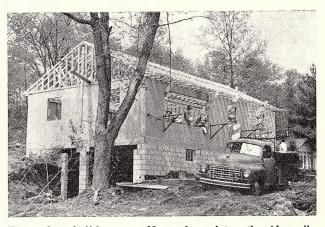
Five and one-half hours—or 22 man hours later—the side walls, trusses, and some of the roof sheathing are in position. It was conceded that builder could have made better time without interruptions and interference
