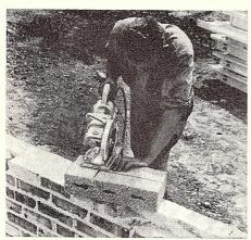
Concrete or cinder block is also cut with abrasive disc. Block can be scored on both sides to assure cleaner break
