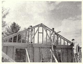
Gable end truss and one standard truss are in position. . . .
