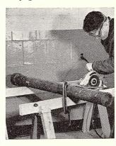
Cast iron soil pipe is cut with abrasive flex wheel. Saw is fed slowly but firmly into cut, turning pipe as necessary
