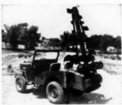
gear driven trencher has hydraulic boom drive
