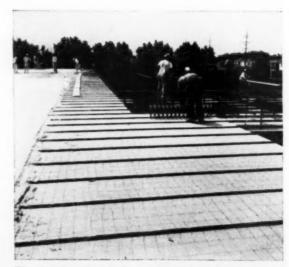
The formboard and the welded wire mesh are placed before pouring of the Pyrofill gypsum concrete
