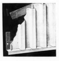
prefab gable end provides baffle-type venting
