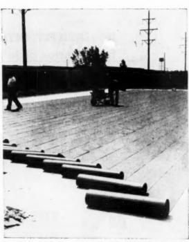
Pyrofill roof decks attain high initial strength within the hour that they are poured. Roofing can be applied immediately
