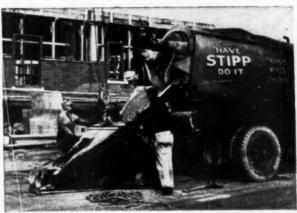
POURING TRANSIT-MIXED DURAPLASTIC concrete for Bell Telephone Dial Exchange in Olyphant, Pa. General Contractor: R. D. Richardson Constr. Co.: Ready-Mixed Concrete: Exra Stipp Constr. Co., Scranton, Pa.
