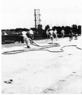
The pump and hose method assures quick pouring of the entire deck area. The slab can be walked on 15 minutes after pouring
