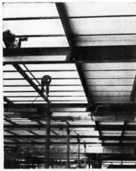
The interior of the job is kept clear of shoring. Erection is fast, and other trades are always free to proceed with their work
