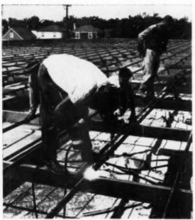
Sub-purlins are spaced accurately to hold the gypsum formboard. These are welded on alternate sides of each purlin crossing
