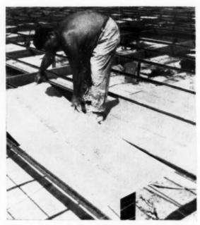
Gypsum formboard,  $\frac{1}{2}$ -inch thick and 32 inches wide, is placed so that the end joints fall directly over the purlins
