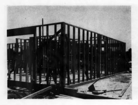
THE CHALLENGER uses conventional 16inch o.e. framing, roof trusses. Labor cost is about the same as for The Westerner
