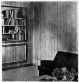
V-PLANK ADDS a note of textured wall interest that says good taste in any price home. Shadow line of grooves adds to apparent height of room.
