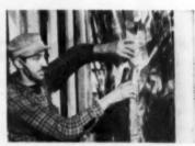
In extra-wide stud spaces where the panels of accordion insulation must be joined together to close up a space, a stapling plier is used for fastening the flange surfaces together
