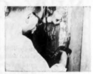
spring-driven stapling tacker is used to fasten accordion aluminum insulation to wood studs where there in not much more than several inches of space in between the studs to be covered
