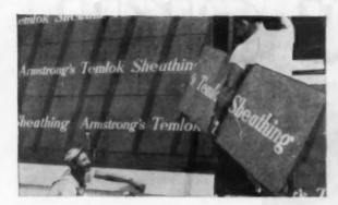
No building paper needed. Because Temlok is completely waterproofed, shingles, clapboard, brick, or stone can be applied directly to it without building paper. Once the house is finished, Temlok prevents dampness from seeping in through the walls, yet allows vapor to pass out through the walls. This prevents condensation from collecting inside and causing damage to the structural members.
