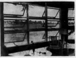
INSIDE—Equally pleasing. New-type Curtis operator provides controlled ventilation yet locks sash securely.
