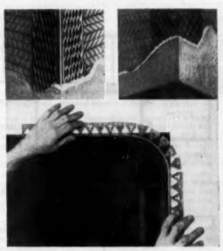
TRUSCON MSTAL LATH protects against cracks. Truscon manufactures more than 40 different metal lath items, corner beads and accessories. They are approved by all building codes, and accepted by plastering contractors. See that metal lath and accessories protect corners, edges, arches, window openings, door openings and other vulnerable spots in your homes. Stocked by building materials dealers, backed by Truscon's nation-wide warehouse service.
