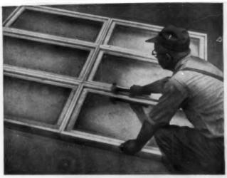
In building up this Flexivent group, workman makes sure that units are kept square and properly aligned...an important step. "It's Flexivent's ready application to all types of construction that makes it a favorite with project builders," says Mr. Musgjerd.
