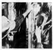
Here is a stapling hammer being used to secure multiple accordian insulation to wood studs. Space between studs allows enough room for hammering movement with this stapler
