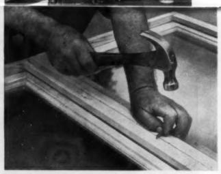
In this close-up a shop workman places Flexivents in position for joining. Joining with corrugated fasteners is best method. "With Flexivents," reports Mr. Musgjerd, "we find we can offer customers a wide choice without carrying a large inventory."
