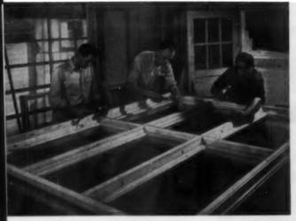
Workmen assemble group of Flexivents in shop at the Richfield Lumber Company, Richfield, Minnesota. "Ease of assembly with Flexivent units means we can produce more units with our regular staff of workmen," says Allan Musgjerd, Manager.
