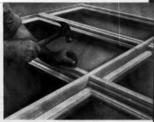
Finishing up the assembly, workman here applies outside casings, subsills and batten strips. The built-up Flexivent groups are trucked to the job all ready for installation. "No unit tops Flexivent," states Mr. Musgjerd, "for combining high quality and low cost."
