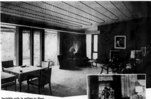
Invisible coils in ceiling or floor.
