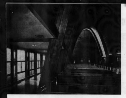
Parabolic in shape, luce, laminated rafters form the skeleton and shape of interior. Iwo-inch depression in brick wan over altar is to receive future ceramic mosaic
