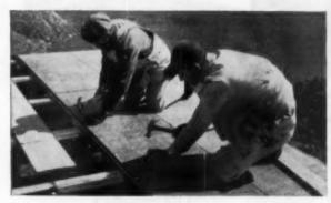
No additional insulation is needed. No matter whether you're building in a warm or a cold climate, Temlok Roof Deck provides adequate ceiling insulation. You're spared the expense and trouble of installing insulation separately. For use in areas where the average January temperature is 40° F. or lower, Temlok Roof Deck is available with a special vapor barrier for protection against moisture.
