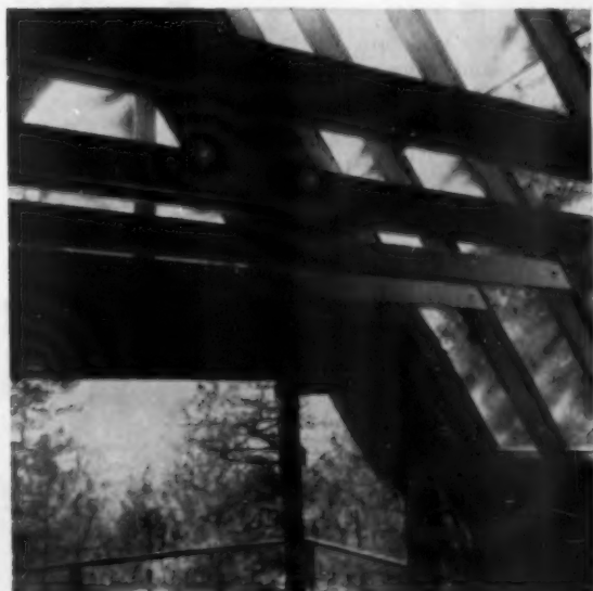
Fixed plate glass placed in steps between rafters' open living room to trees and sky
