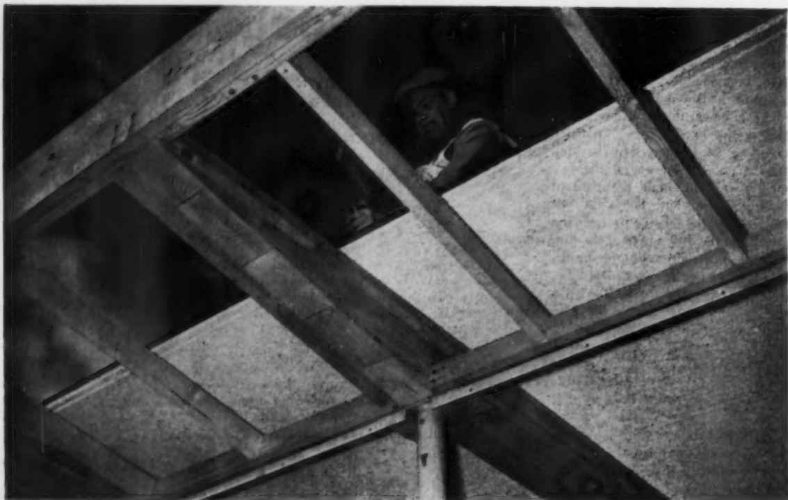
Lightweight roof plank is laid with the long dimension at right angles to the supporting members, and nailed at each crossing of the plank over the frame
