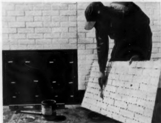
Holl-E-Wood brick can be fastened to surface with mastic cement, as shown here being applied to hardboard, or by nailing
