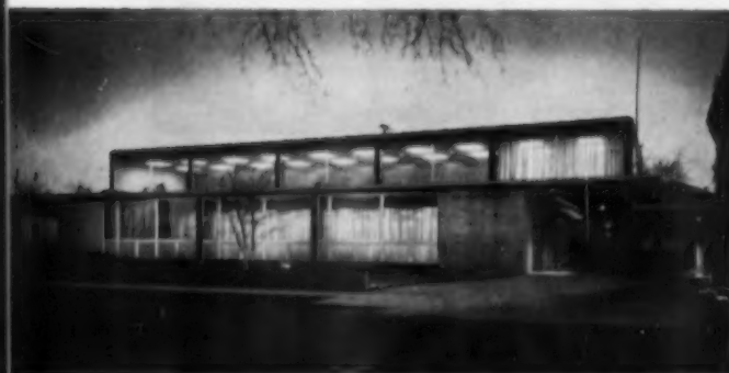
CONCRETE SLAB AND PIER construction is freely revealed. Polished stone veneer facing and aluminum coping make effective trim
