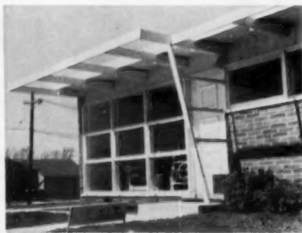
Detail of the front. Note the method of securing outrigger to the extended rafter ends. Designer was Harry J. Quinn, architect
