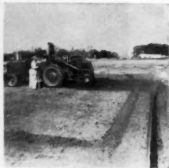
Ditcher is completing the third wall of the four-sided cut
