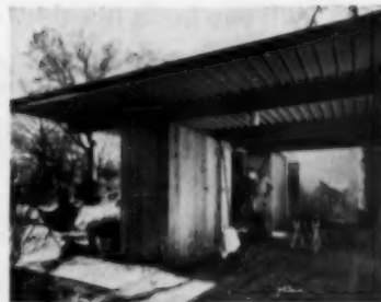
ROOF FOR CARPORT. Not shown on roof framing plan (left), the carport is roofed with a lightweight steel decking supported on cantilevered "I" beams. Less expensive than conventional decking, the material comes in sections 18 inches wide and up to 25 feet long. It is used plain here
