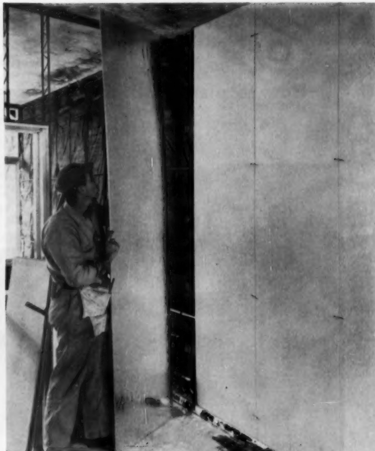
PLASTER BASE is foil-backed Rocklath in 9-foot lengths. Blanket insulation is used between the studs
