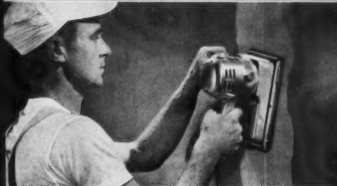
Black & Decker 88 Sander sands joint seams in dry-wall construction satin-smooth in a fraction of the time of old-fashioned hand sanding.
