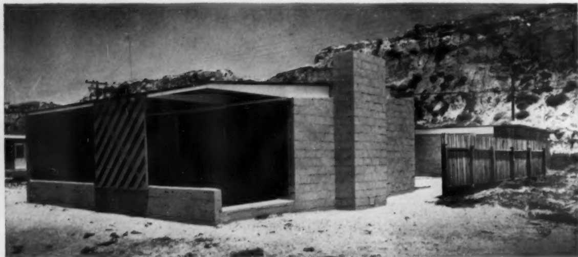
Exterior is faced with a combination of vertical wood siding and concrete blocks left exposed on the interior. Roof is flat except over living zone, where it is pitched slightly
