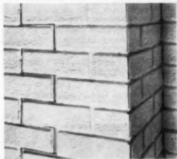
Corners are formed by mortising edge at 45 degrees, so two edges meet to form 90-degree corner cut on straight line. In nailing, drive nails through mortar joints. Use small flat-headed nails or brads
