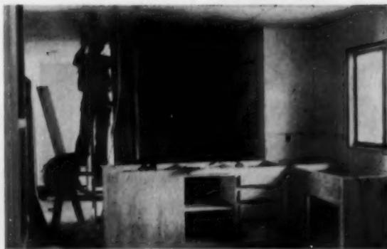
All gypsum wallboard panels for the finished ceilings and walls are nailed in place before storage walls and cabinets are set in place
