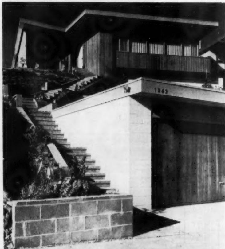
**TO GAIN GROUND** toward the rear without resorting to fill, a portion of the front of the house was cantilevered out from the foundation wall. This adds to appearance without increasing cost. Architect was Morris D. Verger of Los Angeles
