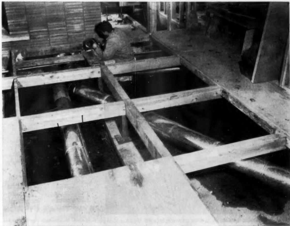
WIDE-SPAN JOISTS AND 1-INCH PLYWOOD SUBFLOOR save time for subs, money for the builder
