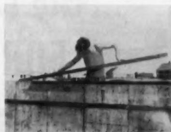
Line-up rails slip into place, eliminating line-up braces, providing positive alignment of forms
