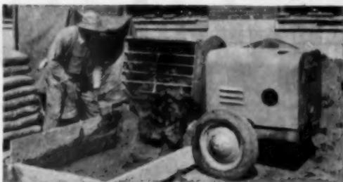
Pugmill type mortar mixers—Jaeger 4-blade Power Hoos give you fast pugmill criss-cross mixing action. Turn out smooth, uniform, even-tempered mortar that's easy and fast to spread. 3½ and 6½ ft. sizes to keep ahead of any size crew.
