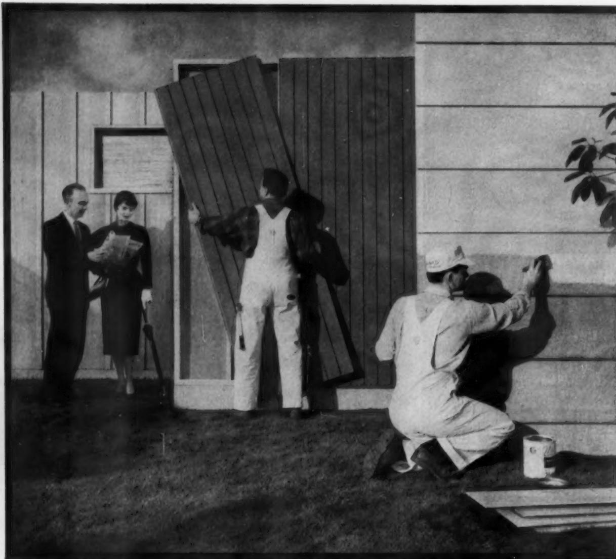
SHOWN ABOVE—(left to right): Rough sawn hemlock board and batten; Tree Life Texture One-Eleven (4" groove spacing); PlyAloy Overlaid Siding.
