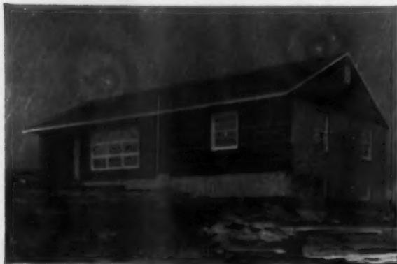
**Rain-Shield® finish guards against moisture damage** Even several days of rain can't damage Temlok Sheathing exposed on the studs. The Rain-Shield finish waterproofs every square inch of Temlok's surface, while asphalt impregnation of each fiber insures moisture protection clear through the board. Carpenters can resume work almost immediately after rain has stopped.
