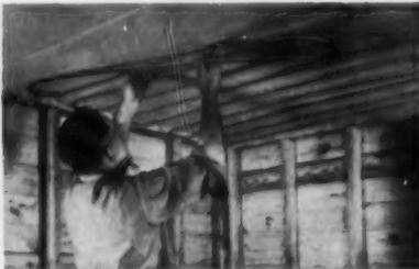
**A HOOK TYPE FASTENER** offers another easy, quick installation method. Fasteners are partially set in joists, PG's are positioned, and fasteners driven home.
