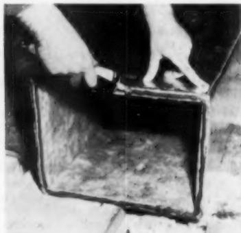
After duct has been cut, sealer is applied to butt ends, in much the same manner as calking compound
