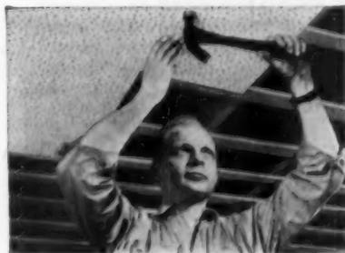
QUICK, EASY TO INSTALL. All you do is nail 1" x 3" furring to joists, then nail Cushiontone to furring, and the ceiling is completed. No special skill or tools are needed. In one simple installation, Cushiontone gives you sound conditioning, beauty, and a finished ceiling.
