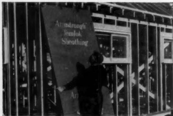
**Eliminates corner bracing** Temlok Sheathing has triangular bracing built right into it. Because of its large size and exceptional strength, corner bracing can be completely eliminated when you build with 4' x 8' x 2 1/2" Temlok Sheathing. This size board provides over four times the building strength of horizontal wood sheathing. When you build with Armstrong Temlok, you know you're using a material that exceeds all Federal Specification strength standards for insulating fiberboard.
