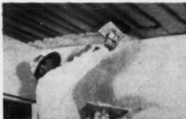
**NO SAGS OR DIPS** in the tube lines permits a uniform plaster thickness, which means savings in time and materials.
