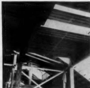
**A SHED-TYPE STRUCTURE**, 50 by 60 feet, with columns 20 feet apart, uses clay tile decking and clay tile girder that spans 50 feet. The prefabricated members were set in place in half a day
