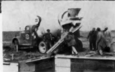
Gates Engineering Department designed one set of Horizontal Rod Panel Forms that could be used for all four plan variations in this development. They were manufactured of plastic-surfaced plywood in 32" widths—for maximum speed in erection and stripping. Delivered to the job at noon one day, the forms were set up, ready for pour, by 9:30 the next morning.
