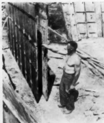
As forms go up, tie rods are slipped into position, secured into place with Simplex Locking Levers, remain in finished wall. No walers are required
