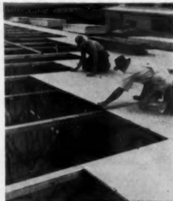
**$\frac{3}{4}$ -INCH PLYWOOD DECKING** goes over 4-foot spans and is nailed to 4x4 nailers secured to tops of the joists
