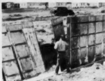
Forms are placed in approximate location when unloaded (left). Then starting at one corner, forms are put up in counterclockwise direction. Inner and outer forms are erected simultaneously
