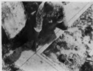
Foreman makes layout on footing. Each form touches footing, anchoring itself, overcoming unevenness of footing. Most hardware is mounted on forms, cannot be lost, eliminates "pick-up" operation
