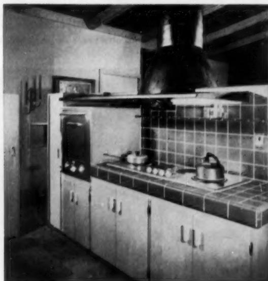
**BUILT-IN KITCHEN** units are placed against 5 foot-high fireplace wall that screens cooking activities from living room. Fan in hood over range is vented by 6-inch flue running inside 24-inch chimney pipe
