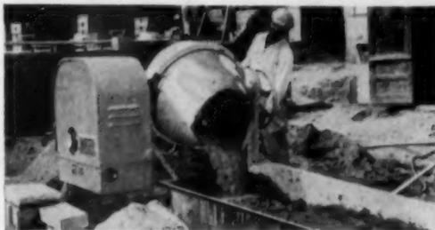
Mix better, pour faster—Jaeger 3 1/8 Tilter drum has patented "dual mix" V-bottom that gives double the mixing action of ordinary tilters and also speeds discharge. Produces big daily yardage of high strength, high quality concrete or mortar. Tows fast, spots fast.
