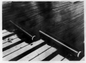
Koroseal vapor barrier being applied over Fenestra acoustical panels with Lexsuco fire-proof adhesive
