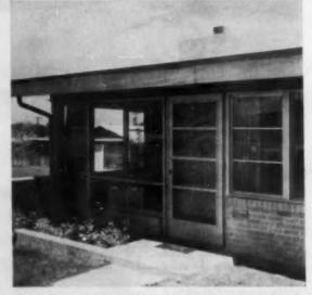
A simple screen door design with a minimum width for rails and stilles. This screen door is particularly effective when used in conjunction with a slab type of exterior door. The drawing of door frame and adjoining window on opposite page is applicable to this installation
