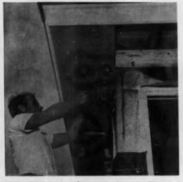
FIRST STIP in eave plastering, after installing 2x6 ribbons, blocking and vents (Fig. 2, upper right), is to apply rocklath. Knuckle-bustin' job of notching lath around rafters in open-end eaves is eliminated.
