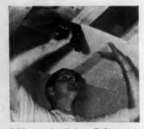
Quick, easy installation. Cushiontone is a complete ceiling in itself . . . goes up fast without special tools or training. It's quicker and less fussy than plastering or drywall. Cushiontone can be stapled, nailed, or cemented. No finishing is required.
