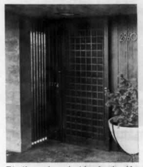
This grid-patterned screen door is hung from the end face of the door frame. The frame can be built of 2x6 or 2x8 inch members, depending upon the adjoining materials
