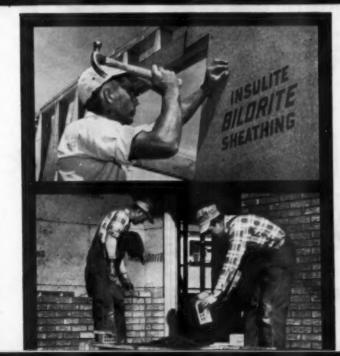
Bildrite goes up faster, easier. One carpenter can sheath 1,000 square feet in 6 hours or less with Bildrite. Cuts application time as much as 43% compared with wood. Adds strength. 4' Bildrite has more than twice the bracing strength of horizontal wood sheathing, thus eliminates corner-bracing. Waterproofed throughout with asphalt. No need for building paper. Can be used or stored anywhere in any weather.
