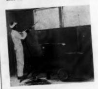
Plastering machine has instantaneous control at gun head
