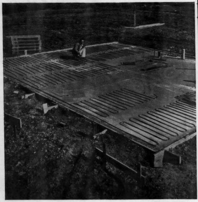
IN THREE HOURS, this crew has the floor radiant panel heating system 75 per cent completed, thanks to AnacondA Pre-Formed Panel Grids.
