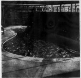
The entire rear yard with the swimming pool is covered with plastic screen that allows bathers to get sun tan but keeps out insects and cold. Pool shapes are different, conform to the individual lot size and shape
