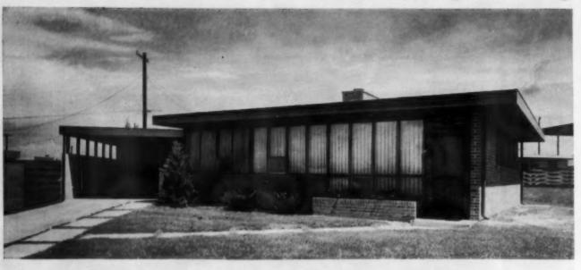
\$14,000 Brick cavity walls with a combination of face brick and plywood for the interior finish
