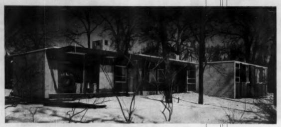
FIRM GRIP of midwestern winter holds no fears for Wessel household. Roof, walls and slab are insulated with fibre-glass. Window wall has insulating glass.
