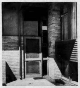
An effective design of screen door, sidelights and transom for a split-level house, with a minimum width required for mullion and transom. The drawing of door frame and adjoining window, left, shows how the door extends across the face of the frame. This can be easily changed to conform to the photo where a  $1\frac{2}{3}$ -inch rabbet is provided in the frame
