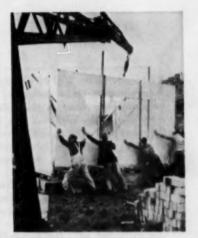
Wall is lifted by crane for placement on hardwood floor joists
