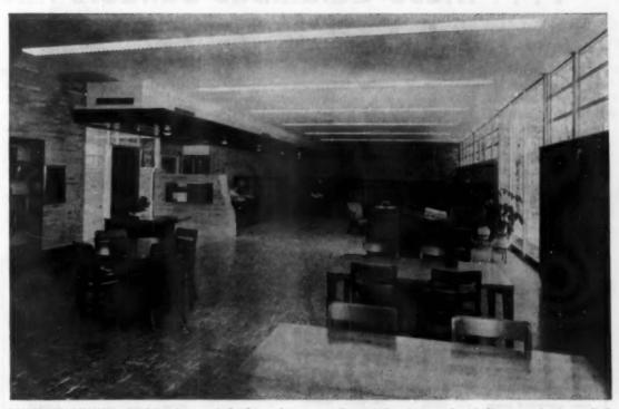
SOUND CONDITIONED CEILING of acoustical plaster has fluorescent fixtures to supplement north daylight, Floor-toceiling window is framed with Kawneer aluminum, Redwood of canopy is repeated in librarian's desk below.
