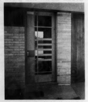
A change of pace is indicated in the width of the rails and stiles of this door. The center cross members protect the screen wire while adding design value to the door. The frame as detailed in the adjoining drawings can be used for a brick veneer or cavity brick wall
