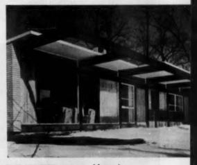
**POST AND BEAM** structure of house is emphasized on exterior. Cantilevered 5 feet past posts, black-painted beams have 42-foot fascia to form overhang.
