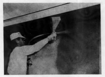
FINAL STEP in eave plastering is to shoot eave and sidewall with stucco in continuous operation. Operator works off platform, gives first coat light wettings before browning. Stucco is dumped in funnel at top.
