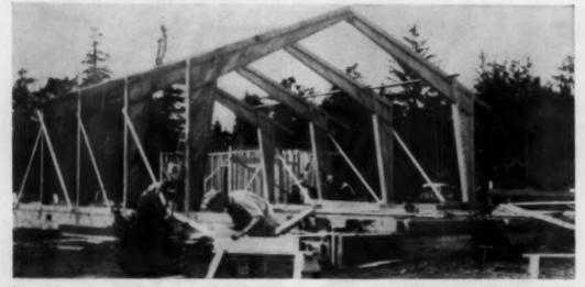
Beams shown here are being erected for a building at a Boy Scout camp, have 36-foot 8-inch span and are placed 14 feet on centers. Drawings detail this type of HB beam. HB beams can take many forms
