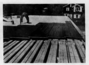
Fibrebourd insulation is placed over Koroseal after a mopping of Lexsuco adhesive
