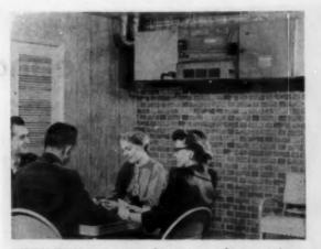
OFF-THE-FLOOR can menn playroom, crawl-space, attic, or utility room installation for the Coleman Blend-Air horizontal furnace. Burner and controls are shown in left section, but are convertible to right hand placement.
