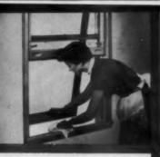
Cleaning and painting is a cinch. The entire window unit swings out for easy sill cleaning. Or you can lift unit off entirely for painting.
