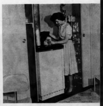
**INCINERATOR**, Brule Model M-1, is at exterior wall side of service lounge and has its own vent through an annular flue collar. Air-cooled sides are safe to touch. Utility meters and more storage shelves share rest of wall space.
