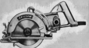
NEW SKIL SAW 77 (7%" Biade-Super Duty)-Speed increased 40% to 4500 r.p.m. and weight cut to 15% lbs. Power output boosted 100%. Depth of cut 2%"-Bevel cuts 2" dressed lumber at 45". Most popular SKIL Saw for all-round carpentry-the standard for general construction. Power to cut wer lumber or tough materials such as metal, stone, compositions.
