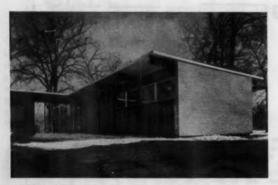
APPARENTLY PITCHED plank and beam roof is actually flat. Entrance of house at left of center is flanked with redwood slats in keeping with redwood front.
