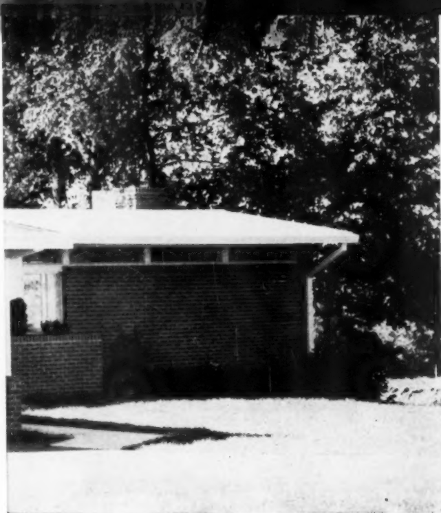
◀ TAPESTRY FINISH red brick exterior has contrasting white roof, V-groove vertical siding and white trim. Entrance door is red. Planters appear at entrance and on terrace.
