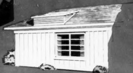
Houses of hip-roof design require only inclusion of an inconspicuous dormer to accommodate the unit.
