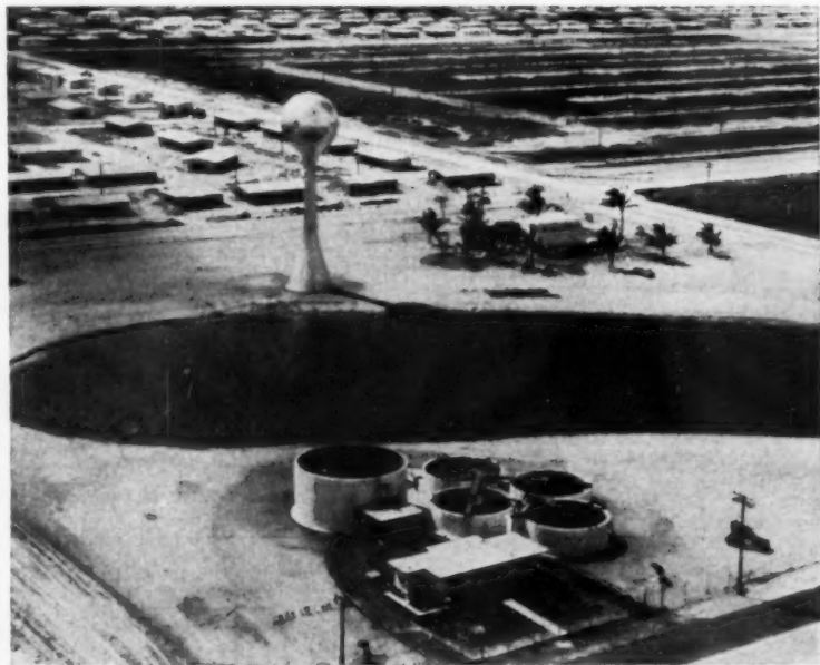
COMPACT sewage treatment plant set up as the Carol City Utility, Inc., to serve Julius Gaines' 10,000-home development.
