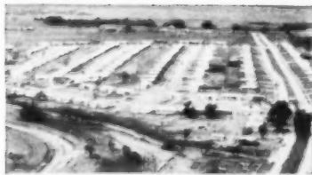
This is an aerial view of some of the homes being built by the Hines Building Corporation in Valwood Park, near Dallas. All 222 homes feature the birch and copper "Pioneer" by American Kitchens.
