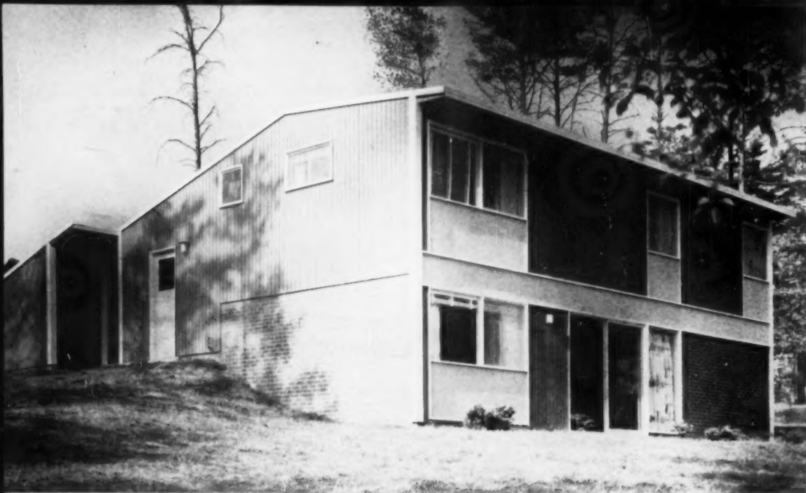
MODULAR HOUSE in McLean, Va. has exterior of common brick, plywood, with spots of architect-controlled color in window panels. Every effort was made by builders and architect to preserve sites, keep monotony out.
