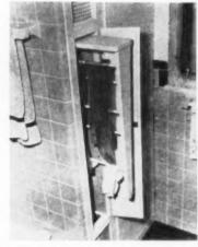
**BUILT-IN** lingerie dryer has heating duct at floor level. Warm air circulates around clothing and out at register provided at top. Racks slide out.
