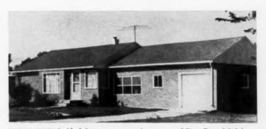
NAILON BRICK is ideal for new construction or remodeling. Remodeled house shown above was Nailon brick veneered over original clapboard surface.
