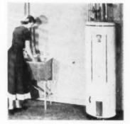
The important thing to bear in mind in selecting water heaters for new or old homes is the need for adequate capacity. In the 1920's, the average family found it possible to get along with a 20gallon gas-fired automatic water heater. By 1950, the increasing need for hot water required by laundering equipment and dishwashers, had boosted the average heater capacity to 30 gallons. How large a water heater does the average American family need today?
