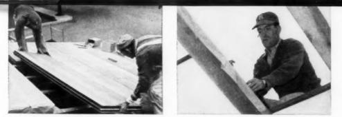
Each piece of Temlok Roof Deck provides 16 sq. ft. of deck, insulation, vapor barrier, and finished ceiling.
