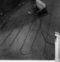
BY BRINGING EACH HEATING PANEL individually to a common header, as shown in the bailer hockup, and equipping each with its own valve, heat is easily and accurately regulated to suit individual room requirements.
