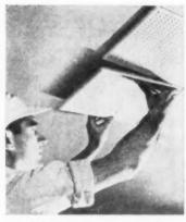
ACOUSTICAL TILE is easy to install, can be attached with adhesive, as above, or nailed to sleepers attached to ceiling. Cost: about 50 cents a sq. ft.
