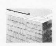
DETAIL OF HOW Rancho Ventura brick walls were laid. Note resemblance to standard Flemish bond.
