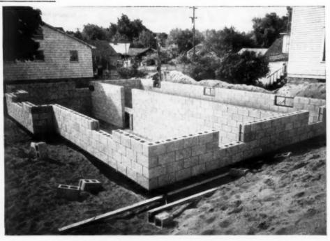
Basement for a Vibrapac concrete block home. Note standard 8" units can be used in center of basement as a bearing wall, instead of using conventional steel posts.
