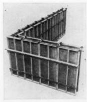
CORNER SECTION of outer forms shows plastic impregnated plywood walls, metal walers built-in to forms and adjustable panel clamps.
