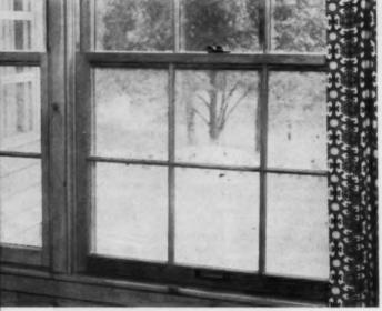
Wood, with its fine thermal insulating qualities, is exactly the RIGHT material for windows. Even glass is many, many times more efficient as a thermal insulator than aluminum. Try the touch test and you'll see why condensation runs down metal windows to make puddles on the sills.
