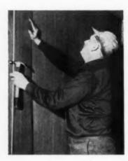
A FITTING the piece into place. There can be no second guesses, for the cement grabs. Or place a paper buffer between panel and wall; slide it out after the panel is aligned. Then panel is pressed to the wall.
