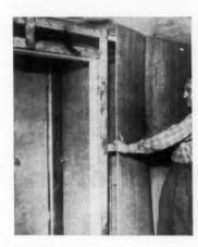
2 LAYING OUT. Plan sequence of panels around room for desired color and grain relations. Leave in place 24 hours to adjust to room climate. Start from corner or from both sides of a major feature.
