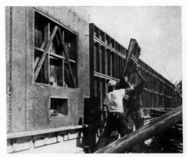
BUILDING GOING UP, Rocforms coming down. Forms simplify and speed concrete construction, are then easily
