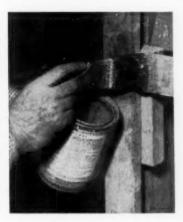
applying Additional Additional Better bond is achieved if one coat of cement is applied to the strips and allowed to dry, and then another coat is applied. Without addesive, the panel may bow and make the nails pop.
