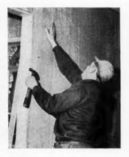
**5** PRESSING the whole piece to the wall. Here the random grooved plank effect offers some relief from need for perfect butting or matching of grain of adjacent panels. Grooves are spaced to occur at 16" intervals.
