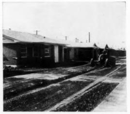
20 FINAL YARD GRADING is done by a small Allis-Chalmers "maintaining" machine. Several houses are finished at once in large developments like this, but such a machine saves money on a single job as well.
