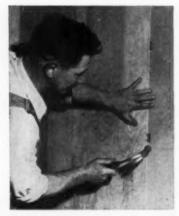
Tufacturers for specially grooved panels, hold panels to wall and join them together. Clips are held by nails, which must go through drywall, as in photo, to studs or furring.
