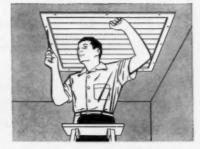
**Step 3.** Screw-fasten automatic ceiling shutter. Metal trim covers edges of opening. No finishing.
