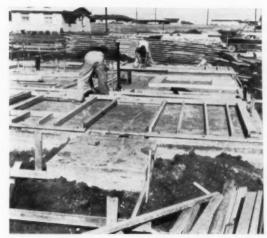
11 SHOES, STUDS, plates and frames for walls are laid out on slab by laborers. All timbers arrive at house in one bundle, cut to length and marked. Framing crews do no cutting, just lay out and nail.
