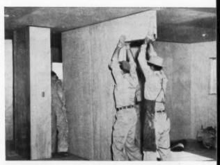
BEDROOM WALL section is moved into place by 3 men. Built-in sliding door is already in place, complete with all hardware. Shop-built components such as these make better product possible at lower cost.
