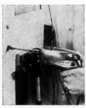
of scrap behind plywood panel, placed so that the bit emerging on the other side will not tear the fine wood grain. When using screws with hp panels, always drill pilot holes.
