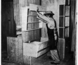
2 BATHROOM VANITY wall section goes into place easily, reduces need for skilled labor in building separate parts on job. Tutt Cooper predicts greater future use of built-in furniture in houses also.
