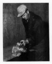
1 CUTTING a panel to fit. Portable power saw, cutting from above, requires that the good face of the plywood be turned down to prevent fuzzing the surface. (Compare p. 82, no. 2, for use of bench saw.)
