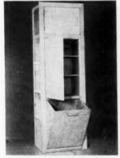
LINEN CLOSET, open here to display its adjustable shelves, hamper, and storage space. Above, Fabricator's 23 LH which is 2'3" wide, 1'10" deep, 7'6" high.
