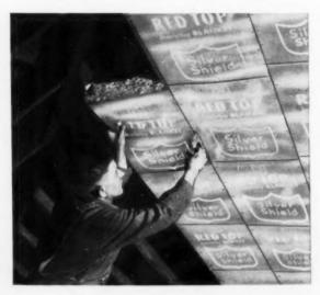
CUT COST OF AIR CONDITIONING—your biggest sale feature—by insulating your home with RED TOP\* Wool with the "Silver Shield". Reflective aluminum cover bounces back up to 95% of sun generated heat rays, when blankets are properly installed between attic roof rafters or floor joists. Hundreds of dollars can be saved on original central air conditioning equipment; operating costs are sharply reduced.
