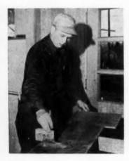
2 COATING the back of the piece with contact cement. Before this, the cut edge was planed and back-cut slightly to make a better butt joint. Various plywood manufacturers give instructions on use of own cements.
