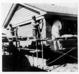
16 TWO-LEVEL STEEL SCAFFOLDING speeds work of bricklaying crew. Lower rows are done from ground, top rows from intermediate level. Top level serves as shelf for brick, is handy for roofing crew.
