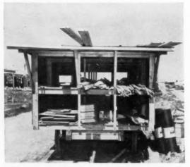
18 TRIMMING WAGON has bins built onto it, holds all trim for exterior, interior and cornices. It is towed by truck to whatever house is ready to be trimmed out, makes trim selection fast and easy.
