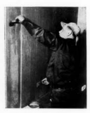
GOATING WALL. Each panel must be fitted and prepared separately for application at right degree of tackiness. The wall surface must be clean, bare and flat so adhesive will not pull away. Furr out plaster walls.
