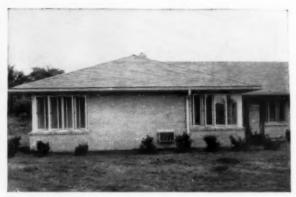
for instance-Curtis Silentite casements come in different styles-single light units as pictured and divided light in several arrangements. Sash are made 1'7" wide and 2'0" wide and may be grouped to fill any size opening. May be used with large picture sash for weather-tight window walls that are truly practical.
