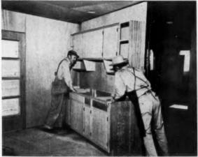
COMPLETE KITCHEN WALL section is shoved into place on Bates job by two workmen. Philippine mahogany cabinets and wall surfaces have furniture-like finish. The entire unit takes only a few minutes to install.
