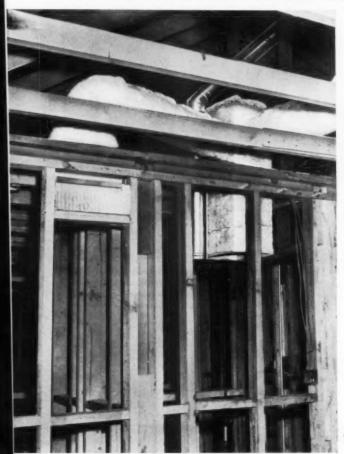
17 DUCT AND VENT PIPE are in place, ready to receive heater and air conditioner. Ducts in attic space are much easier to install than in slab. At right, the layout shows short duct runs.
