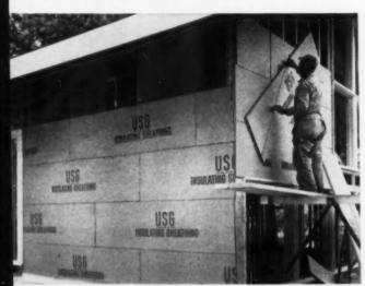
YOUR REPUTATION FOR QUALITY HOMES will be thoroughly protected when you provide added comfort with USG Insulating Sheathing. It insulates more than twice as effectively as nominal one-inch wood sheathing; "k" value is 0.33. Sheds water, repels wind, weather. Light-weight, yet so strong that FHA requires no corner bracing when the 25/32", 4-ft. width board is used. Saws on studs, saves valuable time.
