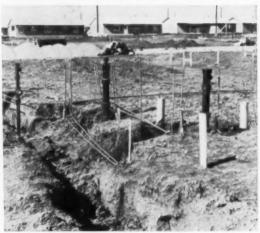
2 TRENCHES IN SLAB FILL are dug by backhoe, prefab plumbing sections are put in place by laborers. Higher priced plumber makes connections and tests. Standardized jobs are easy for lower cost help.
