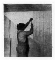
4 NAILING ONLY. Make sure to go through plasterboard into studs beneath, with small finishing nails or brads, which will be countersunk, and into plate and sill with heavier nails where moldings will cover.
