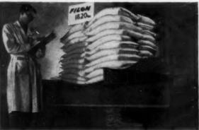
FILON HAS MUCH HIGHER LOAD CAPACITY THAN REQUIRED BY STANDARDS OF THE INDUSTRY. Shown above is a 26" wide FILON type 250 panel over a 4" span supporting a static load of 1820 lbs.—equivalent to 210 lbs. per sq. ft. Compare this with the 100 lbs. per sq. ft. required by industry standards.
