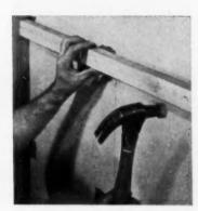
DRILL WOOD, NOT CONCRETE. With the new perforated anchor nails that are attached to a surface by powerful adhesive, you no longer need stardrill holes in masonry and fill with wood plugs or expansion bolts. Drill into the furring strips, hang them on the waffle nails, and clinch ends.
