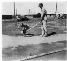
**5** GASOLINE DRIVEN POWER TROWEL is used to finish off newly poured slab after it has partially set up. Machine pays off in two ways: it is three times faster than hand work, and gives a smoother surface.
