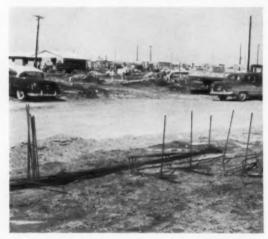
COPPER TUBING for water pipes is prefabricated into large section off the site. Smaller builders could have plumbing subcontractor do the same. Work like this done off site is better controlled, cheaper.
