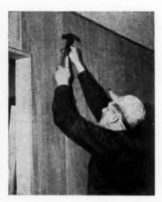
**6** NAILING with 4d finishing nails to plate and sill and along the stud to reinforce the cement bond. Nail holes are countersunk and filled with matching putty. In unfinished panels, fill holes after applying first coat.
