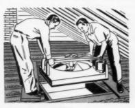
**Step 2.** Place Hunter Fan on attic floor or joists over ceiling opening. Easily wired from fan junction box.
