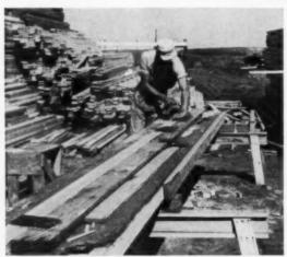
**9** HAND POWER SAW is used here to cut jack rafters to length. A simple jig like this is easily set up to different lengths; when used with a hand saw it permits changes of cut lengths.
