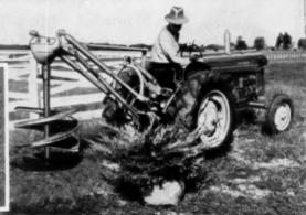
Above—The Utility Tractor and Power Hole Digger—today's easy method for digging holes for posts, guard rails, tree settings, and construction work. Digs as deep as 40 inches; several auger sizes.
