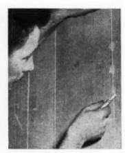
PUTTYING. Prefinished panels come with putty sticks of the right color for filling nail holes. In unfinished paneling, nails should be set and holes filled after applying first coat, usually primer or sealer.
