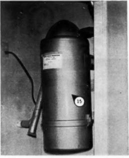
THIS 15 THE MOTOR that ends cleaning worries. Highpowered and heavy duty, has to be emptied only once every few months. The Vacu-flo equipment, a lightweight stretch hose and a few cleaning tools, is all that is used. The hose locks into an inlet upstairs, you flip a switch and you're ready to clean house. (Check 15 on reply cord.)
