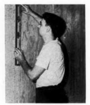
**9** A WARNING: keep checking for plumb. Shim out furring strips or fill hollows of walls. Keep a level on deck for true up-and-down. Molding will take care of irregular meeting with floor and ceiling.
