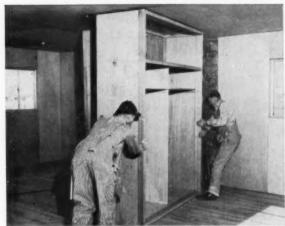
4 wardrobe component also acts as room divider, is set into place after finished floor is laid. Workmanship on unit is far more polished than is possible with small town local labor. Costs also are less.
