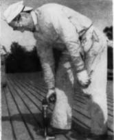
J. S. Stephens and Sons, Tampa, Florida contractors, used DRIVE-IT tools to speed the installation of the steel decking used as the roof of the Dunedin Shapping Center. Mr. Stephens used two model 330 DRIVE-IT tools to drive over 4,000 drivepins to anchor the steel decking to the steel roof trusses. Installations of this type average about 75% savings over drilling and other outmoded fastening methods. If you fasten anything to concrete or steel—you can save with DRIVE-IT tools.
