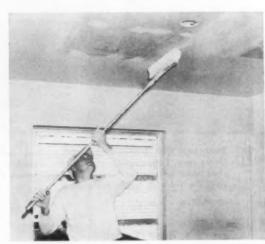
19 LONG-HANDLED PAINT ROLLER two feet wide lets painter do ceiling without ladders or scaffolding. Paint is latex-based, covers well enough so that one coat does job, gives attractive sand finish.
