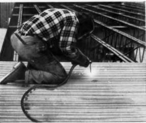
Ribform is easy to handle. Just weld it to the joists
