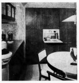
STORAGE WALL has planning compartment built in. Doors of St. Charles unit are two pieces straight grain white select birch (here finished in brown) on hollow core, hinged on steel cabinets.
