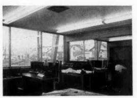
MODEL MAKERS' shop on lower level has gyp. board ceiling, post and beam framing. Benches are close to machine shop.
