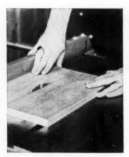
Power sawing. Face good grade of hp panel up when using bench saw. When both sides are good grade, as in cabinet doors, place a piece of scrap beneath plywood to prevent fuzzing the side that faces down.
