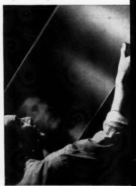
BUILD, INSULATE, CONTROL MOISTURE in one low-cost operation with Insulating ROCKLATH\* plaster base, applied to outside walls and top floor ceilings. Aluminum foil backing provides a superior vapor barrier, protects framing from damaging moisture condensation. Properly installed, it reflects 95% of sun-generated heat rays, keeping rooms up to 15° cooler—an important sales feature.
