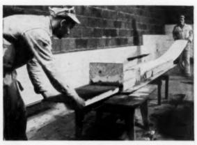
2 MORTAR of portland cement is applied to Styrofoam...
