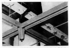
WAKEFIELD CEILING provides high level, flickerless light, and also serves to conceal water sprinkling pipes and air conditioning ducts, upper right. About 85 per cent of commercial buildings are poorly lighted.
