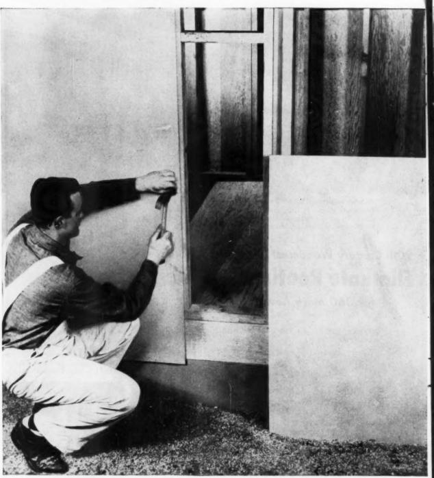
WHAT COULD BE SIMPLER? Duraply can be nailed right to the studs with no sheathing, no building paper. Big size of panels means you can close in a house in a day . . . save extra material and cost of installing them.
