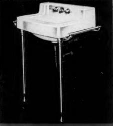
The Whittler is typical of the many Beautyware wallmounted models available in shelf-back, ledge-back or start-back design. Optional ledge and towel bars require no special well attachments—are simply installed.
