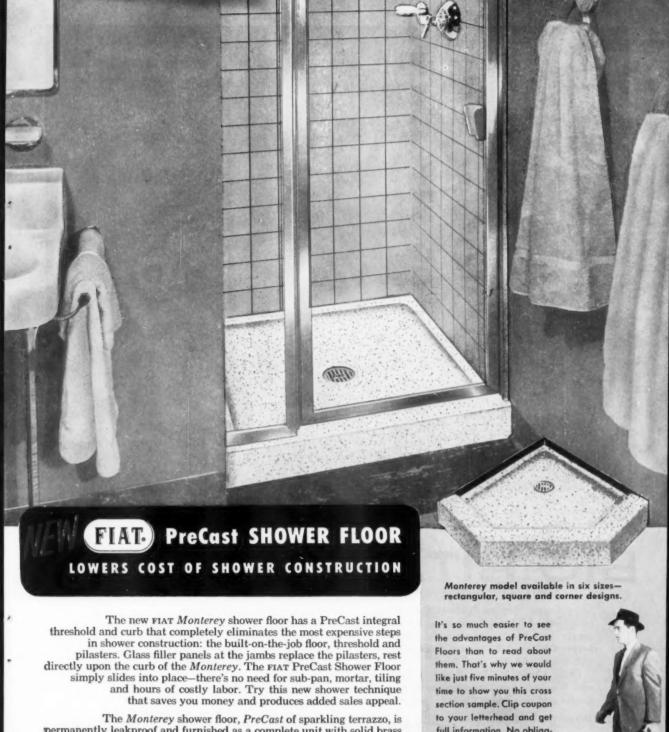
permanently leakproof and furnished as a complete unit with solid brass drain and stainless steel strainer plate. There is nothing else to buy -nothing else to install! The photograph shows an excellent and economical shower combining the Monterey floor with a glass filler panel and door forming the front. Either hinged or sliding doors, by others, may be used as the solid threshold provides a convenient foundation for the track.
