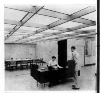
FOUR-FOOT MODULE of suspended ceiling is used throughout entire building. Light level is 100 foot-candles at wall. Ceiling is of acoustical baffles and plastic diffusers. Partitions are removable.
