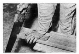
2 CUT SIDE DOOR jambs, and trim. Mitered joints where side jambs and head meet are not nailed. Note spring steel in the shape of arc.
