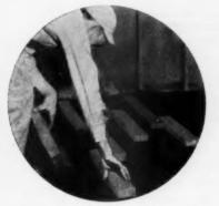
2. Lay short lengths of 2x4 on 12" centers. Lap joints.
