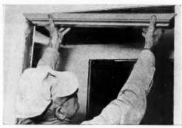
ADJUSTABLE door jamb and trim is redwood. Here, workman is placing the head but does not nail it in place. Head is screwed in place later.
