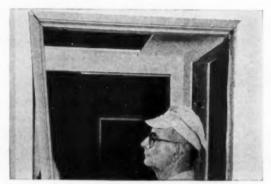
PLUMB AND SET hinge side. Use shims under hinges. Plumb and set opposite side. Apply shims here too if necessary. Pull head down and fix.
