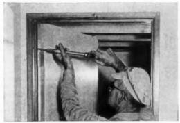
WHEN DOOR is hung and jambs and head are in place, adjust jambs and head to proper alignment. If door sticks later adjustment can be made.
