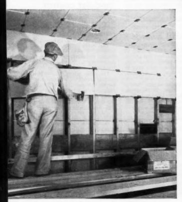
SECRET OF CRACK-RESISTANT WALLS is the spring steel clips used with U.S.G.'S ROCKLATH Resilient Lathing System. The plaster base is floated free from framing, which provides maximum resistance to cracks due to structural movement. Also provides extraordinary resistance to sound transmission (loss rating up to 47 decibels).
