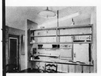
SLANTED CEILING in builder Walter Tally's house, Atlanta, Ga., uses recessed slimline tubes in kitchen, pendent fixture for dining area. Installation of slimlines at right.
