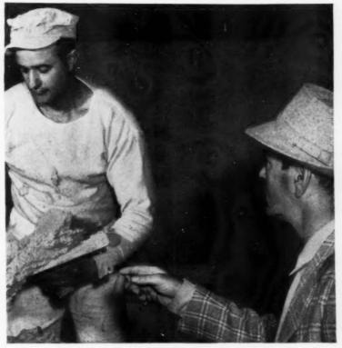
only the addition of water—saving time and materials. In many constructions it fights fire up to twice as long as sanded plaster, yet is 50% lighter in weight. Stabilized set assures maximum strength of the plaster slab.
