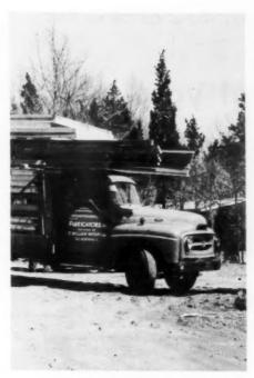
2 COMPLETE SHELL arrives on site in one truckload. If truck can be spared, ideal arrangement is to park it, erect parts as they're unloaded.
