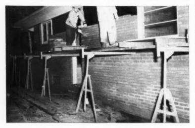
FOR FAST MASONRY CONSTRUCTION, mason contractor L. Hubbard of Euclid, Ohio, uses new "Trouble Saver" Putlog Trestles on a project for Joe Miller Homes Co. The new Putlog Trestles are 5'-long and provide nine height adjustments, ranging from 4' to 6'. Masons set each Putlog on the top course, then brick is laid over them. Putlogs are pulled out of the wall and adjusted to new height as the job progresses. When a pin is removed, the new Putlog Trestle swings down flat for easy storage or shipping.
