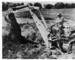
180 DEGREE BOOM SWING is one of the features of the new TerraTrac backhoe. Designed for heavy-duty use with TerraTrac crawler tractors, the 180° swing is done with hydraulic foot pedal control, enabling operator to maneuver bucket and dipper stick while swinging. Unit digs 12½ ft. deep, has 18 ft. reach and 13 ft. dump height. Easily detached when using front-mounted loader or dozer. From American Tractor Corp., Dept. AB, Churubusco (Ft. Wayne) Ind. (Circle No. 10030 on page 154).
