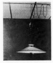
TRAVELLING FIXTURE by Lightolier. Shallow parasol shade fixture called "The Traveller" is suspended by a counter-weighted cord, glides across ceiling on slim brass track as far as 72". Fibreglas shade ribbed with walnut strips. About \$72. From Lightolier Inc., Attn. J. Levine, Dept. AB, 346 Claremont Ave., Jersey City, N.J. (No. 10034 on page 154).
