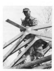
ROOF TRUSSES come with pitches from 1½" on up, spans of from 12' to 36'. Prices are from \$15 to \$45.
