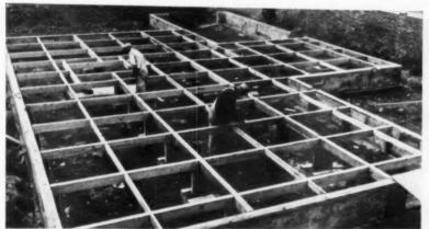
Weldwood 2.4.1 plywood will be installed on this 48" o.c. "grid system." Once it's nailed in place, you're ready to lay finish flooring.
