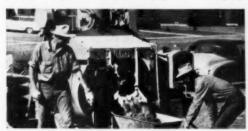
Pours 60 yds. a day with Jaeger 6S Speedline mixer. Mixer and 7 man crew (3 loading, 3 wheeling, 1 operating mixer) averaged a batch every 194 minutes pouring footers and floor slab. Famous "Skip Shaker" loader speeds batch into drum in 5 to 7 seconds. Discharge is just as fast. Criss-cross double mixing action assures uniform quality concrete.
