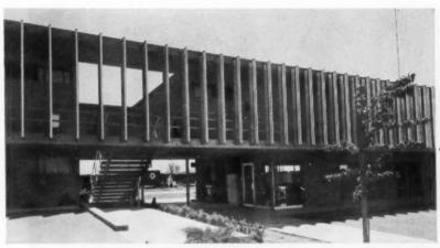
MAIN ENTRANCE TO MOTEL is at center, where walk leads past manager-owner's office to heated pool in rear. Parking space is under balconied upper story. Louvers were installed for design purposes only; motel faces North. Stair treads of poured concrete have V-shaped metal pans.
