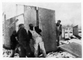
COMPONENT SECTIONS enable the builder to erect walls and roof quickly. Tricky work like measuring and cutting, hard in awkward mittens, is done in the shop.
