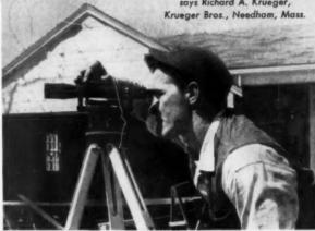
"Here's how: we figure a clear saving of \$60 per house on labor, gravel and cement by getting 'on-the-button' accuracy in measuring excavation depths, establishing foundation heights and grades for drainage and streets. Focusing our Berger Dumpy Level is quick and easy; optics are clear as crystal - which cuts time in setting up batter boards, leveling off first floors within 1/16th inch and installing the first course
