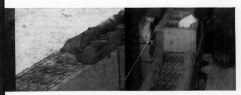
MORTAR FLOWS READILY around KEY-WALL to give full embedment, as well as maximum reinforcement value. Tests show an exceptional bond. MASONS LIKE the way mortar flows over Key-Wall; the way it aids full embedment; the way blocks settle in place without interference.
