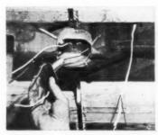
SIX-VOLT remote control system by Remcon (Pyramid Instrument Corp.) uses standard outlet box and miniature relays. Because of low voltage, small bell wire can be used. Installation of low voltage relay system in Oceanside, Long Island, homes of builders Ballin, Glicksman and Langfur was big but economical sales feature.
