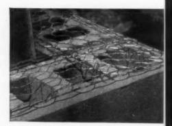
KEY-WALL is lapped at corners without adding thickness to the joint; without special cutting and fitting. It's easy to build up Key-Wall reinforced corners.
