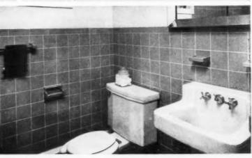
The adhesive method was used to apply ceramic tile to the bathroom walls and in the inviting shower enclosure. Alert use of progressive new techniques like prefabrication and adhesive installations help to sell homes at a fast—and profitable—rate.
