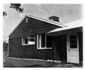
EFFECTIVE USE OF SIDING is seen with horizontal gable lines contrasting with battens below. Height of garage in relation to house can be shifted up and down to meet terrain changes, helps alter appearance of house.
