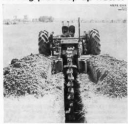
**TRENCH-HOG** is Arps low cost tractor attachment to handle big yardage jobs. It is available in three boom lengths, with digging depths of  $3\frac{1}{2}$  to 7; cutters available 6 to 20" wide. **Circle No. 10002 on reply card, p. 134.**
