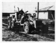
Quick back-up (to 13.7 mph) saves time in shuttle-grading. Wide forward speed-range gets more work done in less time.
