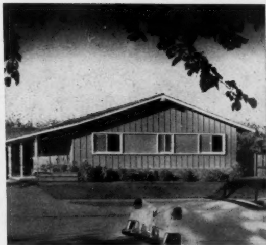
5 THIS FINISHED HOUSE was built from an O'Neill package by Brown and Kauffmann of Palo Alto. They estimate precutting costs them $50 extra per house, but saves them many times that in speed and efficiency.
