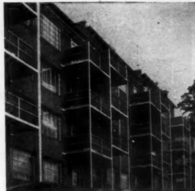
Washington Vista Apartments, Roslyn, Va. Here Builder Phillips used big, 25-light steel casement windows so that tenants can enjoy the magnificent view from their hilltop location.
