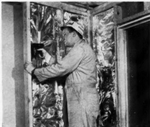
ALUMINUM FOIL OR COATED sheets are especially effective as a heat reflector. "Twinsulation" combines aluminum with rock wool. National Gypsum Co., Dept. AB, 325 Delaware Ave., Buffalo N.Y. (No. 2048, p. 156.)
