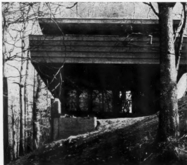
SIDE VIEW shows how the house sets snugly into the hill, despite the steepness of the slope. Balcony above opens off the master bedroom, also serves as a roof to make the lower-level patio into a weatherproof front entry.
