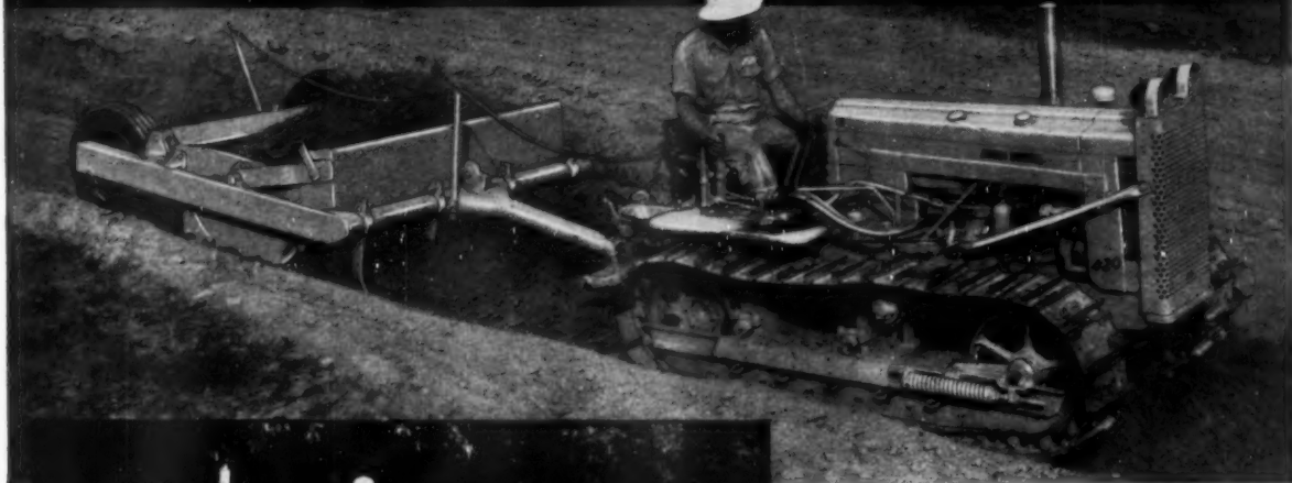
John Deere crawler tractor excavating for sanitary landfill. This low-cost crawler, with its 30 engine horsepower, is just right for many municipalities.
