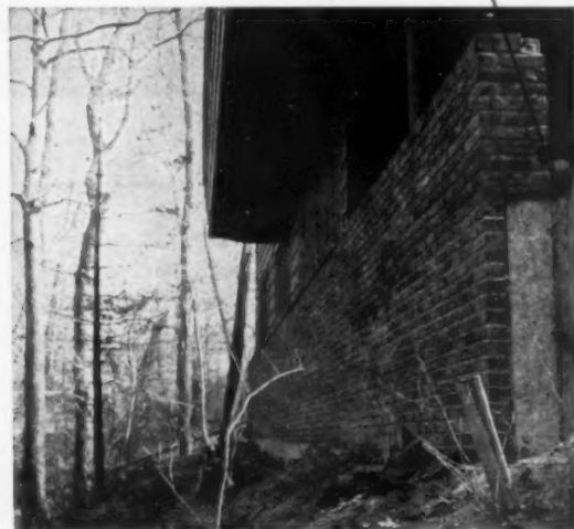
BRICK VENEER makes this attractive finish on the front of the wall. One of the extra expenses when such a house is finished, is landscaping. Planting, plus extra costs for walks, steps and drive may run as high as $500.
