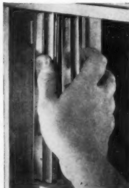
Dura-seal and complete sash balance easily snaps in or out of the four Snap-Clips with slight finger pressure.
