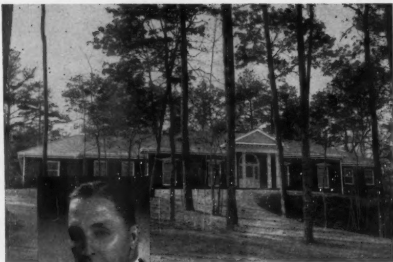
CUSTOM BUILDER —W.C. Knight, Atlanta Georgia, builder of five to ten $50,000—$80,000 homes per year, similar to the Knight-built home above.
