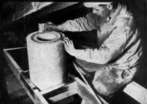
Completely packaged Van-Packer Chimney installs in 3 man hours
