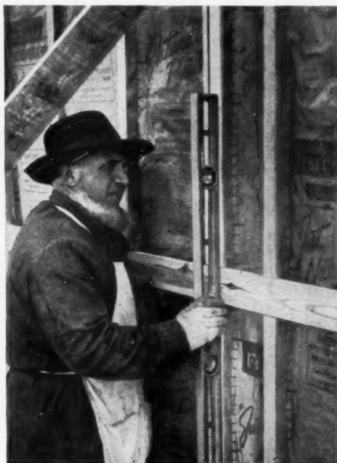
EXTRA RIGIDITY —Note how 1" x 4" half-stud on one edge of panel joins 2" x 4" stud on next panel to make a 3" x 4" support every 4 feet. Notched-in 1" x 4" nailing-strip across mid panel is another American Houses' extra feature.
