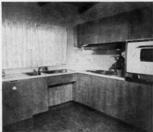
ARCHITECT-BUILDER QUINN designed the cabinets in the kitchen to resemble fine furniture, used walnut plywood, Micarta Unitop and Westinghouse appliances.
