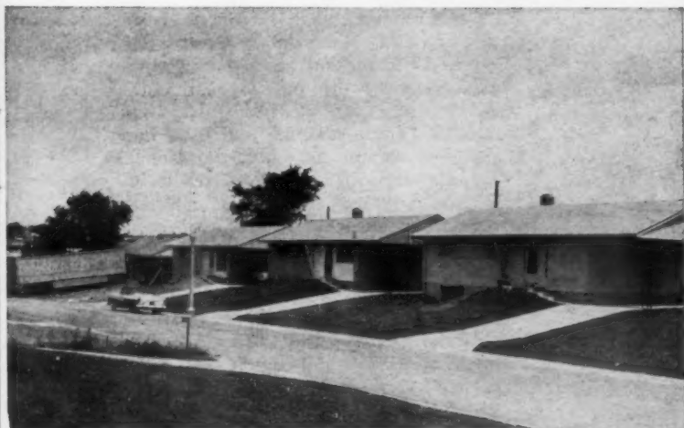
ATTRACTIVE Eugene Field 29-home subdivision of Wilson Homes in St. Louis has concrete streets and 56' frontage. Unbroken gabled roof extends over carport, located off kitchen. Two-foot overhang makes roof look low. Delivery was geared to sales.
