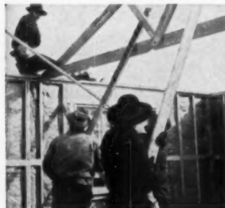
SELF-SUPPORTING TRUSSES —American Houses' rink-type split-ring trusses require no support. Inside partitions carry no load. Walls and partitions are notched for quick, accurate spacing.
