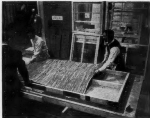
LU-RE-CO WALL PANEL is built in demonstration. The 2x4 frame has already been assembled on the jig table, and the blanket-type insulation is going on. Jig is simply pieces of angle iron bolted to a plywood table.
