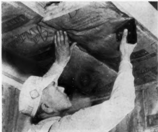
MINERAL OR VEGETABLE FIBER-TYPE insulation usually comes in blankets or a roll to be cut off at end of joists. Here, Owens-Corning Fiberglas, Dept. AB, National Bank Bldg., Toledo 1, Ohio. (No. 2047 on p. 156.)
