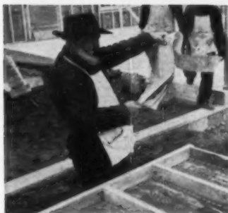
UNITITE PANELS —Basic element of American Houses' construction is the 4' x 8' Unitite Wall Panel, ready-to-erect with insulation in place.
