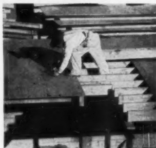
PREASSEMBLED FLOOR PANELS —American Houses' floor panels are factory-assembled with subflooring nailed to joists for speedy installation.
