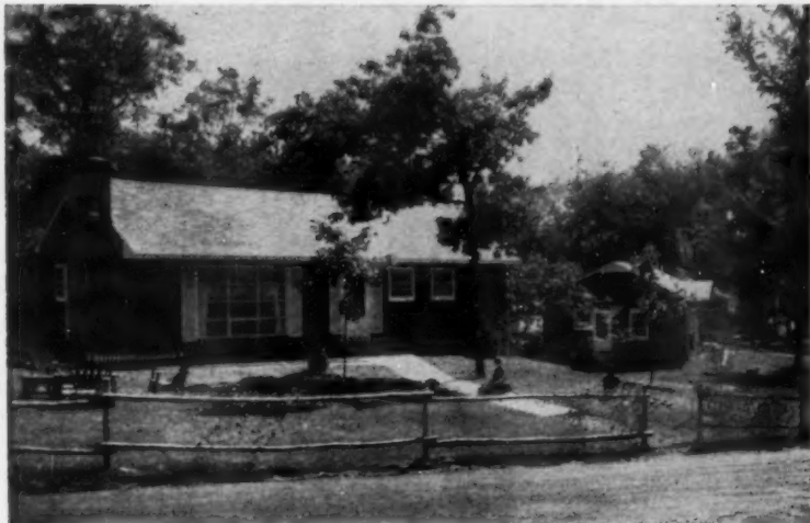
WOODED TRACT of well-contoured rolling land, convenient to Twin Cities, is being developed by Maple organization with 85 Page & Hill units. Shown is 40'x24' model, with two fireplaces and built-in garage, sold for $13,500 with land.
