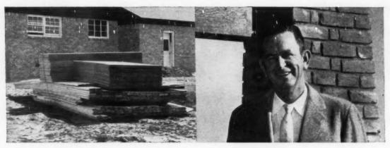
**Stockplies at job site** need little protection, as Insulite Sheathing comes through any weather safe and sound. Latch takes deliveries in large quantities, drops enough for each house near the foundations.
