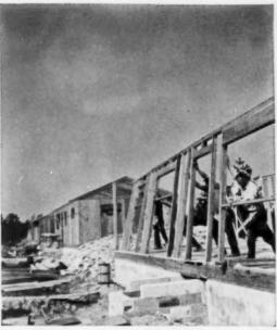
FRAMING: all parts of the building operation are aimed at speeding up the work of the man in the field. By getting the house under roof quickly, bad weather can be kept from slowing down crews, hamstringing the whole operation.
