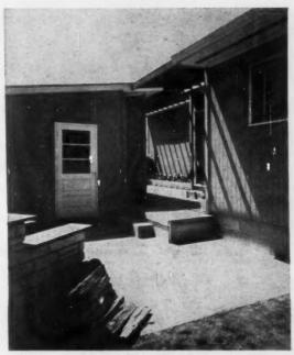
HIDDEN VALUES like waterproof cement block foundation and vented soffit provide sound selling points. Outdoor grille is optional, but long planter along raised terrace wall is included in basic price.
