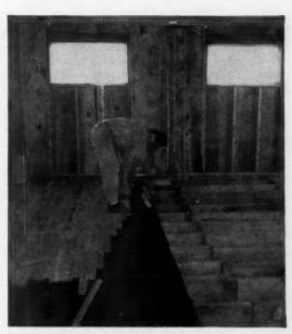
HARDWOOD FLOORING is laid directly over joists instead of having a sub-floor between. Roofing felt serves as a sealer and noise-deadener. Besides eliminating sub-floor, method saves by allowing one-big-room floor job.
