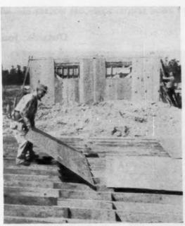
PLYWOOD SHEETS are spread out over floor joists so exterior walls can be assembled. This is not subflooring; when the walls are up, the plywood will be taken up and sent to the roof, where it will become the roof sheathing.
