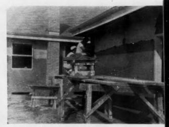
STUCCO is troweled-on over the insulated wire mesh panels forming the outside wall surface. In future, the stucco as well as the plaster can be integrally colored and sprayed on. Aluminum siding or brick veneer can also be used.
