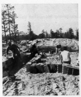
FOUNDATION WALLS for crawl space are the first step in building the shell. Considering the sandy soil and his method of installing floors, Schmertz says this is better than slab construction, the wood floors easier to sell.
