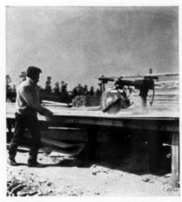
**POWER TOOLS:** properly set up and used, they permit a man to do many times the work he could do using hand tools. And heavy equipment, like this radial saw, speed up ripping and cutting operations even more.
