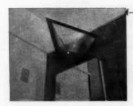
LIGHT FIXTURE over medicine cabinet in bathroom (and other fixtures) is made of a wood frame and frosted glass, uses simple light sockets.
