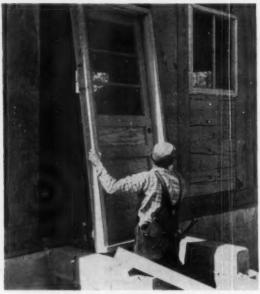
PREHUNG EXTERIOR DOOR is set into place. Schmertz does his own prehanging and millwork in two shops that are really just unfinished house shells. Two more of these shells serve as warehouses for finished millwork.
