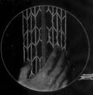
KEYBEAD corner lath with precision formed bead for outside corners. Open mesh assures strong, solid plaster corners.
