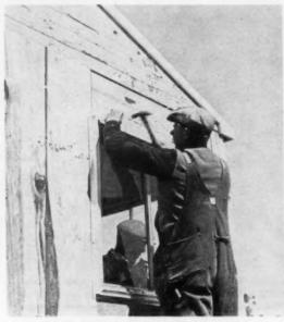
**ALUMINUM SLIDING WINDOWS** are nailed onto the facing of the window frame, require no fitting or shimming. They are made waterproof when the siding laps over the flanges and caulking compound is added to all joints.
