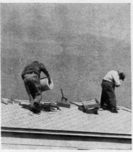
PACKAGED PREFAB CHIMNEY for the furnace is quickly installed by a two-man crew. Schmertz buys the packages, but subcontracts the actual installation of them. The cost, representing purely labor, is \$10 per house.
