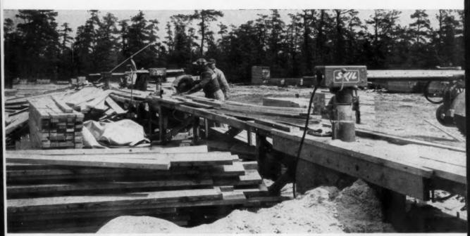
"ASSEMBLY LINE" of the prebuilding yard is this long table with its three heavy-duty radial saws. Here, all parts of the house are cut precisely to size. At intervals, all
