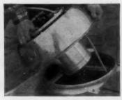
**3** BX CABLE is run through fittings; Kitchen-Aire positioned over flashing and connected to attic duct. From Stewart Industries (No. Y8, p. 128).
