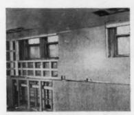
DURING: Walls, ceiling are framed and Korelock, a hollow-core hardboard paneling, is easily applied.
