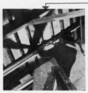
FIR PLYWOOD panels, based on 1x3" nailers alongside each rafter, were fitted inside to allow ½" exposure of original ceiling rafters.
