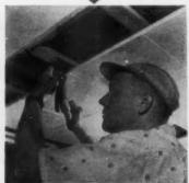
CEILING TILE went up next with help of Insulite clips. Clips were inserted along edge of each tile, then nailed directly to the furring strip.
