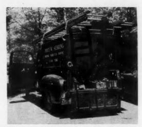
THE RIGHT EQUIPMENT has to be readily at hand, particularly for the little, less-than-a-day jobs. This is Sebring's "one-stop" maintenance truck, which carries supplies for fixing anything from a roof to a cellar.
