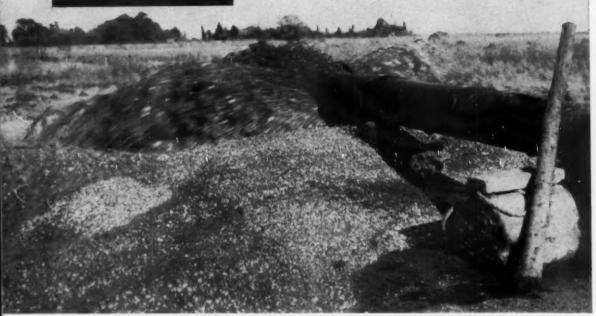
A THOUSAND YARDS A DAY of fill can be dug, moved and pumped in this dredging operation.
