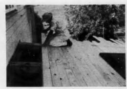
TONGUE-AND-GROOVE decking goes down next. Underside provides finished ceiling. After deck is completed, overhang is cut with power saw. Deck's thickness is intrinsic insulation—a "hidden value."
