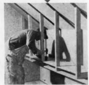
BASE SURFACES were covered with plywood; then framing for storage bank under eaves went in, leaving space underneath for roll-out day beds.
