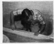
1 TUB ENCLOSURE to up-date the bathroom. Job begins with cutting of sill section, and installation after application of adhesive.
