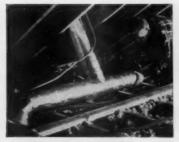
2 DUCT GOES into attic. Seveninch spur goes to range hood; shorter duct to intake grille in bath. Same ventilator will serve both rooms.
