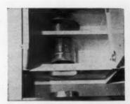
1 VENTILATION for kitchen . . . duct cuts through cabinet to fit hood at bottom. At finish, loose duct is pulled down to slide over collar.
