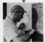
WALL FINISH of Durolite Plank was easy to apply because of its t&g nailing flange. Plank was stapled through flange to furring strips.
