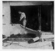
WALL IS REMOVED to accommodate door which reached job site as a complete unit. Worker assembled frame at the site.
