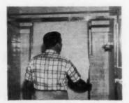
3 DOORS LIFTED together as unit and placed with head lowered onto top of jambs and filler strips. From Ludman Corp. (No. Y7, page 128).
