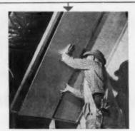
BETWEEN RAFTERS went blanket wool insulation, then ½" plywood panels. Ceiling was braced by 2x4s with plastic panels to conceal lighting.
