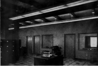
Office Interiors in Dykstra Annex appear extra spacious and roomy with sloping open-beam ceilings. Photo above shows a typical attractive, airy office, finished at modest expense. Beams are glued-laminated wood type,  $3\frac{1}{4}$ " x  $11\frac{1}{4}$ ", 4' on centers. Maximum span here is 21 feet.
