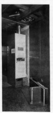
CORNER COOKING unit is only 27%" thick, has electric water heater installed below. Philco Corp. also designed new-type kitchen cabinets.
