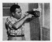
2 JAMBS ARE SECURED to tile walls with long flat-head wood screws after drilling is completed and rawl plugs have been inserted.
