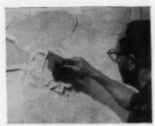
1 PLASTIC TILE goes on more easily, with new plastic grout strip. After applying adhesive with trowel, tiles are snapped into position.
