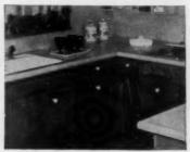
3 AFTER SURFACING is completely bonded to countertop, openings are cut for sink and range. Armstrong Corp. (No. Y9, p. 128).
