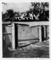
FOR MOTELS, SUBDIVISIONS, etc. the "Du-O-Ject," a "hidden value" duplex pneumatic sewage ejector lift station which gives fast, continuous action. Manufactured by Smith & Loveless. (Circle No. Z23, on p. 114).
