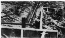
HIDDEN VALUE in the truest sense of the word is castiron soil pipe which Norman lays before foundation goes down. Care is taken to seal joints with poured lead.
