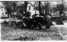
Mr. Reinhardt's HENRY BACKHOE digs a ditch for a sewer line in a Pontiac residential district. Though soil is laced with tree roots, digging goes ahead smoothly
