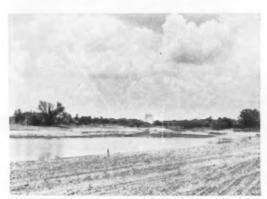
FINAL GRADING has been done on the bottom here, and lake is beginning to fill. Areas close to shore drop off sharply to prevent weed growth, but vegetation is left in
