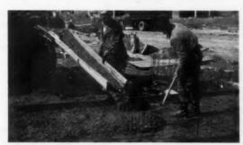
HIDDEN VALUE added to every house at Aurora Gardens is steel-wire reinforced driveway. Sidewalk is put in with similar reinforcement—gives sidewalk longer life.
