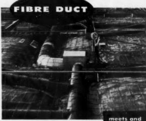
The perimeter heating-cooling system for this \$30,000 residence included a GE Weathertron heat pump and economical Sonoco Sonoairduct fibre duct. Lightweight, long-length Sonoairduct was easy to handle and level, thus saving time, labor and money in installation. By mitering the duct, all T-joints were made Without metal fittings.
