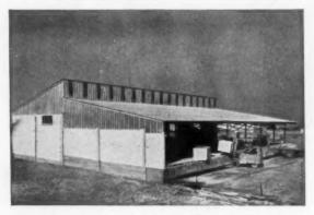
THE STABILITY of rigid frame construction provides a greater capacity to withstand winds, snow, cranes and "bumps" from materials handling equipment. Steel spans also mean more clear working space. This is just what Hansen Lime & Stucco wanted for their new Salt Lake City warehouse and shipping shed...so they specified steel framing, and USS StormSeal roofing and siding.
