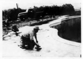
CEMENTING THE APRON isn't any different than a cement job on a house. Roether used his own masons to do work. When crew finishes, the pool is completed.
