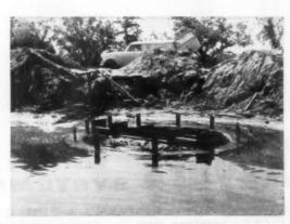
**DRAIN AT END OF LAKE SHERWOOD** serves as overflow to maintain a constant water level, also allows the whole lake to be drained dry for future cleaning.
