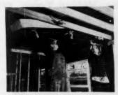
SIX-INCH THICK insulation of spun mineral wool batt suggested as "hidden value," particularly for builders of air-conditioned homes. From Baldwin-Hill Co. (No. Z21, p. 114).
