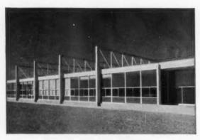
MANY COST-SAVING POSSIBILITIES result from the use of steel framing and wall panels. Curtain walls, for example, are faster to erect and provide more usable floor space. Steel framing eliminates bearing walls and reduces amount of framing. The school pictured above features an all-welded frame which helped make it Utah's least expensive (per square foot) school.
