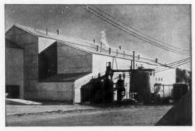
NO COSTLY MAINTENANCE PROBLEM HERE: This new Uranium Mill on the Colorado Plateau is frequently attacked by sand and snow storms. For maximum protection and minimum maintenance, steel roofing and siding was the obvious answer for these buildings. Steel framework leaves interiors open and flexible.
