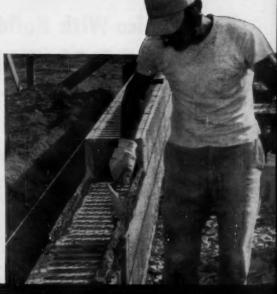
Mr. Ehman finds that mortar flows in, under and around Key-Wall to give exceptional bonding and provide full mortar embedment. Key-Wall is galvanized for protection against weather, assuring a strong bond. It is easy to store on the job. 200-ft. rolls are compact, and can be carried with ease.
