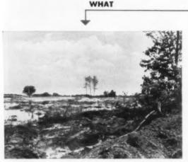
ROUGH EXCAVATING of the future lake bottom is done with dragline cranes. Cole-Easlick uses six of them like the one shown at right. Before joining with Cole,
