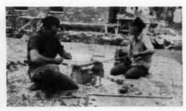
HIDDEN VALUE is this copper tubing which plumbers are preassembling here before frame goes up—a step which cuts time and labor costs from the overall expense.
