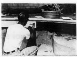
**TILING AND COPING:** one of the last steps before completion of pool, can be done by your own contractor. This work does not have to be subbed-out.
