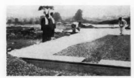
HIDDEN VALUE here is the spreading of polyethylene vapor barrier—almost a necessity in the high-moisture New Orleans area. Product is Visqueen by Visking Co.
