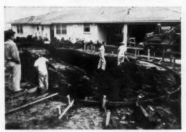
**EXCAVATING** the pool came to \$125. Roether's regular crew dug up 79 cu. yds. of earth. The same crew does the earth-moving work for Roether's new homes.
