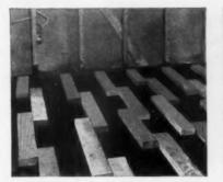
4 Lay screeds flat side down in staggered pattern on 12" centers at right angles to proposed direction of finished floor. Lap joints at least 4".
