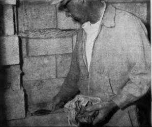
"I build a chase in the wall. Pipes, ducts and con-duits are easy to install when KEYWALL is used. I run the KEYWALL right through the chase," Mr. Gans explains. "The center mesh can be cut away as required without destroying the reinforcement value
