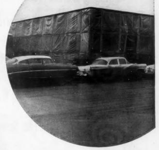
Carl Mitchell and Ralph Hulshizer, job superintendents for Garmer and Stiles Company, general contractors, Des Moines, Iowa, kept their jobs on schedule through snow, sleet and freezing rain by using Olin Polyethylene film as a wind and weather break.
