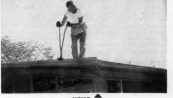
Fing below, arrives on the job with its hooking member set at about a 30-degree angle. Roofing pan easily slips under, and is clamped down with large hand clamps, left. Fascia on the eave edge has a series of openings about two inches in length, an inch in width, to break up flow of water from roof. On a conventionally-sized house, this roof could be installed by experienced men in five hours.
