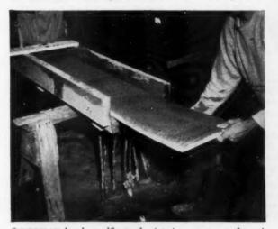
"STYROFOAM bonds readily to the interior masonry surface. A uniform layer of cement mortar is applied by running the 1' x 9' boards through a coating trough."
