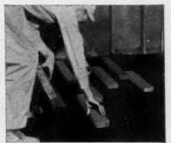
**3** For screeds, use flat, dry 2x4s in random lengths from 18" to 30". Screeds should be preservative treated to prevent rot or termite damage.
