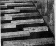
5 Leave a minimum gap of 1" between ends of screeds and baseplate around edges of room to allow for normal expansion of the finish flooring.
