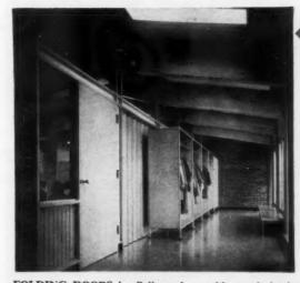
FOLDING DOORS by Pella and movable wardrobe by Fleetwood Products allow the classes to expand into corridor. In detail at right, pipe column carries roof load from truss to foundation.
