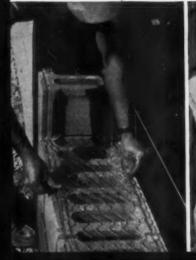
"I have no problem getting ma-sons to lap KEYWALL. I prefer a 2-foot lap. When it's lapped, it doesn't interfere with the embed-ment. Yet it gives the full rein-forcement value of continuous wire," Mr. Gans points out
