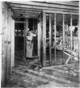
**ELECTRICAL** sub-contractor completes the rough wiring in three hours. When construction has progressed sufficiently, he returns, installs finished wiring in another three hours. This includes two TV outlets.
