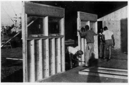
WINDOW AND DOOR PANELS, with their relatively complex assembly, are bought assembled and glazed. Solid walls between panels are measured and built on the job.
