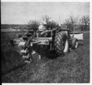
**REAR-MOUNTED TRENCHER** turns tractor into an efficient ditch-digging machine. There are many models on the market. This one, by Earth Equipment Corp., digs four-foot trench at the rate of up to nine feet a minute.
