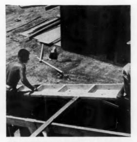
**RAKE OVERHANG AND SOFFIT** is brought pre-assembled, is nailed in place and cut to length. This allows a simple, flat gable truss, speeds up what is normally one of the "messiest" little jobs on any house.
