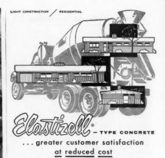
You can offer your customers extra living comfort with floors of this insulating concrete. Even the cheapest heating system will perform with maximum effectiveness when used with an Elastizelltype floor. For further information as to the performance of this type floor, inquire through your ready-mix supplier or write us direct.
