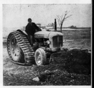
HALFTRACK ATTACHMENT by Arps greatly increases traction, makes it possible to use tractor in sloppier ground. While this does not make tractor a bulldozer, it does permit light dozing jobs like the one shown.
