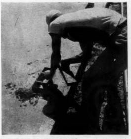
FORMS FOR REGISTER HOLES are set in after slab is poured; done earlier, they'd get in the way of screeding. Disturbed area is easily smoothed. After slab sets, the top of the ceramic duct can be broken through.
