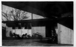
**"Board and Batten"** siding is easily achieved by applying Exterior fir plywood vertically and covering with moldings.
