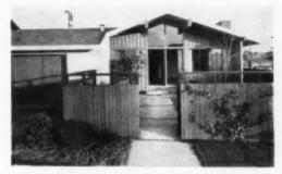
FENCES with a vertical surface should be made of resawn or rough board so stain will penetrate.
