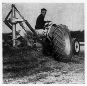
HOLE-DIGGERS come in diameters of from 6" to 24", can dig holes up to 6' deep. They dig holes for poles, planting small trees, or for concrete piers under gradebeam slabs. This one is made by Roper Mfg. Co.
