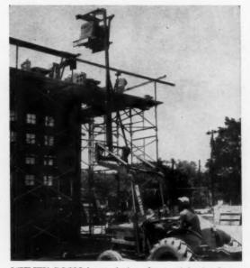
UTILITY BOOM is attached to front-end loader frame, can lift material up to 20 feet, high enough for two-story houses. One accessory is a one-third yard concrete bucket. Made by the Henry Manufacturing Co.
