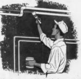
Aluminum enamel is the ideal protective and decorative finish for hot-air ducts, steam pipes, radiators and other metals exposed to heat. Good for temperatures ranging as high as 800° F.
