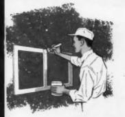
Paint all metal components with Aluminum Metal and Masonry Paint for longer life and better finish coats.
