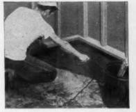
2 With moisture barrier in place, apply mastic to secure screeds over entire slab surface or in "rivers" along lines where screeds will be positioned.
