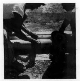
**CERAMIC HEATING DUCT SECTIONS** are joined with plastic tape. Ceramic requires no pre-poured concrete bed, does not float during pour. Note polyethylene vapor barrier, foam insulation, and 2x4 sill bolted to blocks.
