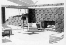
Shadowal block for the home adds new dimension and character to a room. The standard modular 8" x 16" face makes it easy to lay-up in the wall.
