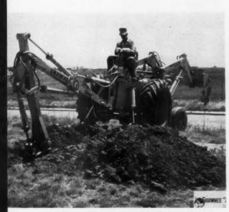
**MOST IMPORTANT ATTACHMENT** for most builders is the backhoe. Average unit can dig about 12 feet deep, has buckets from 12" to 24" wide, can dig anything from a sewer-line trench to a full cellar excavation.
