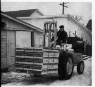
FULL-FLEDGED FORK LIFT machine is a luxury the small builder can't afford; but with this fork-lift attachment on his tractor, a tremendous variety of materialshandling jobs can be done. Manufactured by Oliver.
