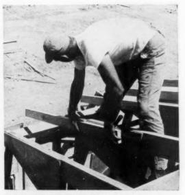
**OVERHANG OUTLOOKERS** are added after trusses are up. Set to a line, they are perfectly straight this way. As part of trusses, they'd be crooked, would make truss handling harder, might break off.
