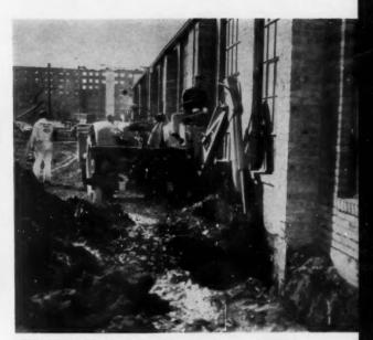
NEW VARIATION on the old backhoe is this unit, which works from both sides of the tractor as well as the center, permits digging close to existing walls. Mid-Western Industries is the manufacturer.
