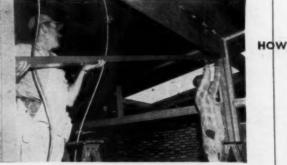
**EXTRUDED** C-shaped aluminum section goes up over beam. Drawing, right, shows how sections and 1 X 3's are assembled on post.
