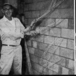
Wherever walls intersect, Mr. Gans uses KEYWALL to tie them together. "It is easy to place in alternate joints as shown," he explains. "And KEYWALL bends out of the way, removes the hazard of projecting rods or wires."
