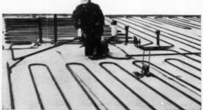
Welding joints of steel pipe on the job for Radiant panels.
