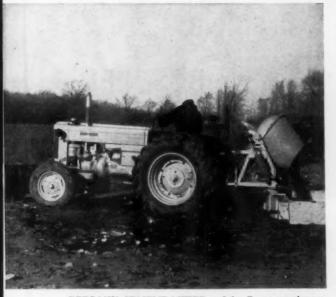
**REDI-MIX CEMENT MIXER**, a John Deere attachment, mounts on the rear of the tractor. Small mixer is standard item for most builders; by attaching it to the tractor, builder is able to mix and deliver to job at the same time.
