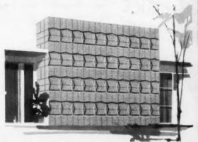
Shadowal block for the exterior of industrial buildings gives the effect of expensive special shapes at only slightly more than the  $8" \ge 8" \ge 16"$  units.
