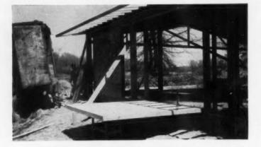
Wall panels follow framing and roof assembly; are non-load bearing, since basic construction of house is post and beam. Panel is a plywood sandwich with insulation already installed at factory. Sections between solid panels will be closed with glass (double glazing optional) protected on the outside with an aluminum grille. A 12' module was used, includes, two glass sections and one wall panel. This photo shows front elevation.
