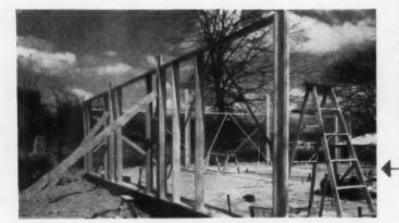
Wall framing sections and panel components were assembled by National Homes in its Lafayette factory. Rabbeted 2x6" frame is made to receive flanged panel (see photo below). Termite shield of extruded aluminum (drawing below), serves also as drip cap, slab stop. Pre-assembled posts are used at corners.
