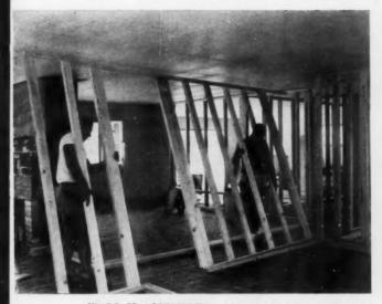
WALL IS ASSEMBLED with one-inch shoe on bottom, plate on top. Studs are cut on job to match shortest distance between floor and ceiling. Wherever possible, studs are set the short way to allow more living area.
