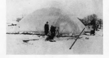
Polyethylene sheet is one of the most versatile materials a builder can use in winter or summer. Here, looking like a gigantic balloon, is a warehouse made out of the material. Sandbags around the edges keep it from taking off, and an old oil burner blower provides enough pressure to keep it ballooned up. At night the blower can be turned off; during the day it allows a man to walk around inside and move material.
