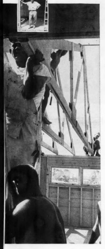
**INTERIOR PARTITIONS** start with shoe nailed to slab on chalk lines. Cut at same time are a second shoe, of one inch stock, and top plate. Heavy paper is used to protect the finished floor.
