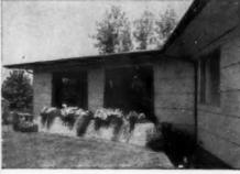
Wide-lapped siding made by ripping panels in half or thirds has unusual "scale." Use standard PlyShield grade or, for smoother, more durable paint finishes, overlaid plywood.
