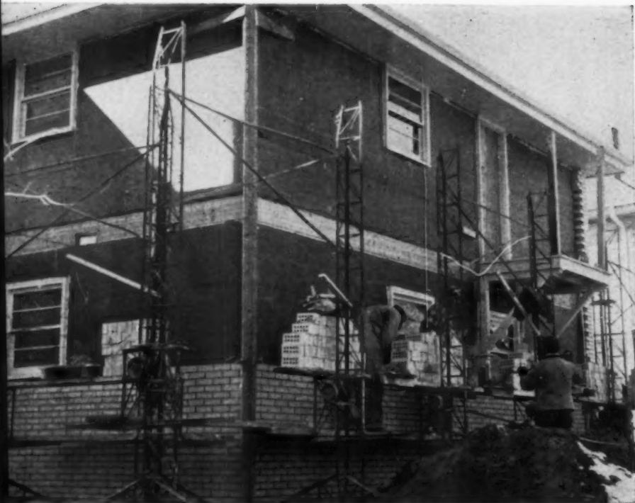
With this new self-elevating scaffold . . .
