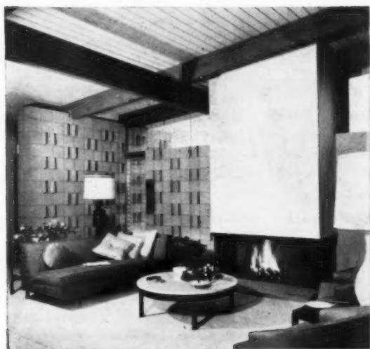
BUILT-IN PLANTER flanks large fireplace with raised hearth. "Outdoors" is carried inside by extending masonry wall to form divider between foyer and living room.
