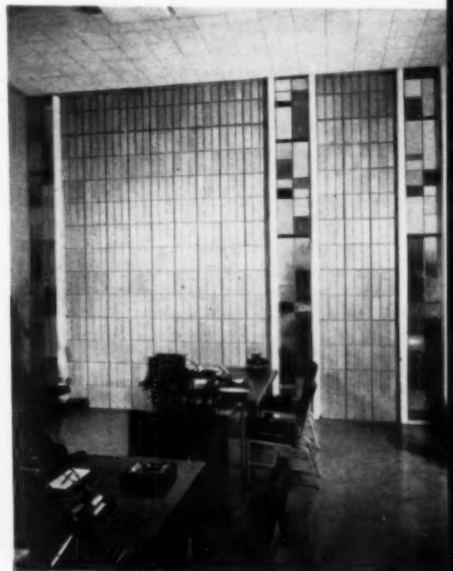
THEME of design is carried inside with effectiveness. Brick on the interior breaks up monotony of plain wall, and also provides an easily maintained surface.
