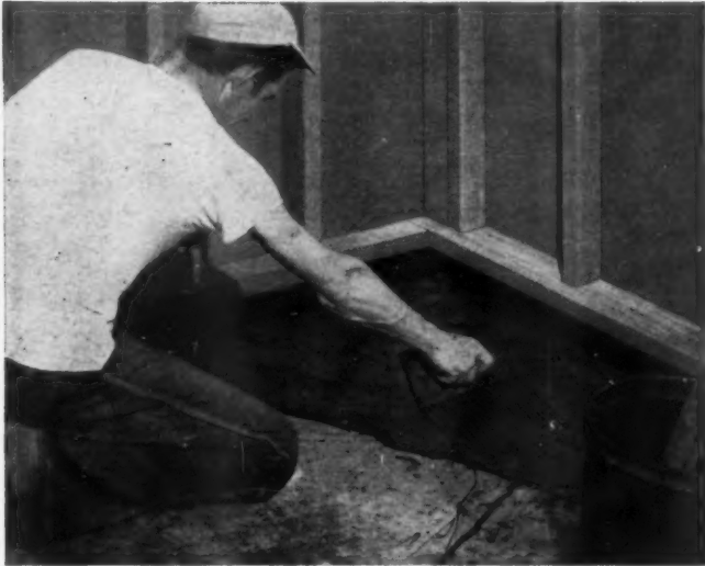
① Spread mastic over waterproofed slab.
