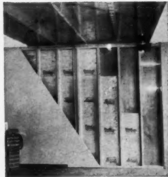
INSULATION , studs, and ceiling structure are shown by cutaway section of living room wall. Not shown: aluminum window display.
