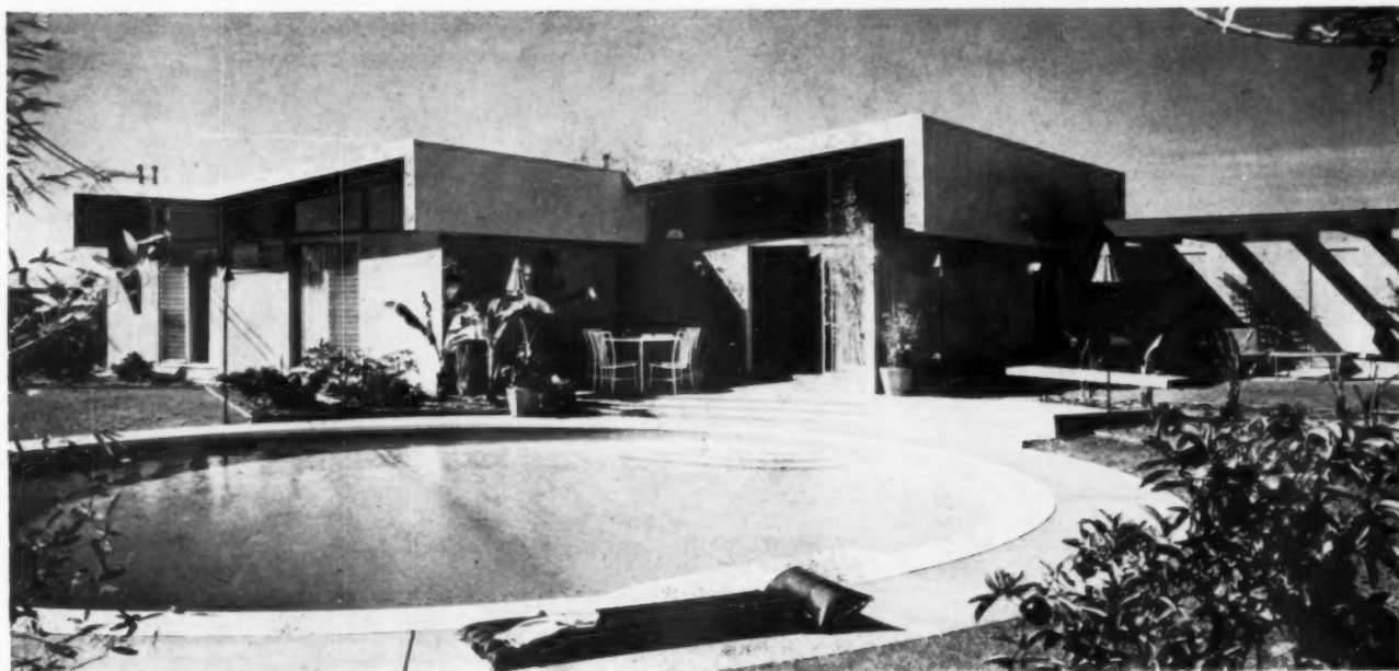
WIDE OVERHANGS and "lap-ear" fascias of the roof provide efficient sun-control.
