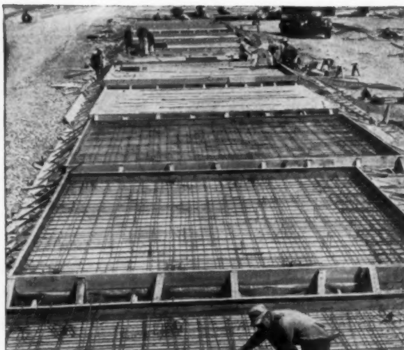
UNDER SLABS—VISQUEEN film keeps moisture out—assures warm dry floors—for life of building!
