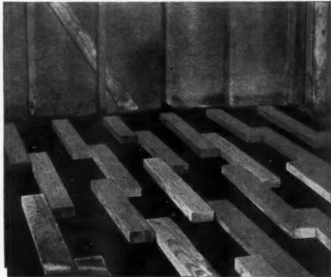
② Lay 2x4 screeds in staggered pattern.
