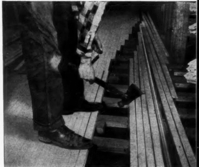
③ Nail Oak Flooring strips to screeds.
