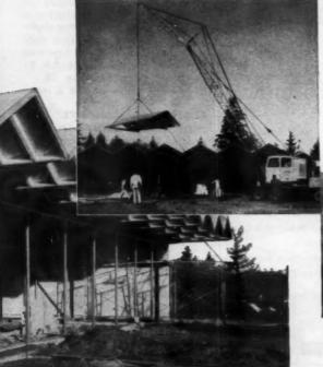
Fir plywood folded plate components were built on ground, crane-lifted into position in pairs. Heaviest lift was about 1,000 lbs. Contractor was impressed with the ease with which his crew assembled and erected sections.
