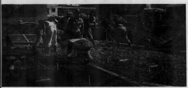
SIX-INCH LAYER of washed gravel is spread over the uncompacted backfill in this foundation. Note hilly site, the reason why so much cutting and filling are necessary in this area.
