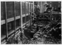
**EXCLUSIVE FLUSH-DIGGING!** Entire most and boom assembly shifts from center to either side for flush digging alongside buildings, fences, by trees, and other obstructions. Only Davis offers this advanced featurel
