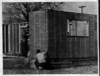
MEN SIMPLY BOLT each masonry component securely to the next. The finished wall has double studs every 4'. These, with 4x4's at each corner, provide strong frame construction.
