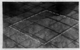
**DOTTED LINE** indicates pier position. Mesh must be lifted an inch off barrier as the concrete is poured.
