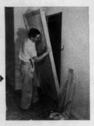
IDEA . . . in the near future perhaps you'll mechanize with a brick panel. SCPI has a panel out, one brick in width, that's designed to be a 2½" thick bearing wall with stacked joints. Speeds up, simplifies construction. See Feb. '58 American Builder, p 206, or (No. Z3, p. 114)
