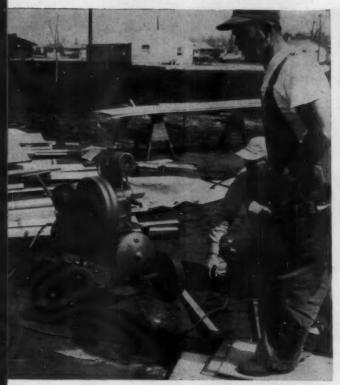
66This is the compressor end of our compressorpneumatic stapler rig. The stapler drives a divergent point staple up to about 1½" long, and it has tremendous holding power. 99
