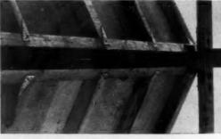
HALF-INCH bolts drew up pairs of panels forming valleys. 56" Fir Plywood, 5'6"x4', was nailed to frame of 3x4's, alternating with 2x4's on 2' centers.
