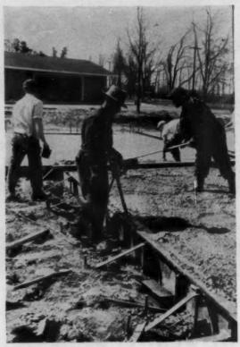
66We find an electric vibrator saves time by floating out the water more quickly. Also it compacts better. We can use a stiffer mixture, which is stronger, and less cement, which is cheaper.
