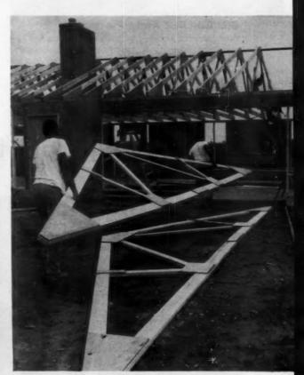
66A 34' truss is practically as easy to handle as a 32-footer. And if you take advantage of all its possibilities, a truss can save you better than \$1,000 a house over conventional framing.
