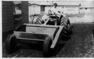
SMALL PAN, or scraper, is easily maneuverable, handy for use between houses. It can grade, carry away dirt, or cart it in to fill low spots. And in a pinch, it can truck blocks, bricks, or kegs of nails.
