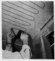
MANY RADIANT heating systems are on market today: electric, hot air, hot water. This is Goodrich's vinyl electric compound. (No. Z31, p. 114.)
