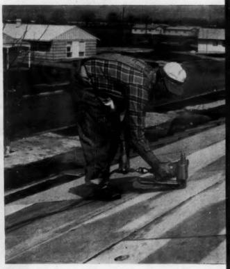
66One man with a stapling gun can keep up with two men laying and tacking down roof sheathing. We can do the whole roof in four hours. The only problem is loading the gun fast enough. ● ●
