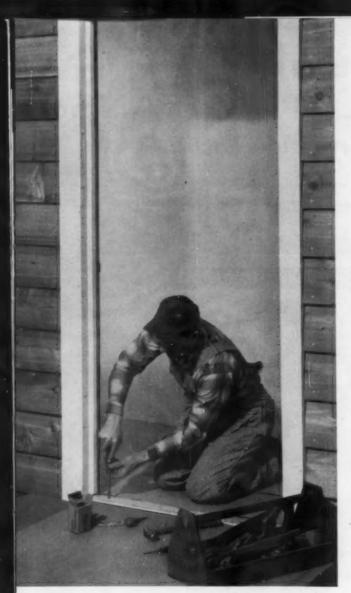
Easy-t0-use corrosion-resistant nails of Alcoa Aluminum reduce labor costs by eliminating time-consuming countersinking and puttying. They drive easily—are etched to hold tightly.
