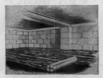
In busementless homes, the simple, low-cost way to protect crawl space is to spread DURETHENE polyethylene film on the ground and then cover it with a heavy layer of dirt. This provides a permanent moisture barrier and prevents serious dry-rot damage to plates, sills, joists and sub-flooring.
