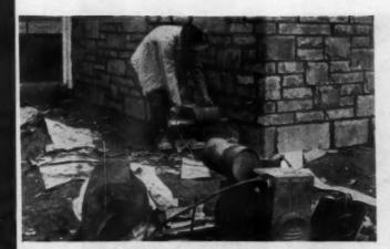
**INVESTMENT** in highly specialized tools is justified when there is high volume. This mortar gun follows the machine in the picture at left, does the job far faster than would be possible by hand.
