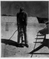
IDEA . . . Three nails a second is the record for this electric nailer. Speeds, by three to five times, nailing of subflooring, roof sheathing, trusses. This one, from B & H Homes. (No. Z11, p. 114.)
