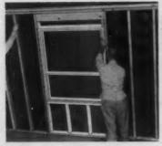
IDEA... Faster framing, done with the help of a Structural Windowall from Andersen. Whole window component is joined to adjacent framing, then tilted up with wall. (Circle No. Z1, p. 114.)
