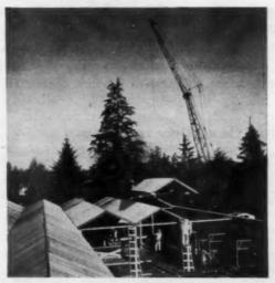
CRANE lifted pairs of panels for the first five bays in 105 minutes. Rest of the bays, after they were completed on ground were erected in 7 hours.
