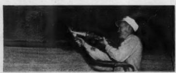
**IDEA** . . . Anything from thick plaster to thin paint can be applied with some type of pneumatic spray gun. Results: a more professional job, by fewer men, in fewer working hours.
