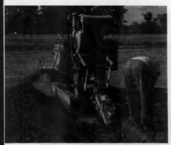
€€We use this trencher mostly for digging foundations. Two men can do a 2,000 sq. ft. house in an hour and a half. The trenches are exactly 8" wide, so we don't waste concrete. 99
