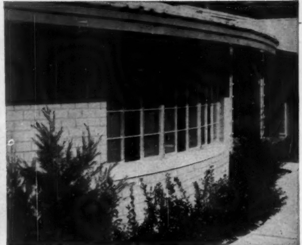
Painted 4"-high units. Another of concrete masonry's many new forms
