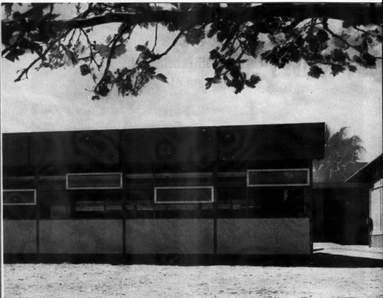
New addition by Calcor Corp. to Cathedral City Elementary School (Palm Springs Unified School District), California
