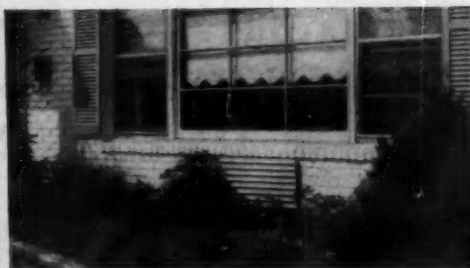
OUTSIDE , the Built-in Thinline has a "no-see-through" aluminum grille. It can be painted to match exterior. From street, it has a neat, built-in look.
