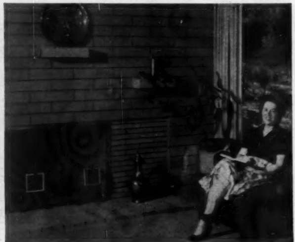
Raked horizontal joints add dramatic shadow lines to fireplace
