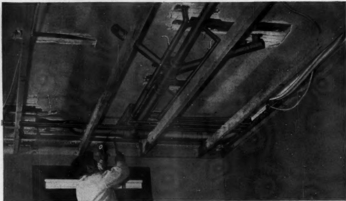
COPPER TUBE made light, fast work of an otherwise tough, slow job of roughing-in for two new baths on the second floor of a large old single-family house which was renovated to make several apartments.
