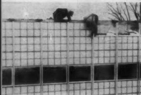
IN PLACE , panels are finished with pre-cut, pre-drilled head members. Neoprene gaskets form weatherproof seal.
