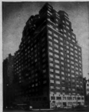
This 19-story penthouse and luxury apartment residence at 50 E. 79th St., N.Y.C., built by Fisher Brothers, features Textolite surfaced cabinets in every kitchen.
