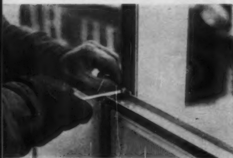
FASTENING panels to struts. It's done with stainless-steel bolt and clip assembly. (See diagram, at right.)
