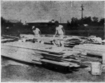
EXTERIOR TRIM is pre-primed and back-primed at shop or nearby. Quality lumber used.
