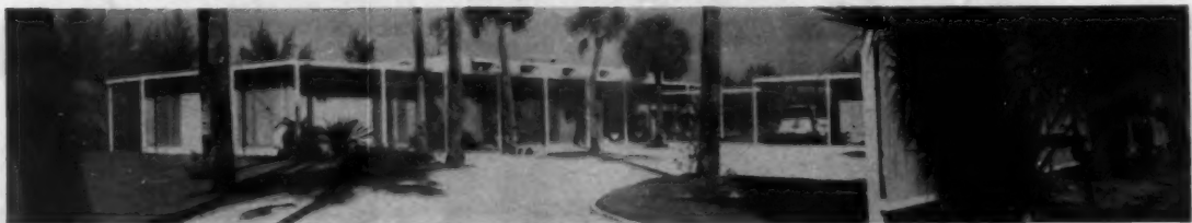
SLEEK, low house is encased in glass. It's located in Sarasota, Fla. Architect: Paul Rudolph.
