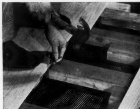
Over concrete, install Strip Oak Flooring this low-cost way... on screeds imbedded in mastic.
