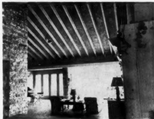
Acoustical ceiling of Cemex in the Dr. Kent Barber home in Quincy, Illinois (architect, Charles F. Behrensmeyer) is highly decorative and helps equalize Midwest temperature extremes.
