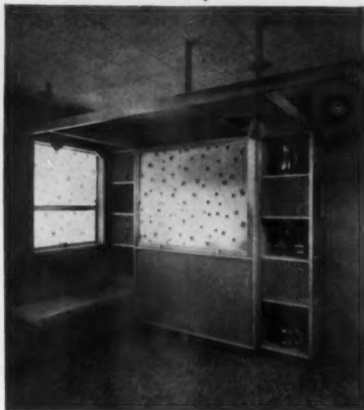
SOFT-DRINK BAR: plastic bar is raised to provide access to bar; plumbing and storage space are below. Drawing illustrates how hardboard panels slide in grooves. Counter top of 3/4" plywood is cut out for sink.
