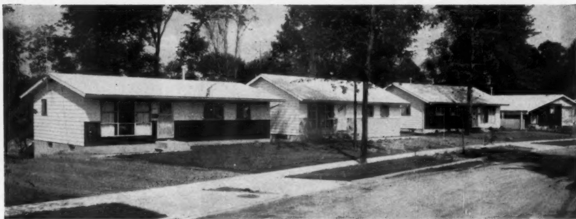
AlSCO siding used exclusively in this 85 home development by N & S Builders, Inc., Massillon, Ohio.
