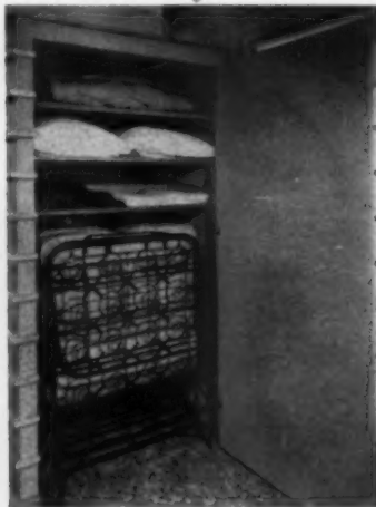
BED & LINEN CLOSET UNIQUE CLOSET: folding bed (as well as linen) fits into this "divider" of 3/4" hardboard. Framing members on outside are decorative, give extra inside space.
