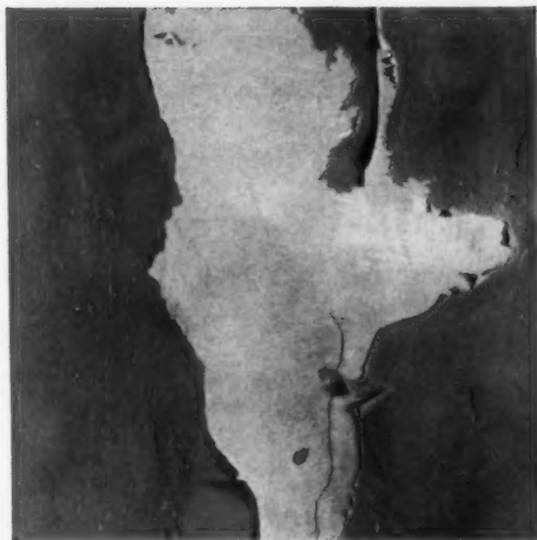
PEELING AND FLAKING of interior paints caused by moisture absorption through exterior walls.
