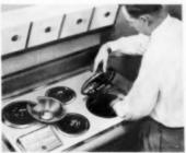
Six thumb screws to tighten . . . one conduit to connect . . . done! Oven and cooktop installed by The Eagles Co., Louisville, in less than 32 minutes.
