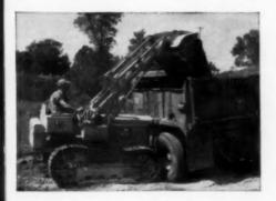
The Oliver OC-46 is the integrated, heavy-duty %-yd. loader—engineered and built as a single unit. Compact design eases close-quarter work. Long, 46"-wide tracks assure stability. Design provides a high dump, a long reach. Gas or diesel power.
