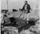
3.  $1\frac{1}{2}$  to 2 hours after screeding, Stow G-42 Roto-Trowel used to float and finish floors.
