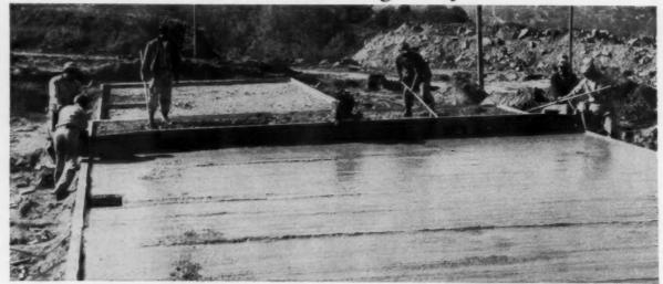
1. Making first pass with 24 ft. 8 in. Stew vibrating screed. 16 man hours per slab saved by Major Building Co.
