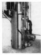
Typical spacesaving B&G Hydro-Flo System heating plant. The boiler has a built-in water heater.
