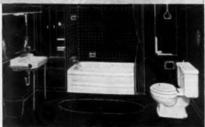
Bermuda Detuxe Bathroom, designed and built for The Mighty Middle. Gerber packaged bathroom No. 2. Ledgetype lavatory, No. 380, 20" x 18", has centerset with aerator and pop-up drain, No. 143A. Closet is deluxe unit-type, reverse trap, 12" rough-in, No. 1200. Porcelain enameled steel recessed tub, No. 05, with 3-valve bath and shower diverter, No. E4802, and trip lever drain, No. 181G.
