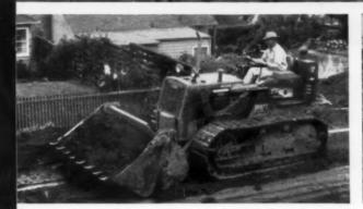
**He can grade with accuracy** using 4-in-1 "carry-type scraper" action to let the dirt boil in. With this same action he can strip sod; skim-off layers of materials. And he can regulate clam lip opening to spread materials precisely!
