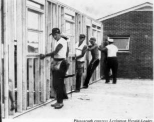
Photograph countesy Lexington Herald-Leader. Saves time, materials I To install Strutwall, Fister-Seeberger workmen simply cut two load-bearing side struts to fit header construction. Nail in place. Tilt up with wall. In multiple openings, Strutwalls are butted against each other. This eliminates need for anything heavier than two 2 x 6 headers in single story construction.
