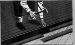
Simplest of all floors to install, Oak is nailed to subfloor in wood joist construction. Modern Strip Oak Floors are precision manufactured in a variety of sizes and grades to suit any building requirement.
