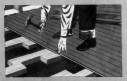
Screeds laid in mastic provide nailing surface for installing Strip Oak Floors in homes built on concrete slabs. Write National Oak Flooring Manufacturers' Association for free installation manual.
