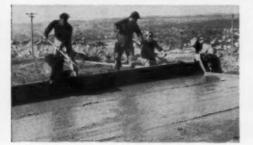
2. 4-inch slump concrete is screeded. Note the termite shield at edge of slab.
