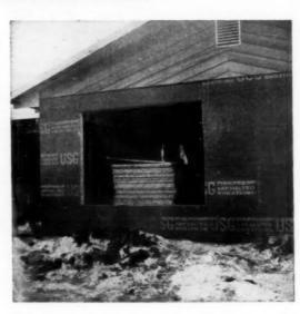
Three man hours per house are saved by putting gypsum wallboard into the house through the rough opening for the picture window. Back filling is carried to wall, truck backs right up to the window.
