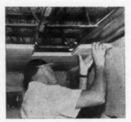
**3.** Tiles are interlocking. They are supported at corners by splines fitted into the tile kerf.
