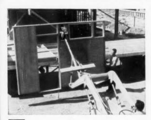
Prefabricated plywood wall panels used for a 50-room motel job in Palo Alto helped Contractor Don Gordon build five buildings in less than 100 days at a cost of less than \$9 psf. The fir plywood components were assembled in jigs and trucked to the job site where they were boom-lifted into position.
