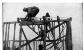
Trusses are positioned and spiked down by a threeman crew on top of the house. To hold the trusses upright in precise position until the roof decking goes on, Stream uses a variation on normal procedure. In-
