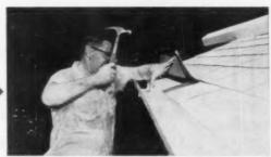
MOLDED-IN FLASHING fits under the roof shingles, and gutter is nailed right to the roof edge. Putting up flashing and gutter in a single operation saves job time, helps prevent ice damage.
