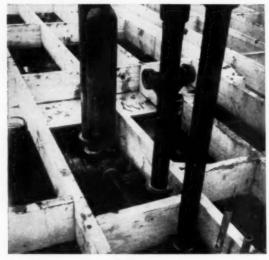
of the foundation. Supporting piers for this girder are poured in paper Deltaforms. Finished floor framing (above) is built around tree, a much cheaper procedure than building pipe around the framing.
