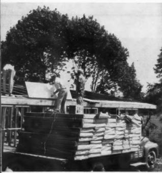
Decking comes in light-weight bundles, can be easily lifted up to roof level. Here it is unloaded directly from truck. To avoid dirtying finished ceiling, workmen should wear gloves or cover their hands with talcum powder when handling unwrapped slabs. (Until it's used, decking must be kept dry and protected from damage.)
