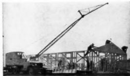
Prebuilt gable end is lifted into place by mobile crane. Stream owns this machine (which converted from a backhoe); the smaller builder, who couldn't afford to buy such heavy equipment, might rent a
