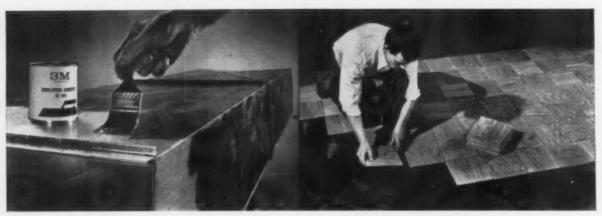
UNUSUALLY HIGH COVERAGE. Insulation adhesive EC-104 covers up to 200 square feet per gallon when brush applied. Goes on quickly, easily, uniformly. Provides fast grip even when wet. Open time: up to 20 minutes when both surfaces are coated.
