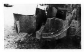
This device saves 2½ to 3 man hours per house. It sweeps loose dirt back into the ditch, to be picked up by the bottom digging buckets. This cleans top of the ditch, eliminates clearing the trench with
