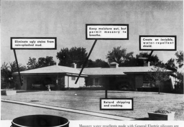
Masonry water repellents made with General Electric silicones are quick and easy to apply. They penetrate deep into the capillary pores of masonry, forming an invisible water-repellent shield. This eliminates those ugly stains caused by rain-splashed mud or by dust and dirt on the masonry surface. Rain runs right off, carrying dirt with it. But that's just the beginning! Silicone water repellents help pre-
