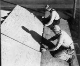
The combination of PlyScord and Plyclips is credited with making possible a 50 per cent labor savings on this 31-building New Hampshire public housing project. Over 160,000 sq. ft. of plywood was used for both wall and roof sheathing.
