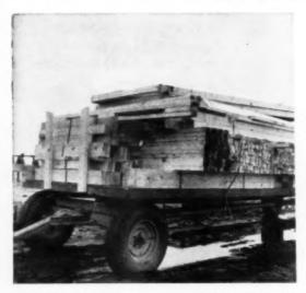
Praming is precut and color-coded to reduce site labor, eliminate guesswork in selecting the right piece. It is packed in steel-strapped bundles (trusses are put into special frames). A crane lifts the bundles
