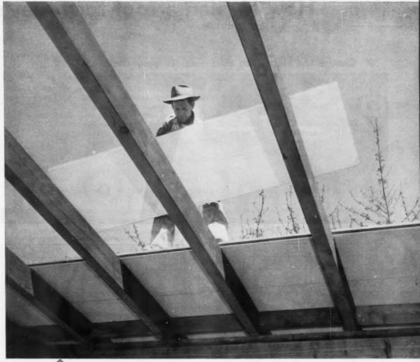
**EASY INSTALLATION** means reduced construction time. Sections are either interlocking or tongue-in-groove. Carpenter merely pushes them together, nails them directly to the roof timbers. Insulating roof-deck slab marks a big step toward using more completely finished building components.
