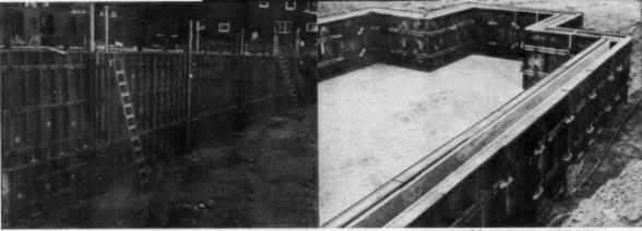
Rocform Systems are easily adapted to any type of forming job. Absolutely no alterations to the standard Rocform panels are ever necessary to form any type angular wall.
