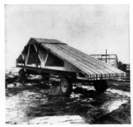
onto trailers for shipping to the site. Stream uses Jeephauled David Bradley (Sears, Roebuck & Co.) farm trailers. They are adjustable lengthwise, but Stream fixes their length by welding and bracing.
