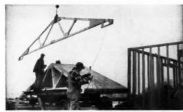
Photo shows a truss being lifted from the trailer.
