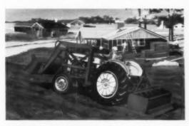
GRADING AND LEVELING—Down-shift in a wink without loss of forward motion when you hit tough spots. As the load eases, shift up again for more speed, more fuel economy. Pull high spots into low ones with quick shuttle-type passes. Use Ford's low, low speeds for more "push" when needed, and for smooth, uniform finish work.
