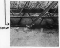
1. Galvanized-steel main runners are attached by means of steel clips to the undersides of steel joists.
