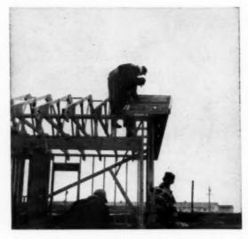
above show the component being installed. Gable end is built 3% in. lower than trusses. Ladder section is run out from truss over the gable end, and is spiked to the rafters of the second truss,
