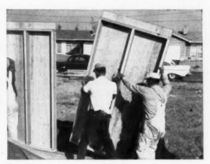
Panelized plywood wall sections permit three workers to erect walls in only 90 minutes on Lu-Re-Co homes built by Hebb & Narodick, Seattle. Components (including trusses and plywood sheathed gable ends) are credited by construction foreman with saving as much as \$300 per house in labor costs alone.
