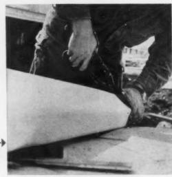
GUTTER SECTIONS are cut to proper length with tinsnips, as shown, or with a saw. Spout holes are located, then cut, using a template supplied with the kit. System is now ready for installation.
