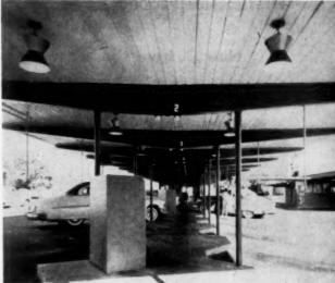
SIMPLICITY OF CONSTRUCTION is shown in this close-up of car shelter. Timber-framed canopy was used instead of metal because of lower costs, easy maintenance. Covered walk at right of photo leads to restaurant building. It took less than a month to build this shelter.
