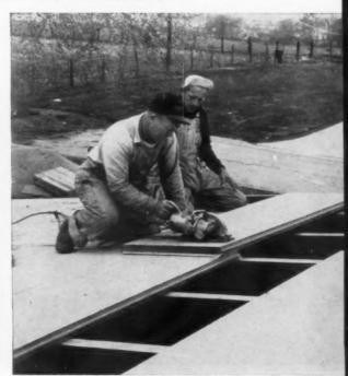
Insulating roof-deck slab is easily cut with a power or hand saw. But carpenters must take care to avoid roughing the edges of finished surfaces, should use fine-toothed blades. To minimize waste, roof should be accurately laid out beforehand. Of course, all joints must fall in the right place—over framing members.
