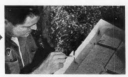
THE SECTIONS are overlapped, then joined with a bonding agent. A coupler is supplied for joining sawed lengths. After gutters are in place, drop outlets are bonded into the spout holes.
