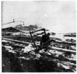
Stream cuts plumbing costs 20 per cent by having his plumbing trees prefabbed off site. Here a tree is being moved into position in a finished foundation. Note the single steel I-beam girder running the length
