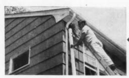
JOB NEARS COMPLETION. Elbow is attached to drop outlet, and the base section of the downspout is nailed to the house, as shown. Downspout snaps onto this base section, requires no bonding.
