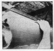
2. Splines snap into main runners, are centered to straddle tile joint. Each spline holds four tiles.
