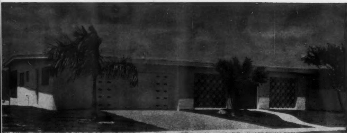
BRICK AND STUCCO EXTERIOR , red door of "Spanish" entry court create favorable first impression. "Lake-
