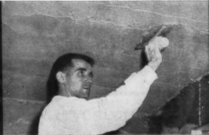
Plaster is applied over reinforced ceiling. The open mesh of both Keymesh and Keycorner assures imbedment in plaster. The open mesh also insures full bond of plaster with gypsum lath.
