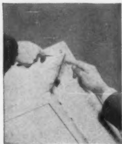
In joints of wood gutters
