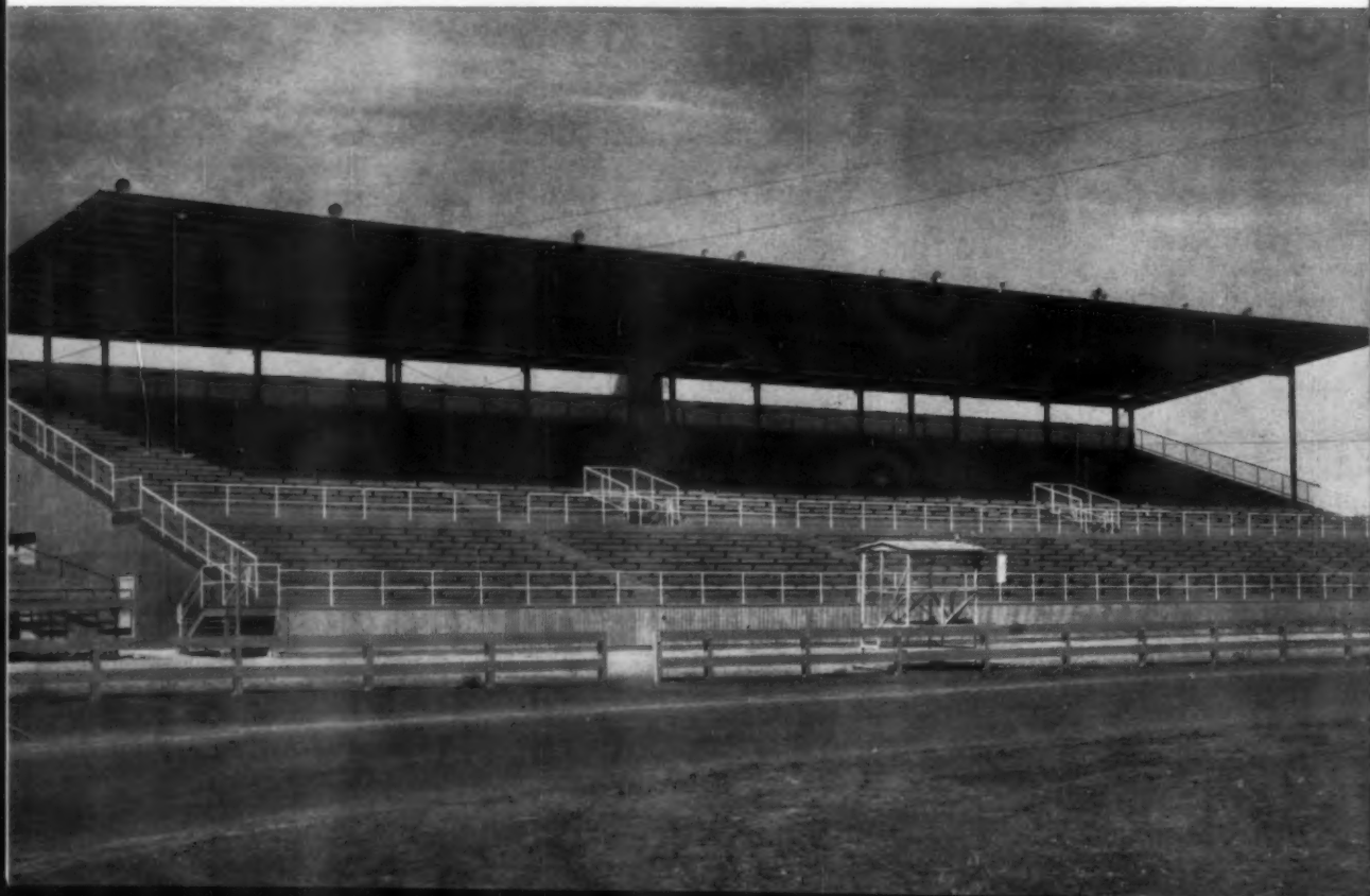
Minot State Fair grandstand, Minot, North Dakota. Fabricated with 92 tons of USS Structural steel and erected in 75 days. Owner: Ward County Fair Assn.; Architect & Engineer: Engineering Division, Arrowhead Engineers & Constructors, Duluth, Minn.; General Contractor: Central Steel Erection Co., Minot, N.D.; Fabricator: Fargo Foundry Co., Fargo, N.D.
