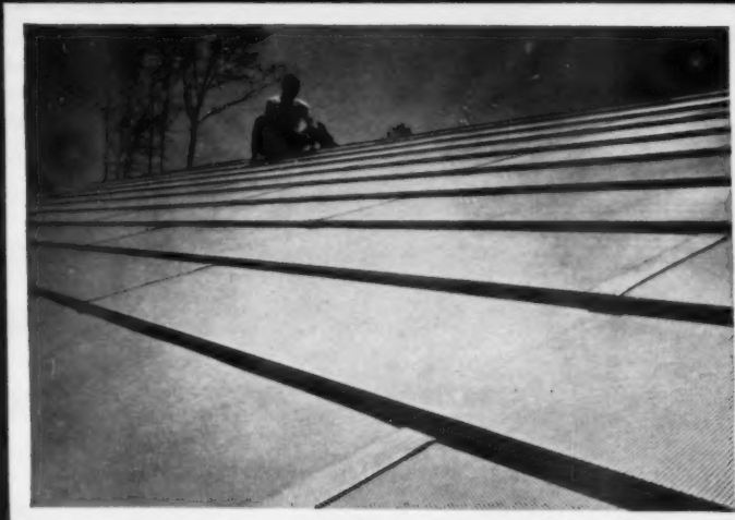
EXPERIMENTAL "BERMUDA ROOF" is made from 1/2-inch plywood panels, 8' by 16", covered with a prefinished skin of embossed aluminum. Panels can serve as both sheathing and finished roofing. Details of joints are shown in drawings. Kaiser Aluminum Co. designed roof, and products below.
