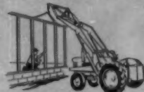
CRANE BOOM lifts partitions, sets forms, window units, bulky articles.
