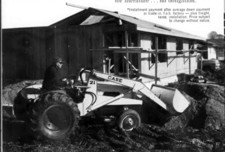
BACKHOE cuts trenches, footings to 10'.
