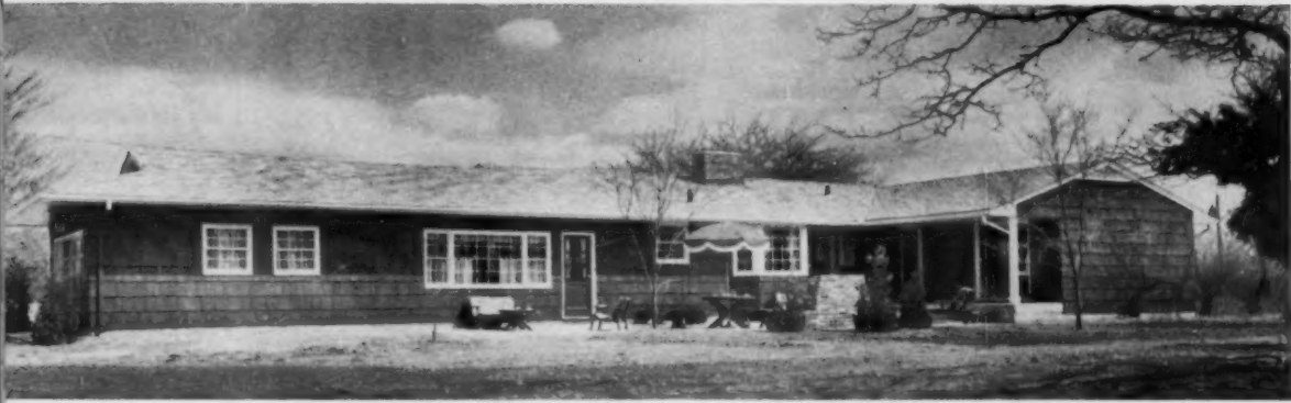
REAR VIEW of the "York" shows the terrace and fireplace, with bedroom porch at the far right.
