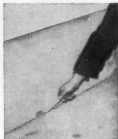
At sidewalk, foundation
