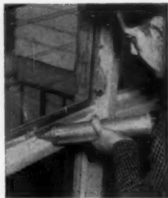
Around metal shutters
