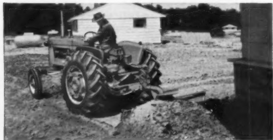
Backfilling a foundation.
