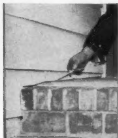
At siding and concrete
