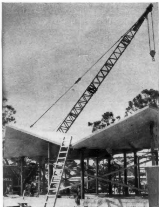
AFTER CURING —concrete attained strength of 3,750 p.s.i. at 28 days—sections were hoisted into place by crane. Weighing 88 tons, the roof is supported by 15 lally columns which rest on concrete pads (see drawings, left).
