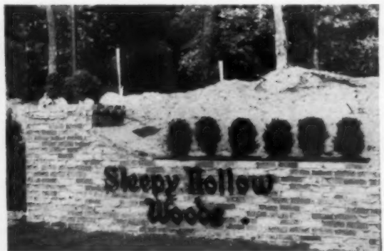
SIMPLE, BUT DIGNIFIED entrance to community consists of brick and shrubbery put up at little cost.
