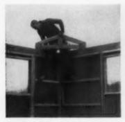
ENDS of first small truss are placed exactly 4 ft. from corner . . .
