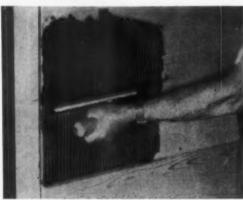
2 MORTAR IS GROOVED OUT. It must be spread as thin as the trowel notches will permit. The new material will bridge relatively deep hollows and still provide a firm tile bed.
