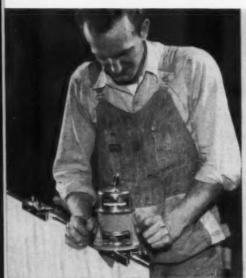
THE CARPENTER-SIZE ROUTER! This is one heavy-duty router designed with the carpenter in mind. Easy to handle. Light-weight—just slightly over 5 pounds. Full ½ hp motor has power to spare. 23,000 rpm spindle speed gives smoothest possible cuts on any routing job. Assures accurate, fast jamb mortising when used with new SKIL No. 17070 Hinge Butt-Template Kit shown.
