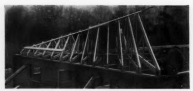
... HIP ROOF BEGINS to take shape as succeeding trusses are installed. Trusses are 2 ft. on centers, but are 2 ft. 10 in. apart along the plate.
