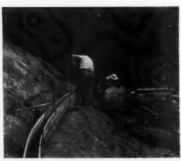
AT SITE, concrete is moved from the bucket into the forms for an interceptor ditch. Normally, the concrete is dumped directly into the forms, but in this case, the narrow space between boards made it necessary to transfer the material by shovel.
