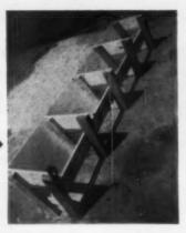
Bearing-wall beam is shaped with this form. Here, rods and vapor barrier are in place, awaiting concrete.
