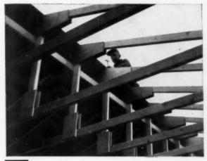
Fir plywood gusset plates are the surest and simplest way of fastening joint truss members together. Plywood provides greater rigidity, reduces deflection. It can be used for either nail or nail-glued construction. The trusses themselves eliminate load bearing partitions, take less time and material to build.
