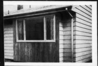
OUTSIDE, the bay fits snugly below existing roof overhang. Foundation didn't have to be altered, because the projection sits on cantilevered floor joists. Bay could be added to an existing structure very easily.
