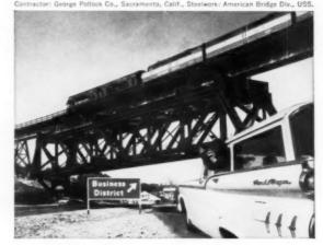
New Lift for Old Bridges. A revolutionary new construction idea—a "piggyback" bridge to carry an existing railroad bridge over heavily-traveled Highway 40 at Auburn, California. The new bridge of USS Structural Steel replaces supporting towers and provides a 240' span for uninterrupted traffic flow on the widened highway below.
