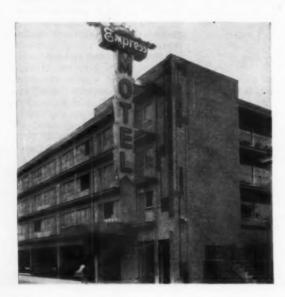
A luminum curtain-wall panels enabled the J & L Construction Co. to cut 50 per cent from the wall-erecting costs of this four-story Atlantic City motel. The panels were shipped to the site knocked down, merely had to be assembled and set on the job.
