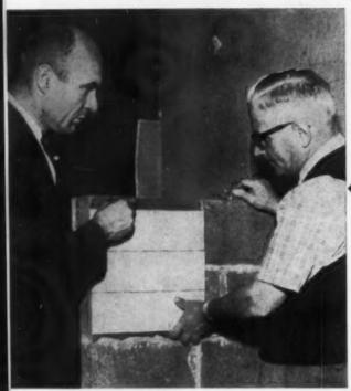
EVEN A ROUGH-SURFACED concrete block wall makes a good tile backing with new dry-curing, thinset mortar. Here editor Lou Volse learns how to use it from John Stefano, at TCA's research center.
