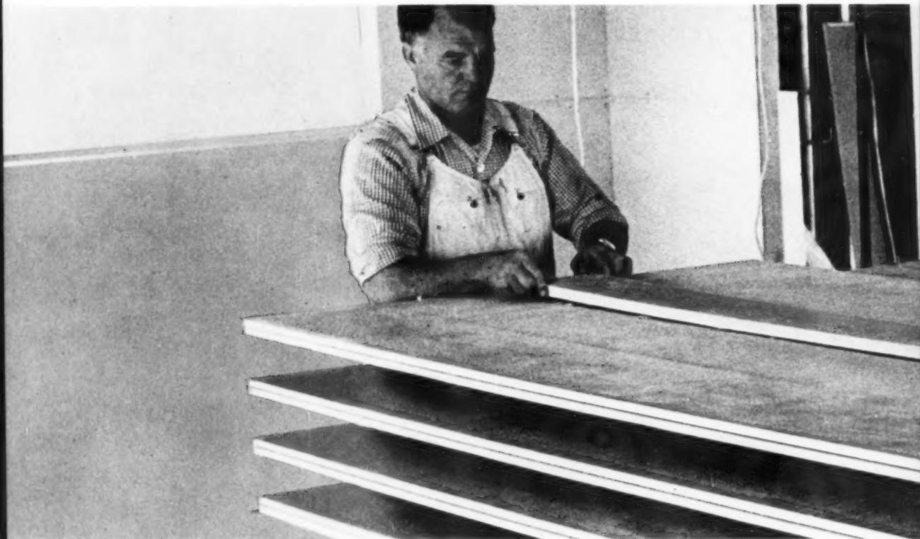
**1** First step is laminating strong 1" x 6" gypsum ribs to gypsum board panels. Ribs are attached on center with Pabco joint cement at a rate of one each 60 seconds. Total laminating time is 40 minutes on an average job.
