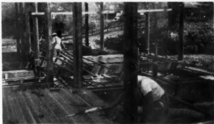
**FLOOR BEAMS** are bolted on both sides of poles. Ends overlap at center poles. Carpenter is shown laying 2x4's on edge, to form floor, which spans distance between beams.
