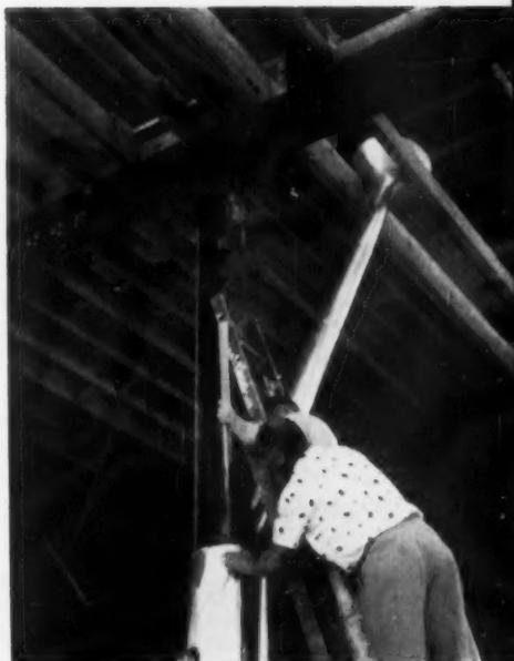
**TO PROTECT** steel columns from moisture at ground level, concrete is poured around them, into metal form, from top floor level of the house.
