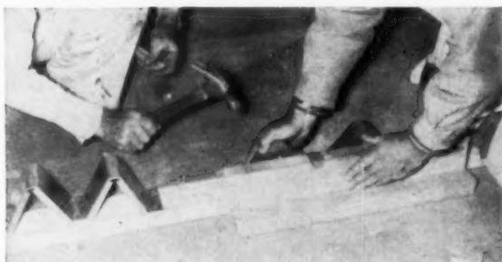
**2 ALUMINUM "W" FLOOR TRUSSES** are nailed to bottoms of 2x4 floor joists. One end is nailed, the other end moved until height is right. Then it too is nailed.
