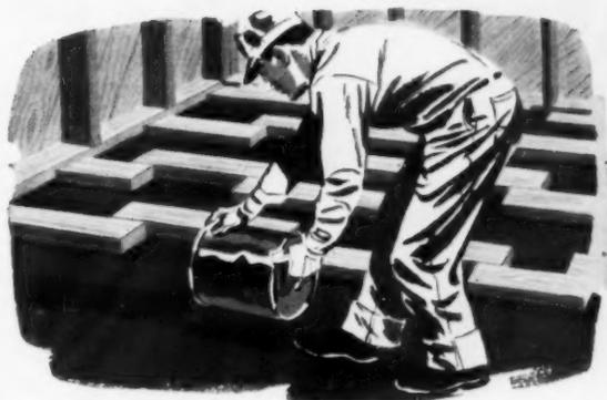
**1.** Apply surface moisture barrier to slab and lay flat, dry, preservative-treated 2 x 4 wood screeds in hot mastic. Use random length screeds, 18" to 30".
