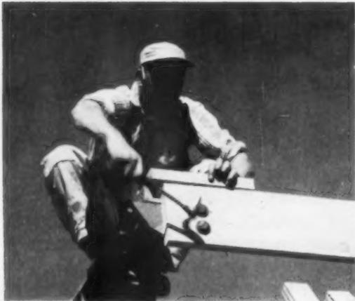
**STEEL FRAMES** have been drilled to receive wooden members. Wooden rafter section will support fascia.
