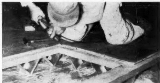
**6 COMBINED SUBFLOOR** and floor is laid on joists. It's a 7-ply plywood with finished flooring on top. Tongue-and-groove edges permit the blind nailing.
