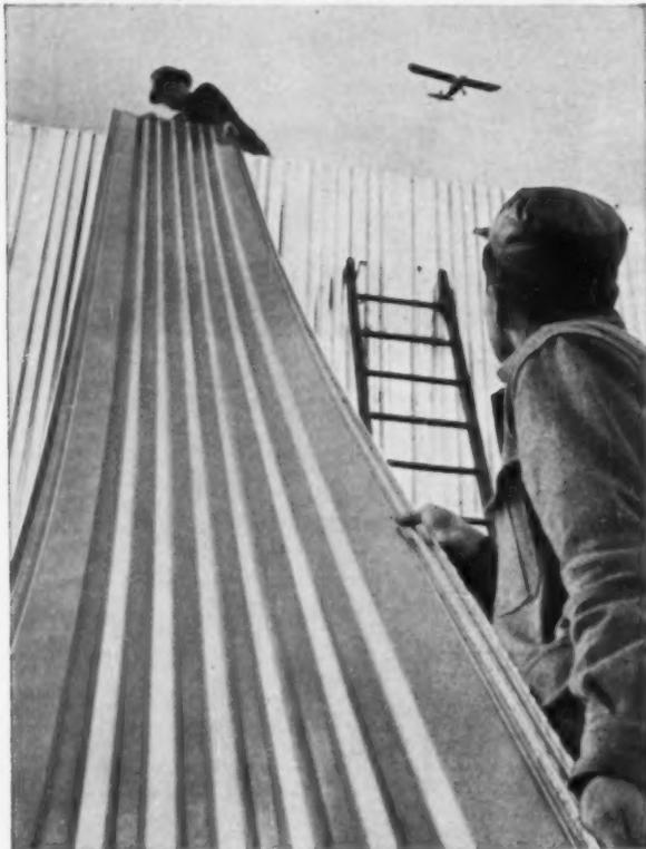
**New Ground Cover for Aircraft.** When storm warnings fly in northern Washington, all planes are secure in weather-proof steel hangers at Arlington Airport. These structures were built to last from USS Galvanized Sheets, formed into special long length panels by Western Aluminum Corp., Seattle. This new application of USS Sheets provides extra strength and saves money, through faster erection time and easier handling.
