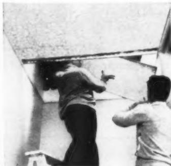
**PANELS** are installed by standard glazing techniques, framed or supported by molding. Material is strong, requires no special handling.
