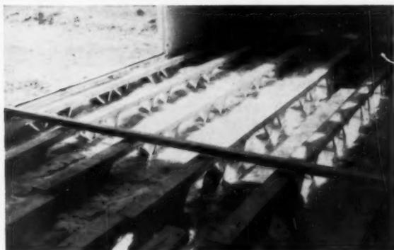
**FLOOR JOISTS**, with aluminum floor trusses nailed to them, turn slab foundation into a crawl-space foundation. Here, joists have been laid out and leveled. Strip in foreground is temporary brace to hold them until floor is laid.
