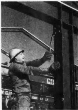
**ALL CONNECTIONS** were designed to be bolted with high-strength bolts and machine bolts. Here, workman tightens beam-to-column connection.
