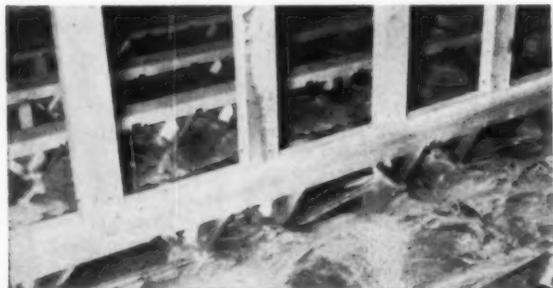
**3 PARTITIONS (ALL NON-LOADBEARING)** can be set before floor is in place. They must be laid out to fall over a floor joist, or a floor joist can be shifted.
