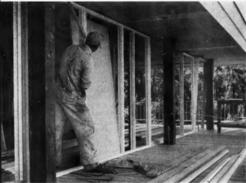
When the steelwork is finished, carpenters move onto the job to cover the house. The roof is 3x6 double tongue-and-groove roof deck, pre-drilled to receive long steel spikes driven laterally through the decking. Underside of decking forms ceilings throughout. Floor framing is conventional 2x10 joists. Decking is plywood with hardwood and resilient flooring. Exterior walls are weatherproof "Timblend" panels set in pre-fabricated redwood frames; stained panel surfaces are exposed on both sides.
