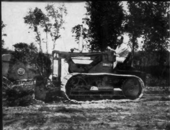
**It's a bulldozer** with exclusive "radius control" of dozing depth which allows you to bulldoze with inch-close accuracy.
