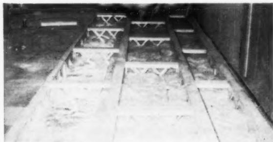
**5 BLOCKING STRIPS**, also with trusses attached, are staggered between joists. They're set on 48-in. centers. Joists go on 24-in. centers for special flooring.
