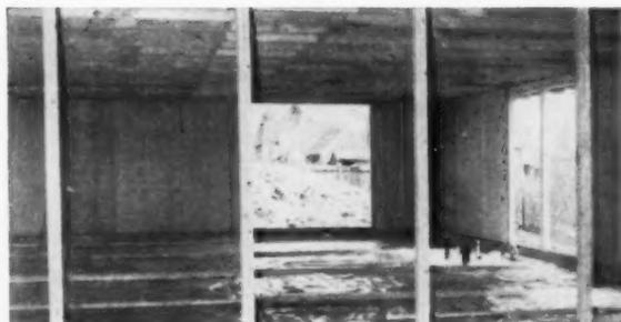
**1 ALUMINUM FOIL** is laid down as both insulation and extra vapor barrier. Perimeter of blanket insulation goes over the foil, to insure a warm floor.
