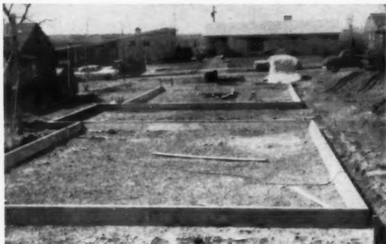
**GRADE BEAM HAS BEEN POURED** and house is ready for slab. Slab will be set low enough so that finished floor will eventually wind up level with top of grade beam. Slot between floor and beam is the warm-air register.
