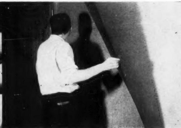
**QUICK GRIP.** ROLITITE® brand contact cement bonds decorative laminates to walls at a touch. No nails or clips needed. No nail holes to fill. Simply coat both surfaces, let dry and hand roll laminate into position. Highly water resistant, it prevents warping or peeling.
