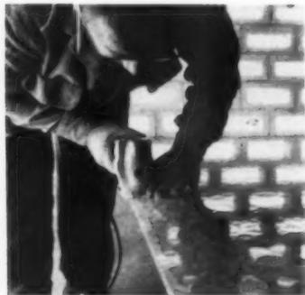
**ELECTRIC SAW** is used at job site to cut Tropiciel to proper size. Panel edges are then taped to prevent dust penetration.
