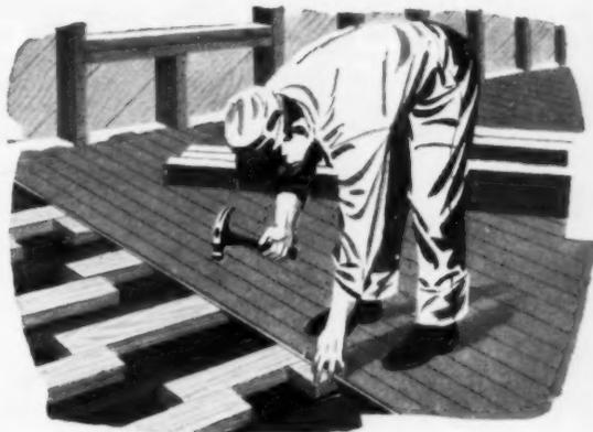
**3.** Blind nail tongued-and-grooved, end-matched Strip Oak Flooring at each screed intersection. Double-nail at lapped screeds. Finished floor is beautiful and durable.
