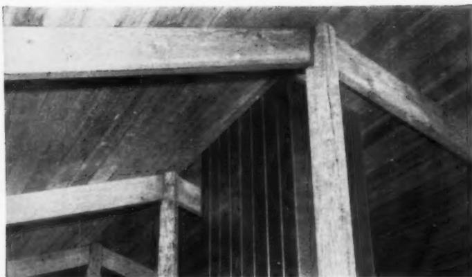
**RAFTER ENDS** butt into slotted center poles at the ridge. Metal straps screwed to top edges of rafters hold ends firmly in place. The decorative cover surrounds chimney flues.
