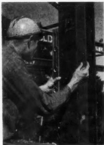
**IRON WORKER** plumbs column with a level. A simple turn of footing bolts, which fasten column to concrete footing, adjusts for plumb.
