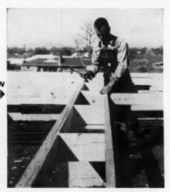
JOISTS ARE NAILED to girder, a faster operation than putting in bridging over a crawl space. To avoid cutting the plywood subfloor, 1x4 nailers are placed inside the girders.
