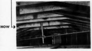
ATTIC VIEW of Lakeview house. Complete antenna is installed here without taking up too much space. Indoor installation performs as efficiently as outdoor, is free from damaging wind and rain.
