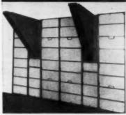
Designed both for residential construction and industrial where a wing wall is required. Forms concrete bracket four feet deep, and extends four feet from wall at top. Eight inches thick at wall, and six inches at outer extremity. Used with woodply or steel-ply forms. Handles provided for easy handling.
