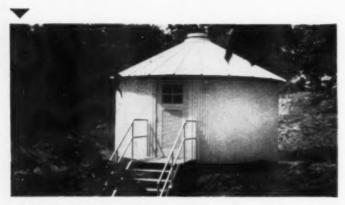
**COMPACTNESS** is a major advantage of the small treatment plant. This housing is all the cover necessary for Dorr-Oliver's 15,000-gallon Comple-Treator unit. The installation is for a small military base.
