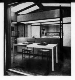
Home is built on three-foot module with four roof heights. Highest is over the living room.
