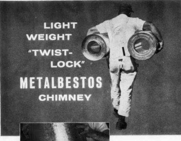
Simple "twist-lock" — like putting the lid on a pickle jar (no mastic, cement or screws). Perfectly safe for all fuels and incinerators (listed by Underwriters' Laboratories, Inc.). Finest materials and construction throughout assure lasting performance. Write to Department L-9 for our new METALBESTOS factory built chimney catalog MC-2.
