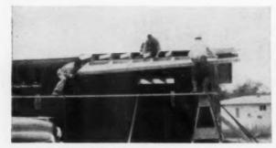
**SOFFIT OVERHANG** is lifted into place by two men. Man on the roof nails the component to walls and truss outlookers. To get maximum efficiency, soffit panels are completed for both sides, and are then installed in one operation.
