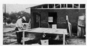
FIRST STEP IS LAYOUT. Precut members (these are for a soffit assembly) are placed on the trailer jig. Bed of the trailer is marked off in 8-in. increments, for 8- 16- or 24-in. centering. This helps minimize measuring errors.
