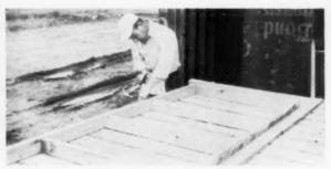
**SECOND STEP IS NAILING.** 2x4 members are placed over approximate mark and nailed up. Note 2x4 backing on trailer bed. It permits one man to nail panels against it. Also note how trailer's height permits man to work without bending over.
