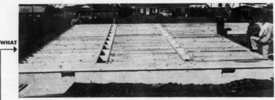
FINISHED FLOOR FRAME is shown above. Girders support three rows of 2x6 joists, which replace the two rows of 2x10 joists normally used. Girders also eliminate the two rows of bridging normally required.
