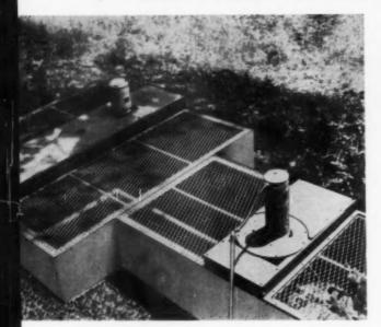
Y eomans "Cavitator" treatment plant, shown at left and in drawing below, is a packaged unit that will serve from five houses up. It is a super aeration type, in which large quantities of air are forced through the sewage to speed up reduction. Yeomans Brothers Company manufacture both the Cavitator and the Cavitette, a single-house treatment plant that operates on the same principle as the Cavitator. (Circle No. S127, p. 164)
