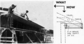
FINISHING OF THE CORNICE now involves merely finishing the roof over it. In photo above, one man uses a power hand saw to trim edge of sheathing along soffit. Man nearest the camera is feeding the saw's electric cord.
