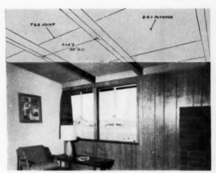
2.4.1 Roof decking is basically a modification of the floor system. Panels serve as both roof sheathing and finish ceiling. Panel edges between beams are tongue and grooved, with eased edges. As with subflooring, the in-place cost of plywood construction comes to \$100 less than car decking; material costs are the same, but plywood can be installed in half the time.
