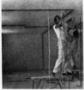
NAILING STRIPS, 1"x1½", are applied to ceilings, floors and sidewalls. Walls are laid out according to blueprint with chalk line and level. Note how interior framing is eliminated.
