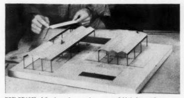
BOX BEAMS of fir plywood are used to support folded-plate roof.
