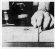
1. HERE'S HOW FAR nail goes through 2x4 into concrete.
