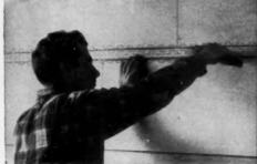
KEYSTRIP can be used as a reinforcement for plaster in a space too narrow for strips of gypsum lath. A full bond of Keystrip to the plaster is assured. Keystrip also adds strength to points of stress above doors and windows.
