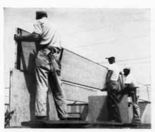
Plywood box beams act as the main roof support, have 3/8" fir plywood skins nail-glued to 2 x 4 top and bottom chords and stiffeners. Projecting (or recessed) end stiffeners form tongue and groove joints over bearing partitions. Advantages of fir plywood box beams include high strength-weight ratio, design freedom, dimensional stability, easy-to-finish surfaces.
