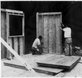
LURECO COMPONENTS go together rapidly to form the shell. Detailed, expensive work, like window framing, is done at the lumber yard.
