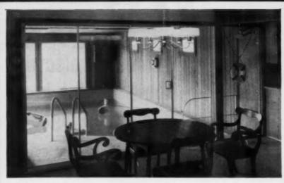
**SWIMMING POOL WING** opens off the living-dining room, is separated from it by a set of sliding doors. Pool itself is extremely simple, consists of a concrete block foundation, with a slab below. A standard plastic pool lining makes the whole thing watertight. House sold for \$24,500 with pool, but without land.
