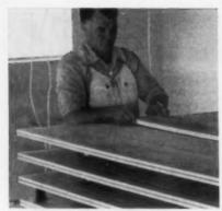
LAMINATE strong 1" x 6" gypsum ribs to gypsum board panels. Ribs are attached on center with Pabco joint cement at a rate of one each 60 seconds. Total laminating time is only 40 minutes on average job.
