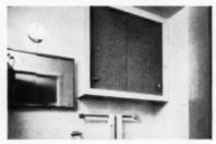
Bathrooms. Sliding doors made of Punched Sandalwood not only add a decorative effect but also offer the advantage of ventilation. It is temper treated for moisture resistance.
