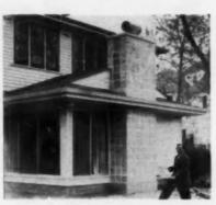
STACKED BOND construction gives the chimney an attractive pattern. Builder Gilhorn, at right, checks the completed job.
