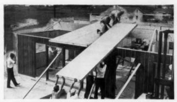
IN THE OFFING: foam core panels with stressed plywood skin to make a wall Plywood box beams and stressed-skin panels form roof.
