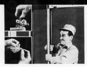
All-steel strength; easier installation, adjustment; 900 FA pocket Kennaframe—Warp-proof frame with a new ratchet type hanger permits door adjustment anytime without removing stops or trim. Only finger-tip pressure on this adjustable hanger is needed to insure perfect alignment. Shipped to fit your exact size specifications. Has removable track and nailing strips in place, ready for faster, easier assembly. Doors are held in place by simple retainer lock that disengages with pencil tip pressure.
