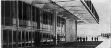
New Space for Cadets. Biggest job of its kind—the new cadet dining hall at United States Air Force Academy, Colorado Springs. Capacity: 3,000 hungry men. The roof is a 2-acre grid of USS Steel, floating on sixteen slender columns. And inside, a massive coffered ceiling is finished in gleaming USS Stainless Steel for permanent beauty and easy maintenance.
