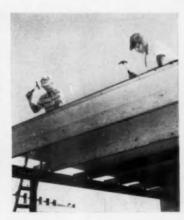
7. 45 min. to install panels and a layer of felt
