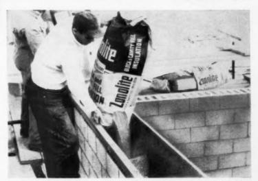
INSULATION NEWS: a masonry fill that makes it easy to pour insulation into cavity walls. From Zonolite. (No. 077, p. 166). Next page has more details.
