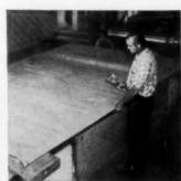
vapor barrier in sidewalls in a quarter hour. This was a onehour chore with hammer and nails. At an average of 10 panels per house, builder puts an additional \$16.88 in the profit column on each house.
