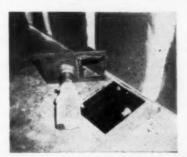
SEWAGE PLANT in miniature. One part: grinder installed below toilet.
