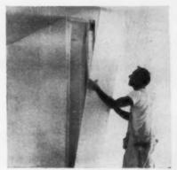
WIRING IS SIMPLE, with conduit coming through ceiling nailing strips and running between face panels to outlets. Note the strong outside corner achieved with 1" x 1½" wood strip.
