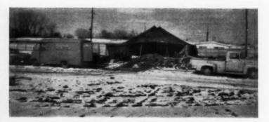
1. Jan. 1st: heated tent is used to thaw ground for a new foundation
