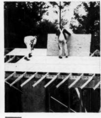
14 Kingpost trusses eliminate load bearing partitions, save 16 man hours per house. Two men take less than 4 hours to install the 24 trusses used on each house. Nail-glued fir plywood gusset plates fasten truss members securely... provide added
