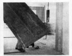
PANELS go up fast, erected with staggered joints for strength and nailed along wood strips. No nails in field of panel. Laminate face panels to ribs at joints. 6" ribs, 24" o.c. give twice as much solid wall as wood studs.
