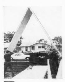
Carport, built by hinging foam-core fir plywood panels together prior to erection, cost some \$400 less than conventional semi-enclosed carport. It demonstrates cost-cutting advantages of components as well as new building forms they make possible.
