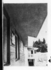
A nother smart idea from C. K. Dart: by using ¼-in. Masonite Pegboard to form his soffits, he gets two advantages: (1) the perforations provide excellent roof ventilation; and (2) the material's surface lends visual interest to large overhangs.
