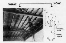
SPECIAL TECHNIQUE . . . Same tool, with special guard, fastens metal overhead door tracks to steel jambs.
