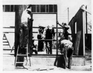
Exterior wall panels were erected in 3 hours, 20 minutes. Outer face is ½" "brushed grain" plywood with inset redwood battens; inner face is ¼" fir plywood. Foamed styrene core gives panel a total thickness of 2¾" and a "U" value of 0.1. The individual panels are tied together with splines and a continuous top plate shaped to conform to roof pitch.
