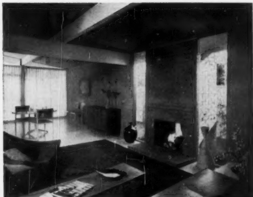
VARIETY: windows flank fireplace on both sides, break flat plane of living-room wall. Rugged post-and-beam construction counterpoints lightness of glass curtain wall.
