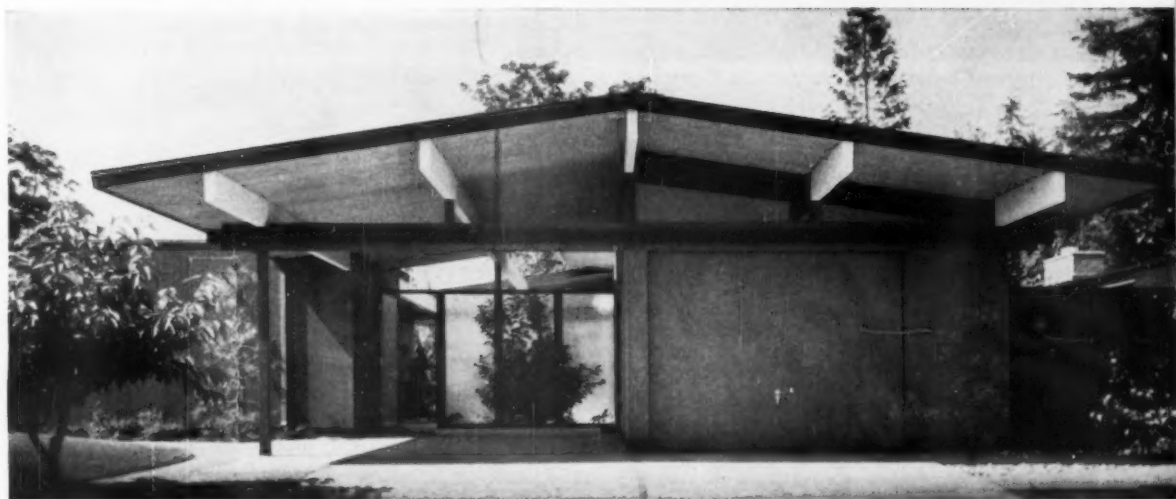
WIDE OVERHANGS, obscure glass panels, create a striking entrance effect. Garage doors echo the theme of restraint.
