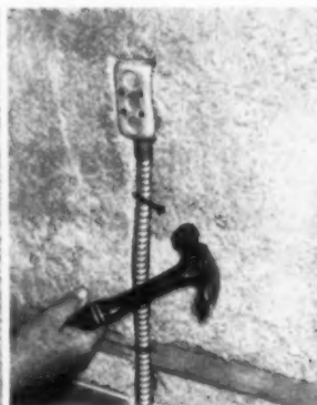
Wiring is easy from either side of wall. Cable is nailed into saw-cut groove.
