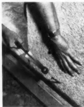
Toe-nailing is required only to position panels while super strong mastic sets.
