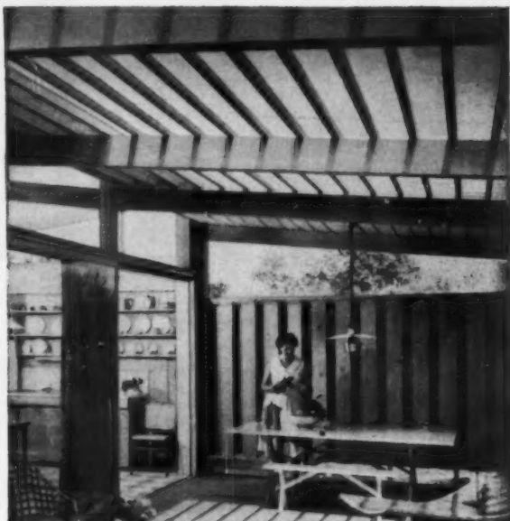
Living just naturally gravitates to the patio under this lanai of basic framing members. Handsome ventilated board fence assures privacy for this expanded outdoor "room," without eliminating breezes. Donald Nick is the architect.
