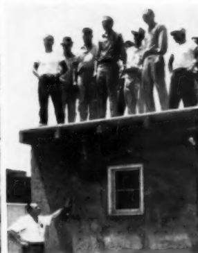
Cemex load-bearing walls eliminate studs, save from 11 to 14% over conventional construction.
