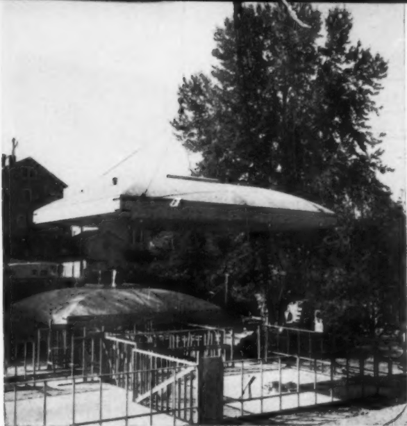
2 One dome-like component roofs an entire classroom. Properly built, such components save time and money, last indefinitely. But 25 years' watch-dogging the plywood industry by the DFPA has underscored the need for quality control in fabrication.
