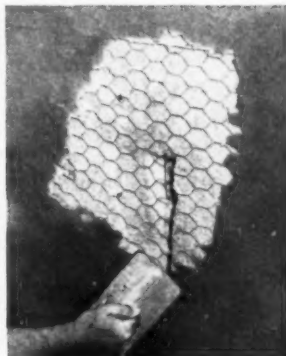
Plaster and stucco bonds perfectly. Only ground and finish coat needed.
