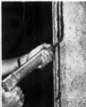
Double bead of Miracle mastic gives joint that is stronger than the Cemex itself.
