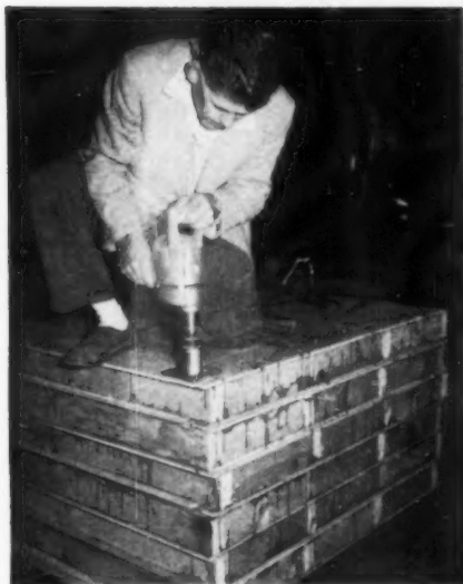
5 Roving quality engineers pull plugs from random panels at nonvital spots. If panel is sub-standard, fabricator's quality label can be withdrawn.
