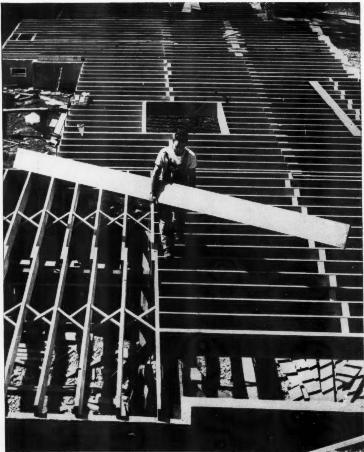
Like more and more homeowners, the family building this modern ranch home specified traditional joist construction with sub-flooring, to provide the comfort and beauty of hardwood floors. John Sutton, architect. Fister Construction, builder.
