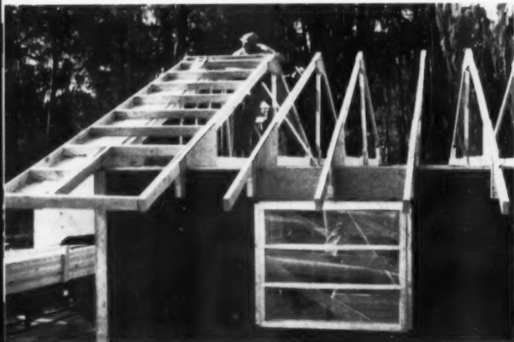
◀ LADDER COMPONENT makes the gable overhang. It's spiked to the last regular truss, extends over top of special gable truss (photo, next page).
