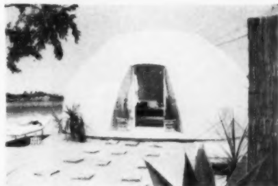
RADOMES —55-ft. plastic-skinned domes like this house radar equipment on the Distant Early Warning Lines. They withstand winds of over 200 mph.
