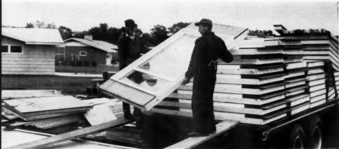
LURECO component system is based on a 4-ft wall panel. This is a window panel being unloaded.
