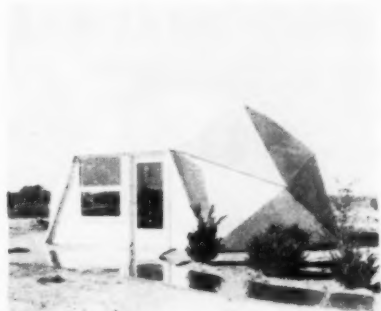
COTTAGES —This one, from Pease Woodwork Co., Hamilton, Ohio, is wood-framed, covered with plastic-faced plywood. Other uses: garage, farm shed.
