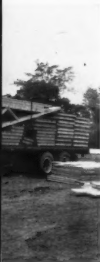
LURECO component system is based on a 4-ft wall panel. This is a window panel being unloaded.
