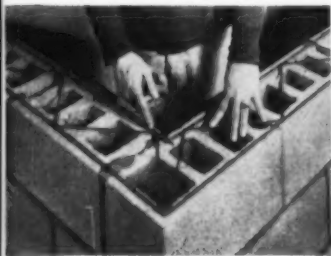
Two engineered products that meet a need. Dur-o-wal reinforcement, shown at left, and Rapid Control Joints, right. Weatherproof neoprene flanges on the latter flex with the joint, simplify the caulking problem.
