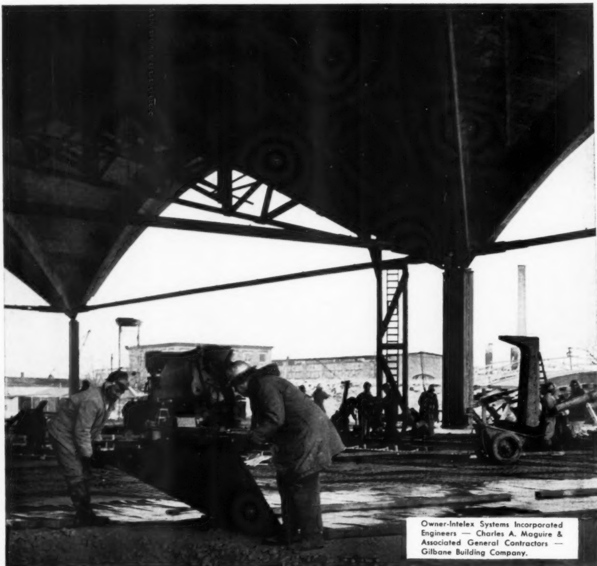
Dry floors assured at construction of new post office at Providence, R. I. Over 200,000 sq. ft. of Moistop used.
