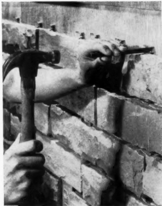
3. RANDOM LENGTHS of stone—from 8" to 24"—give interior or exterior stone-veneer walls a natural look. Mortar between joints finishes job.
