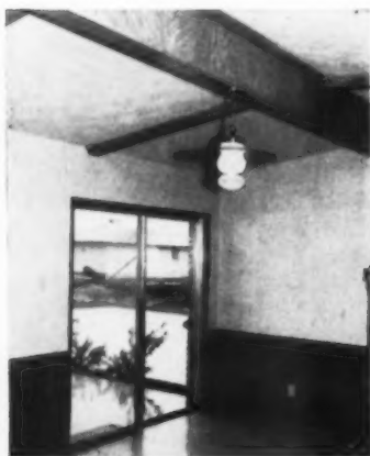
12. Form exposed-beam ceilings with 2x4s
