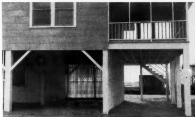
8" CYPRESS STILT foundation protects the house from occasional threat of storms and high water, leaves room under the house for extra storage, bathers' dressing room and shower, plus two car ports.
