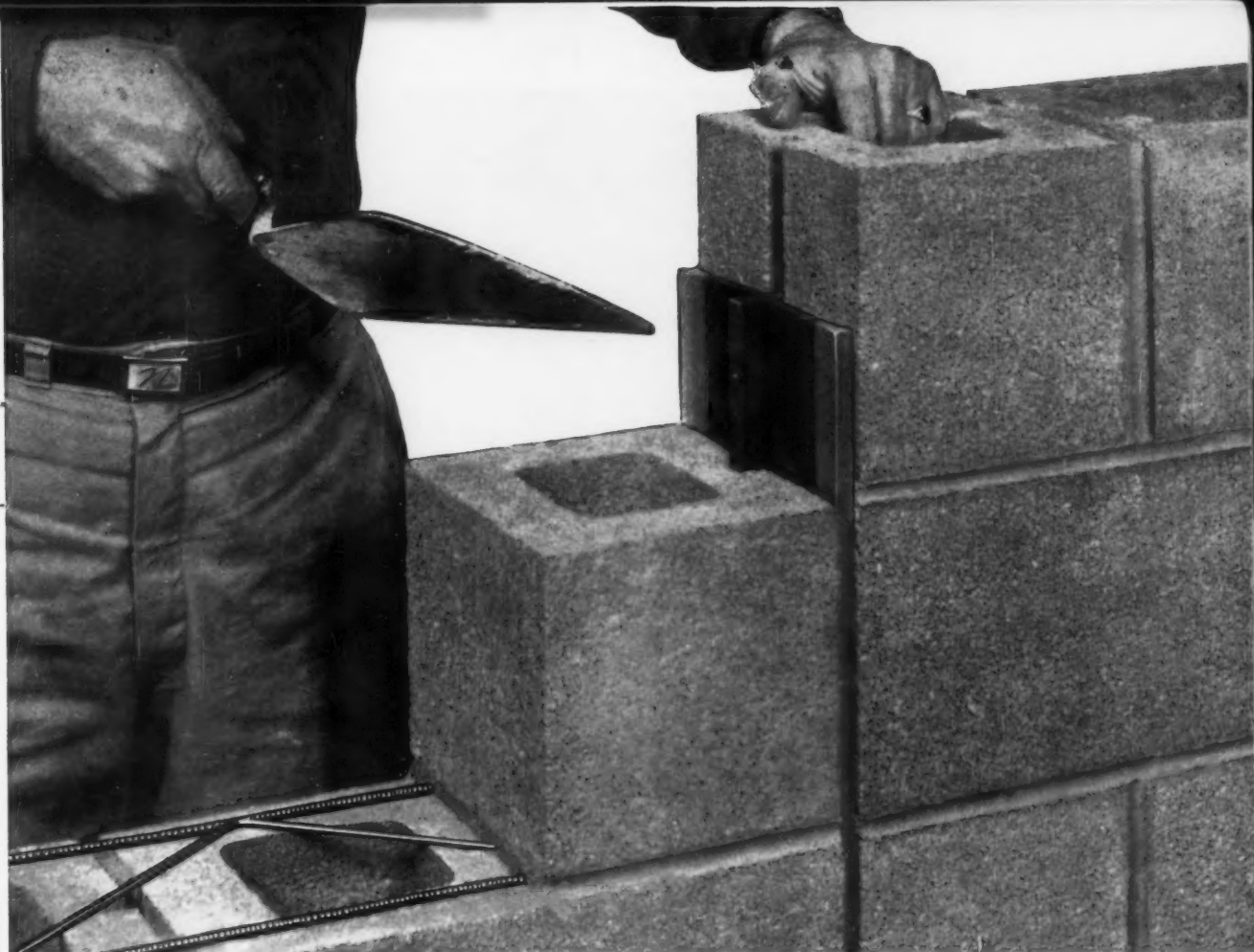
Trowel points to Wide Flange Rapid Control Joint, a companion product used with Dur-o-wal
