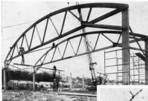
Forbes Lumber & Supply Co., Cheswick, Pa. Contractor: J. O. Thomas & Co., Wexford, Pa. 9 Rilco Bowstring Trusses span 80', spaced 20' o.c.
