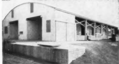
Forbes Lumber & Supply Co., Cheswick, Pa. Contractor: J. O. Thomas & Co., Wexford, Pa. 9 Rilco Bowstring Trusses span 80', spaced 20' o.c.
