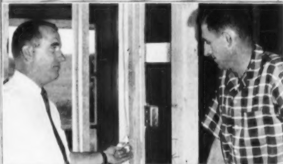
Builder Paul Starck and telephone company man Jack Adams discuss an outlet location for a wall phone in a home that’s partially completed.
