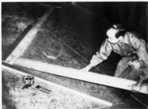
1 SIMPLE JIG made from 2x4s and a plywood sheet is used in assembling the half frames. Jig is needed to make sure all frames are identical in shape.
