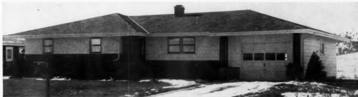
Builder is using B&G Hydro-Flo Heating in one hundred homes like this.
