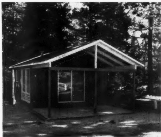
MOST POPULAR of Tingstrom's four models is the Bijou (L). Its completed price of $4,800 includes plumbing, wiring, painting, furnace, and interior paneling. Many buyers take two units, rent out one for extra income.
