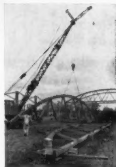
Forbes Lumber & Supply Co., Cheswick, Pa. Contractor: J. O. Thomas & Co., Wexford, Pa. 9 Rilco Bowstring Trusses span 80', spaced 20' o.c.
