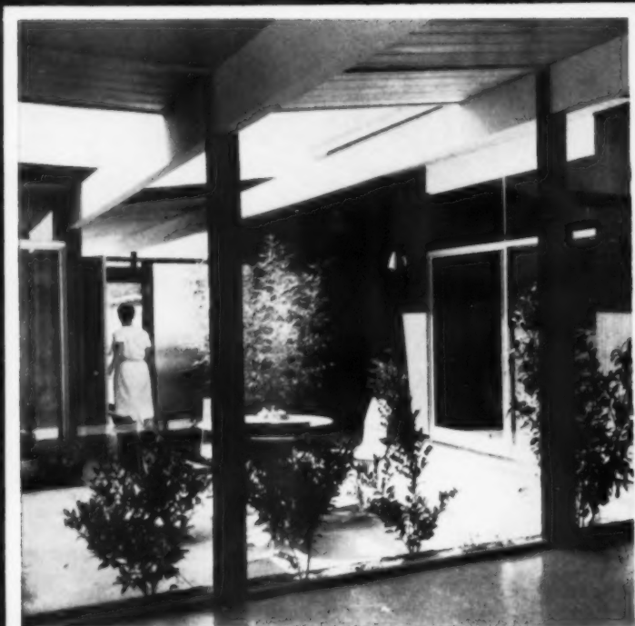
OPEN, UNCLUTTERED view of the outdoors is one of the most important design features of post-and-beam framing. The photo shows how metal fasteners eliminate unsightly scabbing, keep the design clean and simple.
