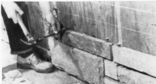
2. MODULAR UNITS of stone are 1/2" thick, 4" or 8" high. Steel anchors fit into stone grooves, are then pinned to wall. Anchors support a minimum of 30 lbs.
