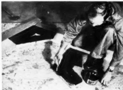
2 STUD, RAFTER, GUSSET plate are coated with glue—casein, or resorcinol-resin—before nailing the plywood gusset in place to make the joint rigid.
