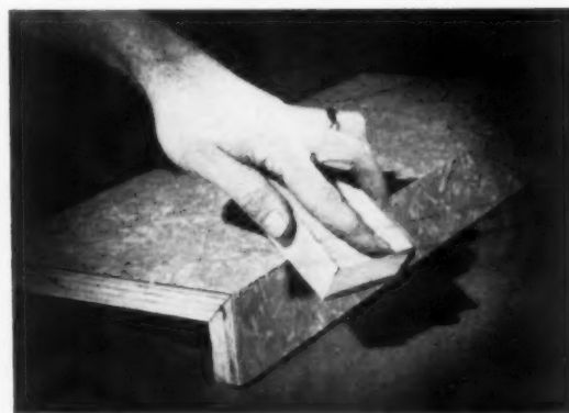
STEP FOUR —Sharp edge may call for light sanding to make mitered joint of countertop safe for handling.
