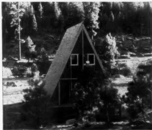
At right is A-frame model built by Rex Reid who operates the Builders Service Center, Donner Lake, Calif. The cabin is an equilateral triangle with 24 ft. to each leg. Reid has commitments to build 52 cabins this Spring.
