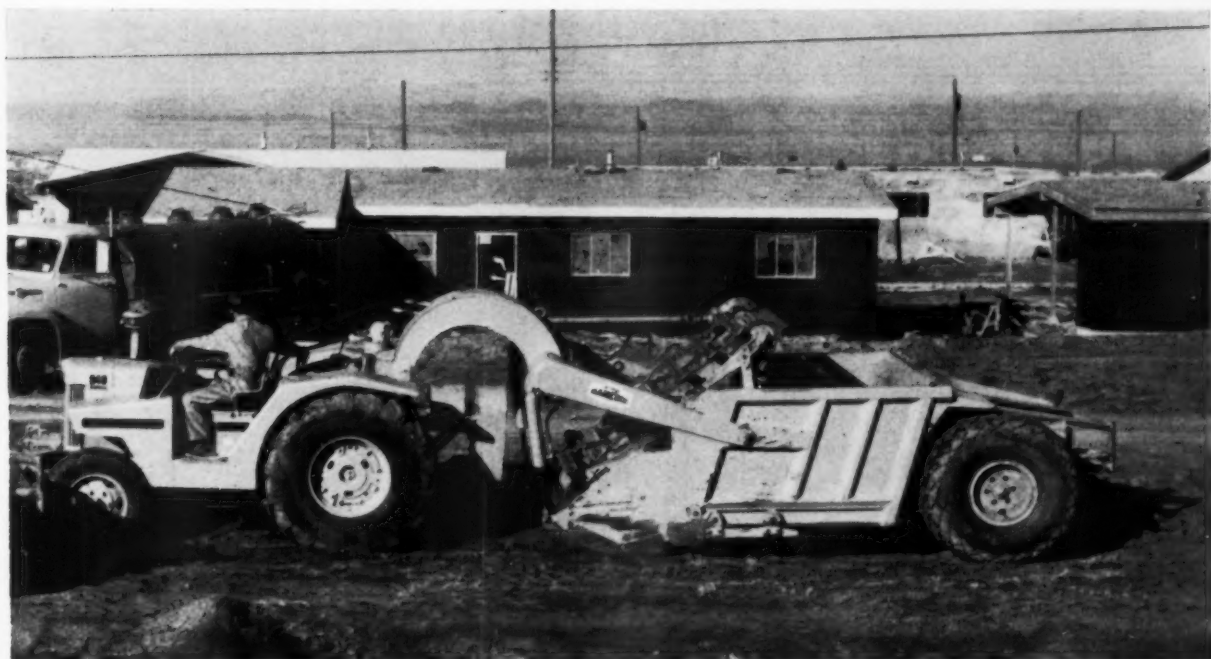
Bellamah subdivision near Albuquerque, N.M. Self-loading, self-propelled rigs started Bellamah moving his own earth.
