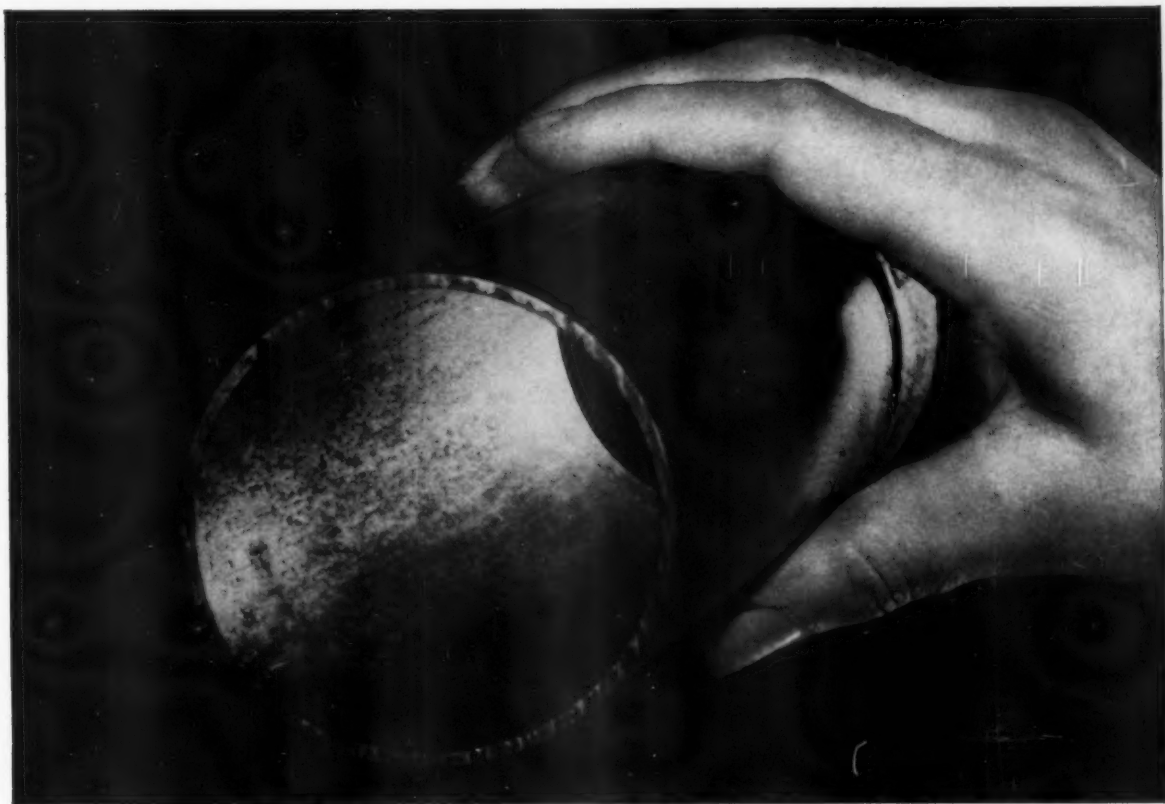
Unretouched photo of 3" dia. copper tube removed after 13 years' service in a soil line.
