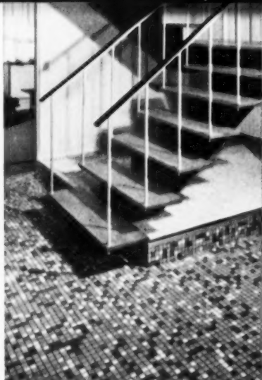
Ceramaflex installation at NAHB RESEARCH HOUSE, East Lansing, Mich.
