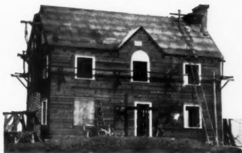
1924: Thousands of Maze rustproof nails, hot-dipped in molten zinc and trademarked "ZINCLADS," were used to build this house.
