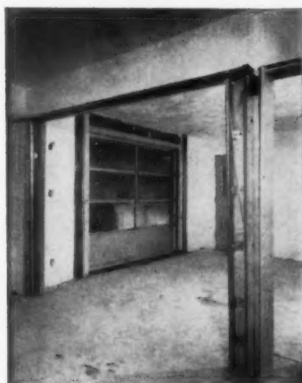
FAMILY ROOM AND KITCHEN become one when Overhead door is lifted. It's mounted to be concealed in the ceiling when raised.
