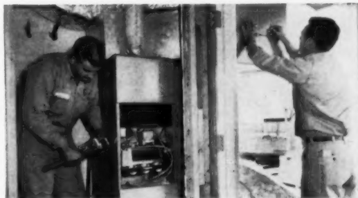
SELF-CONTAINED —Carrier's cooling unit projects through prefabricated sleeve in wall to join furnace plenum. Assembly controls air flow between furnace and cooler.
