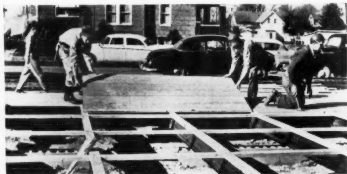
PLACING DECKING —Grids 4 ft. square support 2-4-1 plywood panels that provide a rigid flooring. Floor finish in the form of vinyl, plastic tile, hardwood, wall-to-wall carpeting, etc., can go directly over plywood panels.
