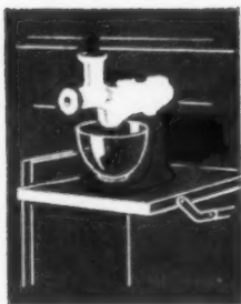
Pull-out mixer unit drops into place below work counter.
