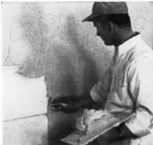
Rutenberg workmen prepared walls for plastering in two-thirds the time required by ordinary methods. Styrofoam bonds directly to wall with portland cement . . . plaster is applied directly to Styrofoam.
