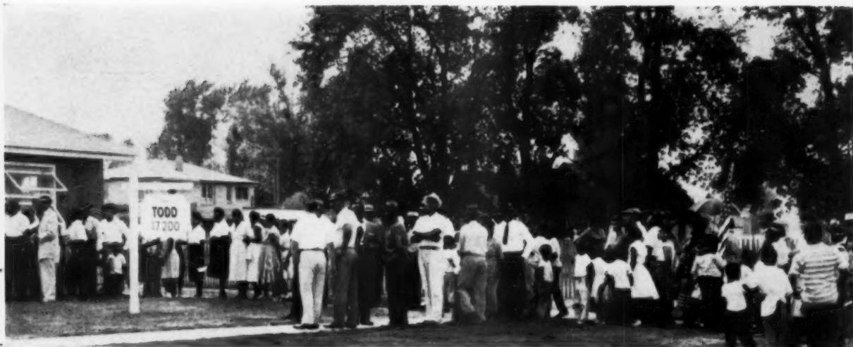
OPENING DAY at Lincolnway's subdivision. Prices for the prefab models range from $14,500 to $17,750, including lot.
