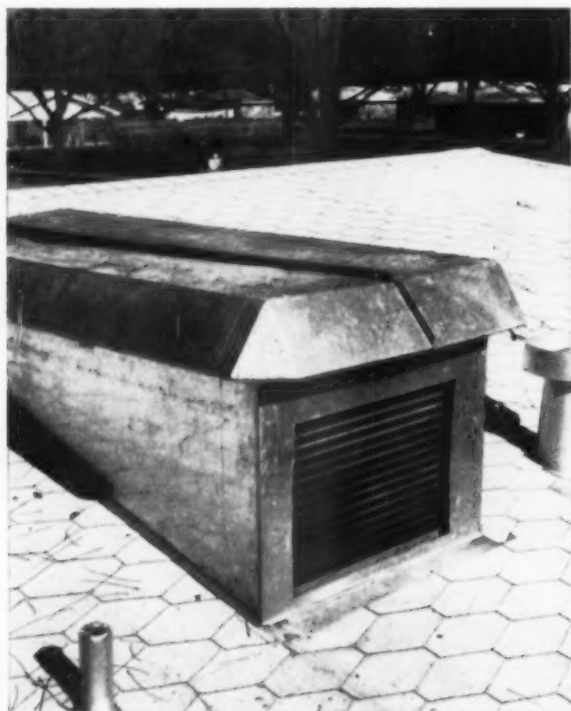
METAL GABLE in position (left). Above, it's easily removed by one man, to permit servicing of air conditioning unit.
