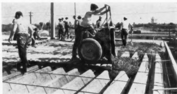
NEW ROOF COMPONENT adds distinctive air to Ontario church (left). Above, component serves as roof concrete form.
