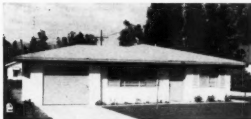
ONE MODEL—Harmony Homes are simply designed, well built. This model sells for $4,845 (without land) plus garage for $395. Exterior walls are stucco; roof is rock.
