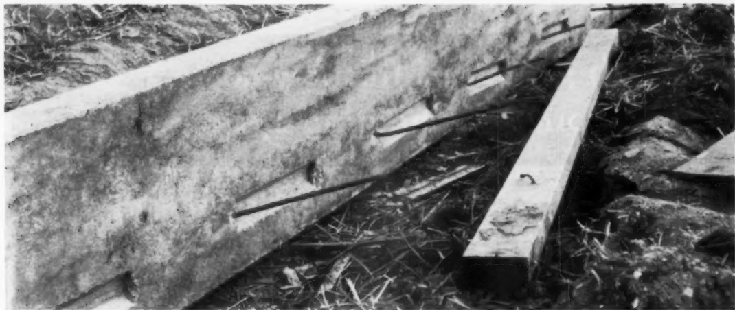
KEYWAYS are cast into beams wherever patio or garage slabs will abut. Bars are pulled out as shown, poured into the slab for a strong joint.
