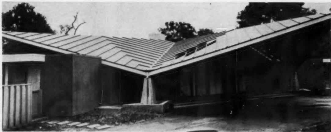
BATTEN SEAM ROOF enhances the modern lines of this contemporary house built in Sunnyvale, Calif.
