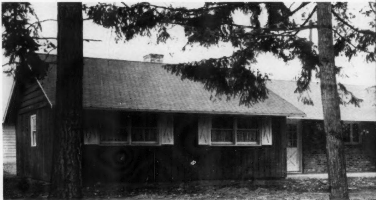
PRICE TAG: $15,000 including an $1,850 lot for this 3-bedroom, 2-bath house built with fabricator's help. Prefab
