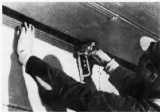
GUN TACKER staples Cornerite to wall and ceiling. You hold material with one hand, staple it with other.
