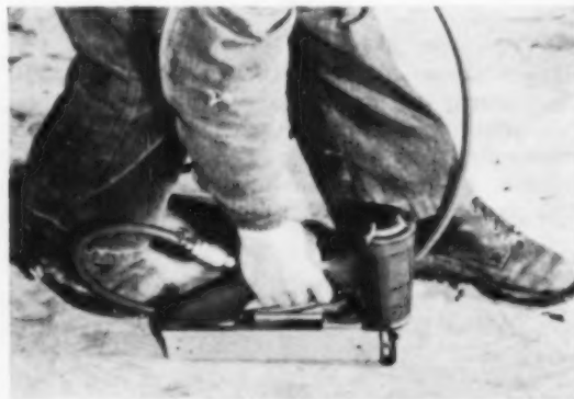
STAPLE NAILER for stapling down plywood subflooring works as fast as man can position tool, pull trigger.
