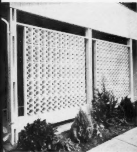
CARPOR-T-SCREENING makes use of 8" lengths of Transite pipe (4 5/8" dia.) in a framework of 2x4's. It's simple to build, lends texture and pattern.
