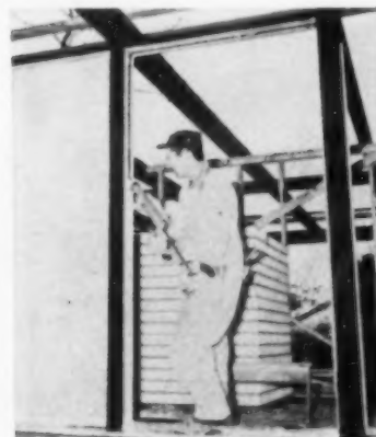
INSIDE STOPS were preset to posts. Liquid butane caulking was applied, then panels were pressed into place.
