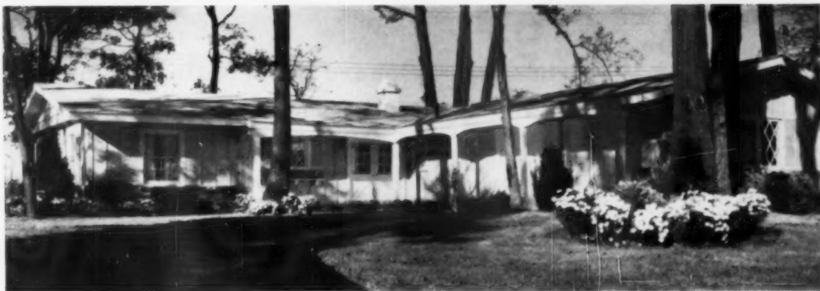
James Crabb Associates, Wilmette, Illinois, checked costs of two homes like this, found copper tube plumbing made appreciable savings over other metals.
