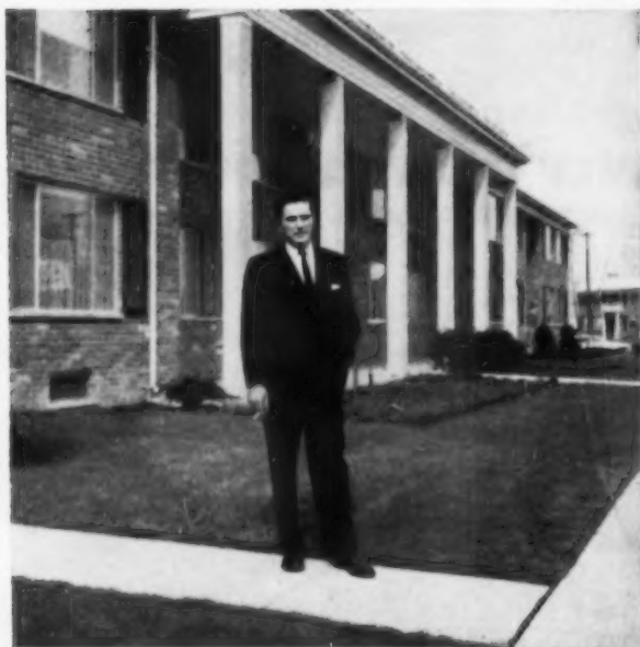
River Oaks garden apartments and Craig Smith of Sullivan-Smith, Inc. builders. All apartments in this development have at least one Built-In Air Conditioner; some have two.
