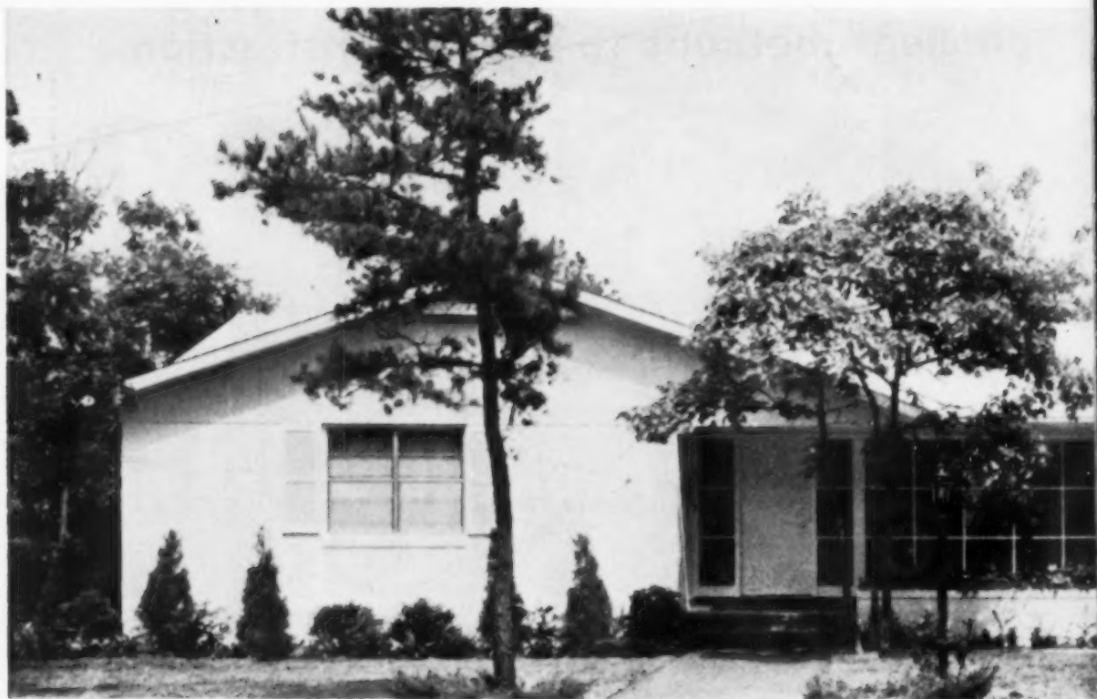
COLONIAL TOUCHES give an air of simple elegance. This elevation is for the North—one of three designed by architect
