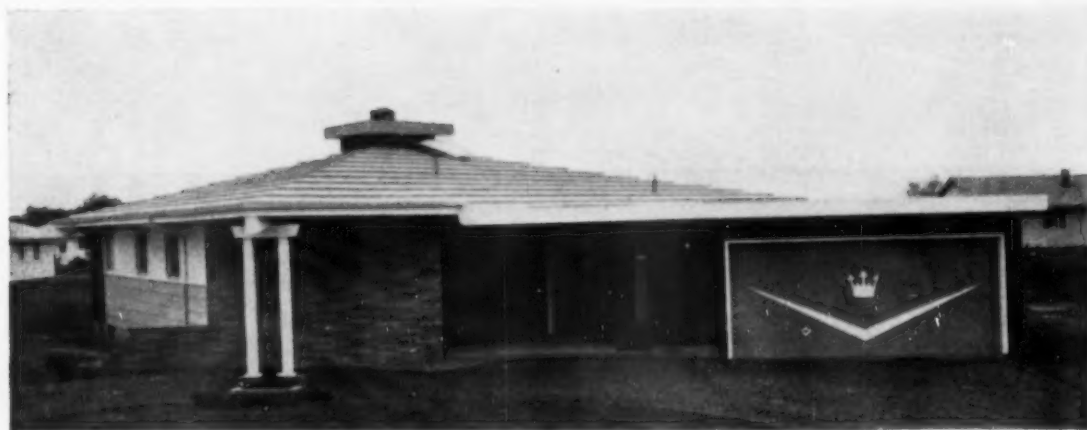
EXTERIOR IS WELL SCALED, gives a low-slung impression. Stylish Bermuda seam terne roof gives a contemporary effect that blends well with the traditional look of the columns and split concrete-block walls.
